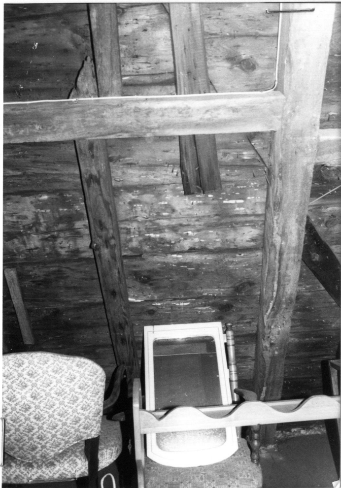
FRONT SLOPE OF ATTIC ROOF (1985)
