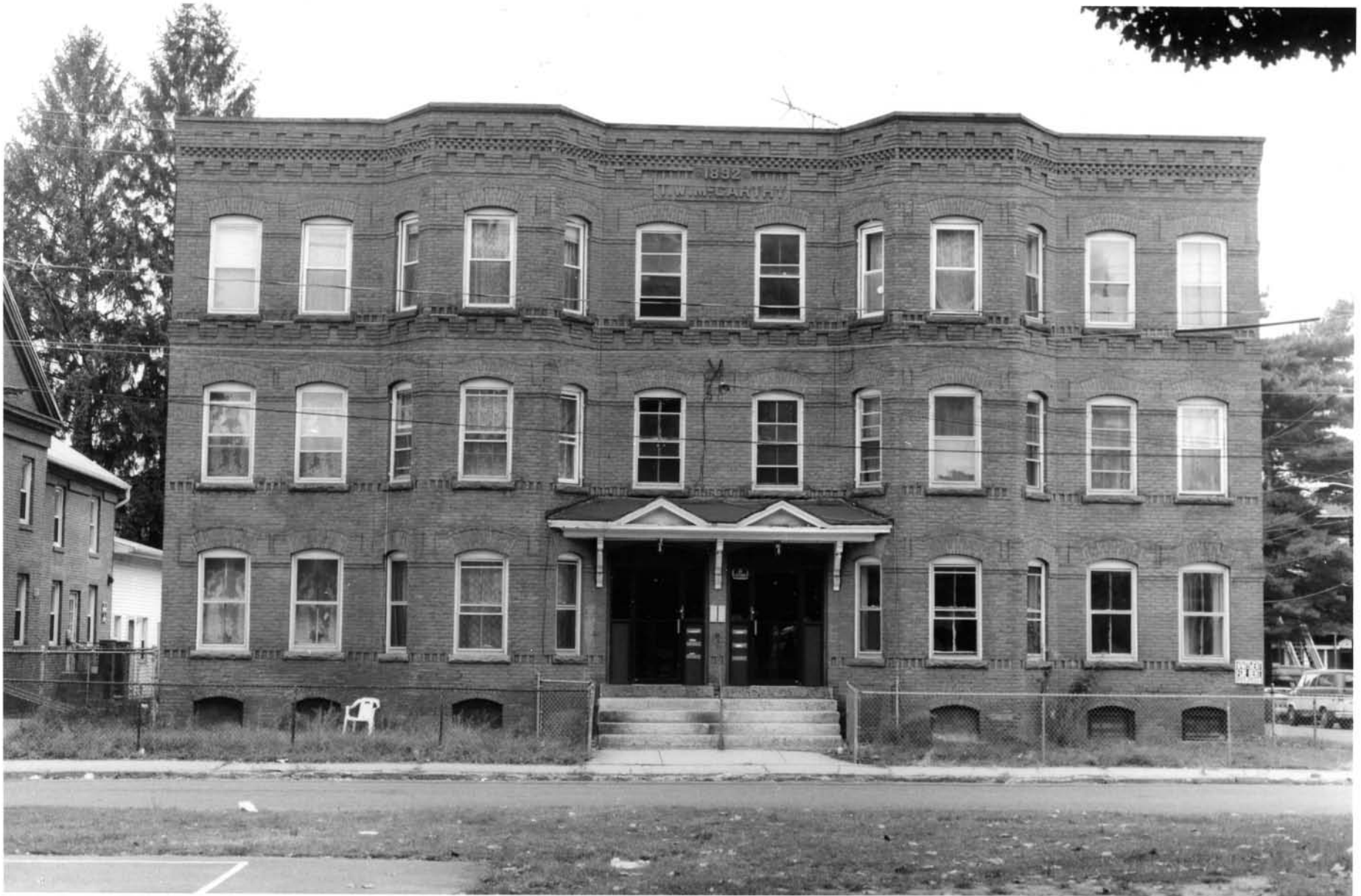
11. 37-39 School Street, facing NW (Photographer: Michele Plourde-Barker, October-November 1996)
