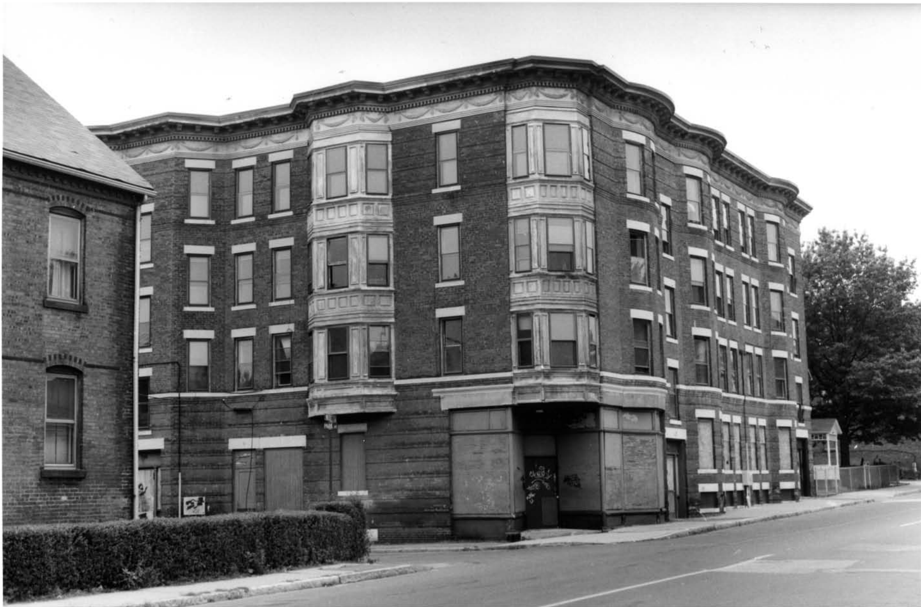
12. 63-71 West Street, facing SE (Photographer: Michele Plourde-Barker, October-November 1996)
