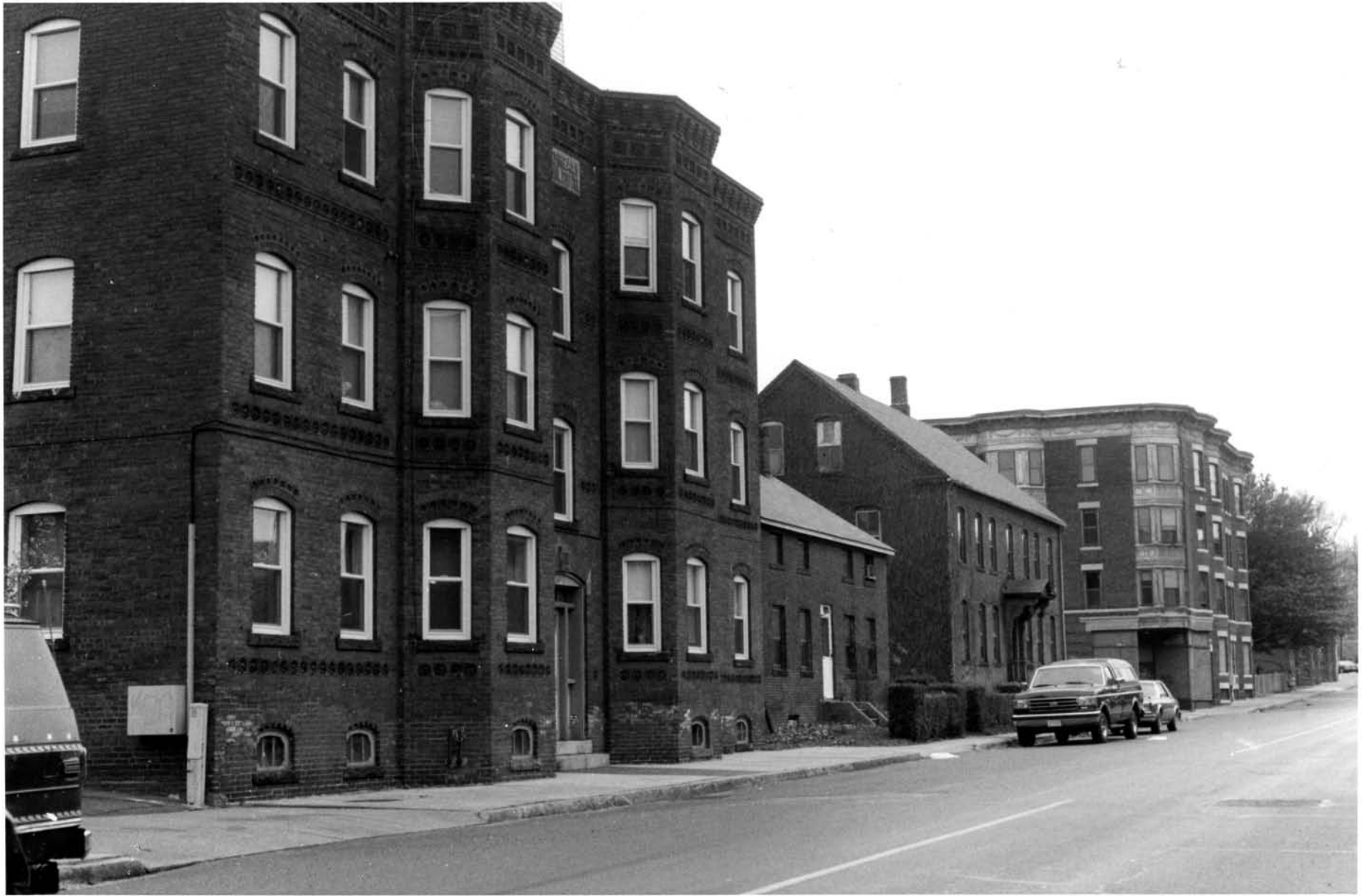
5. West Street, showing 53, 55, 59, 63-71 West Street, facing SE (Photographer: Michele Plourde-Barker, October-November 1996)
