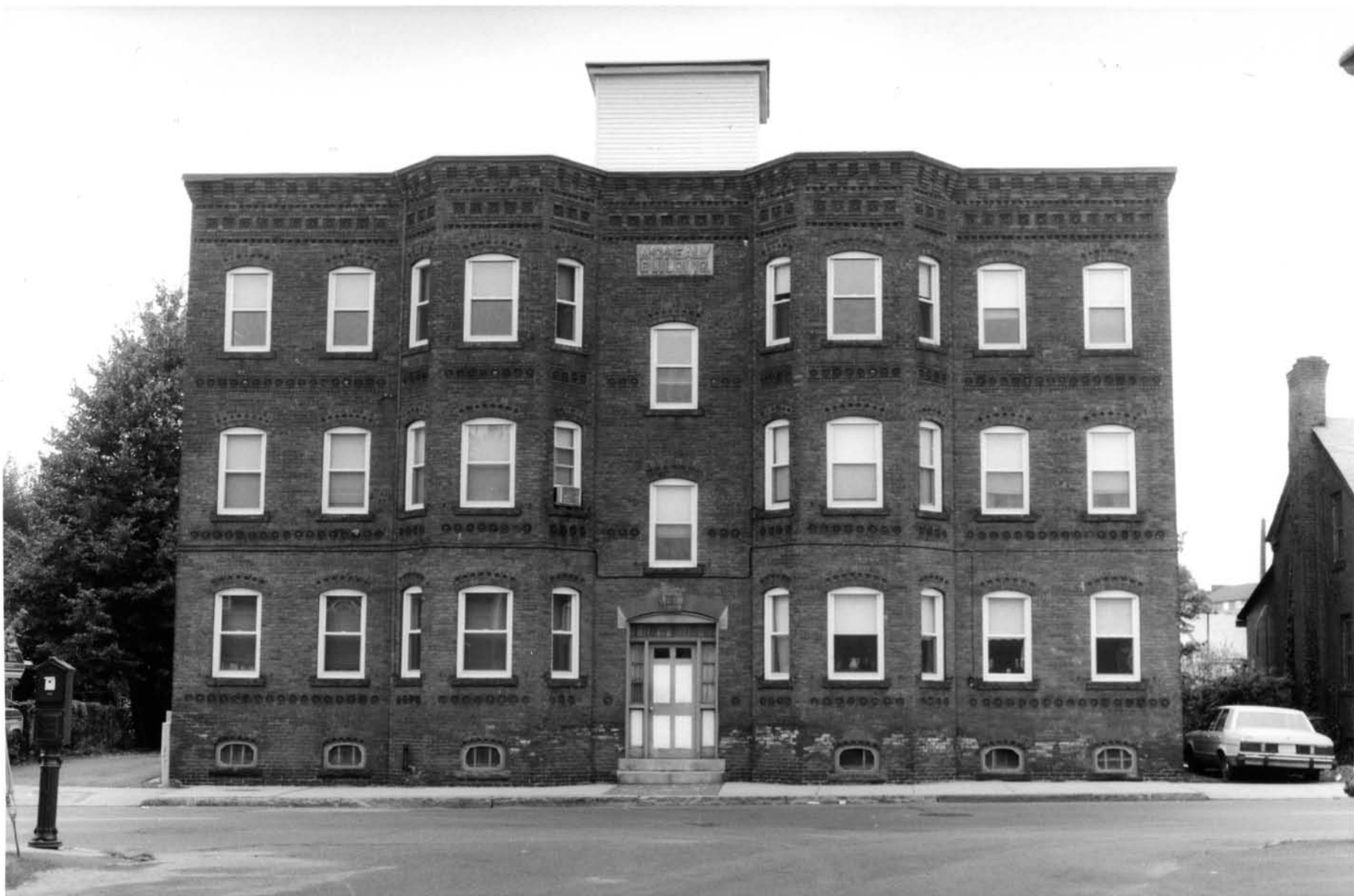
10. 53 West Street, facing SE (Photographer: Michele Plourde-Barker, October-November 1996)
