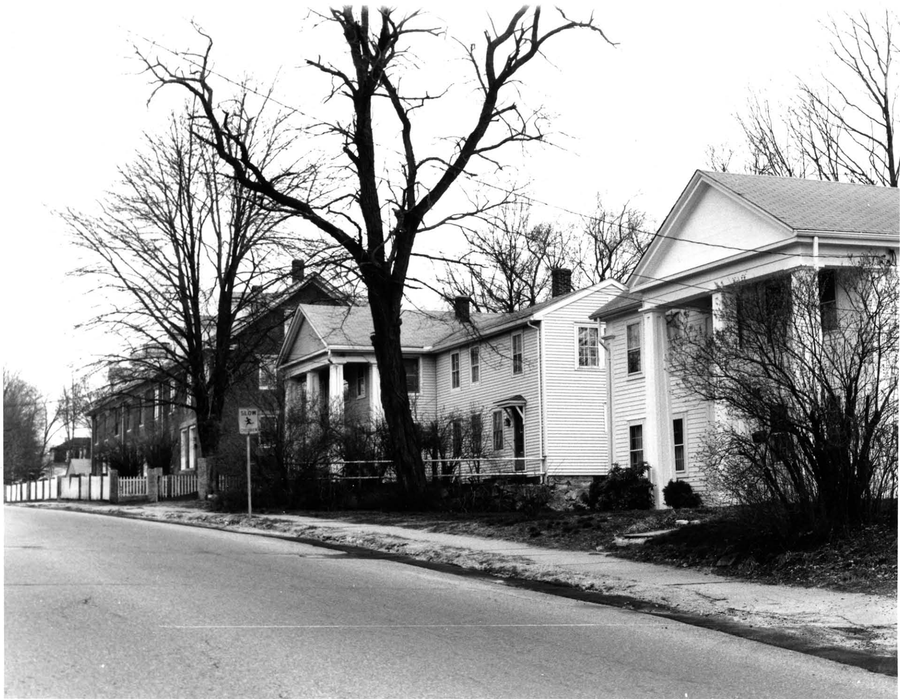
8. 20, 22, 24-34 Mendon Street, Parsonage, Headmaster's House, Overseers Block, looking north, northeast. (Photograph: Gretchen Schuler, April 1994)
