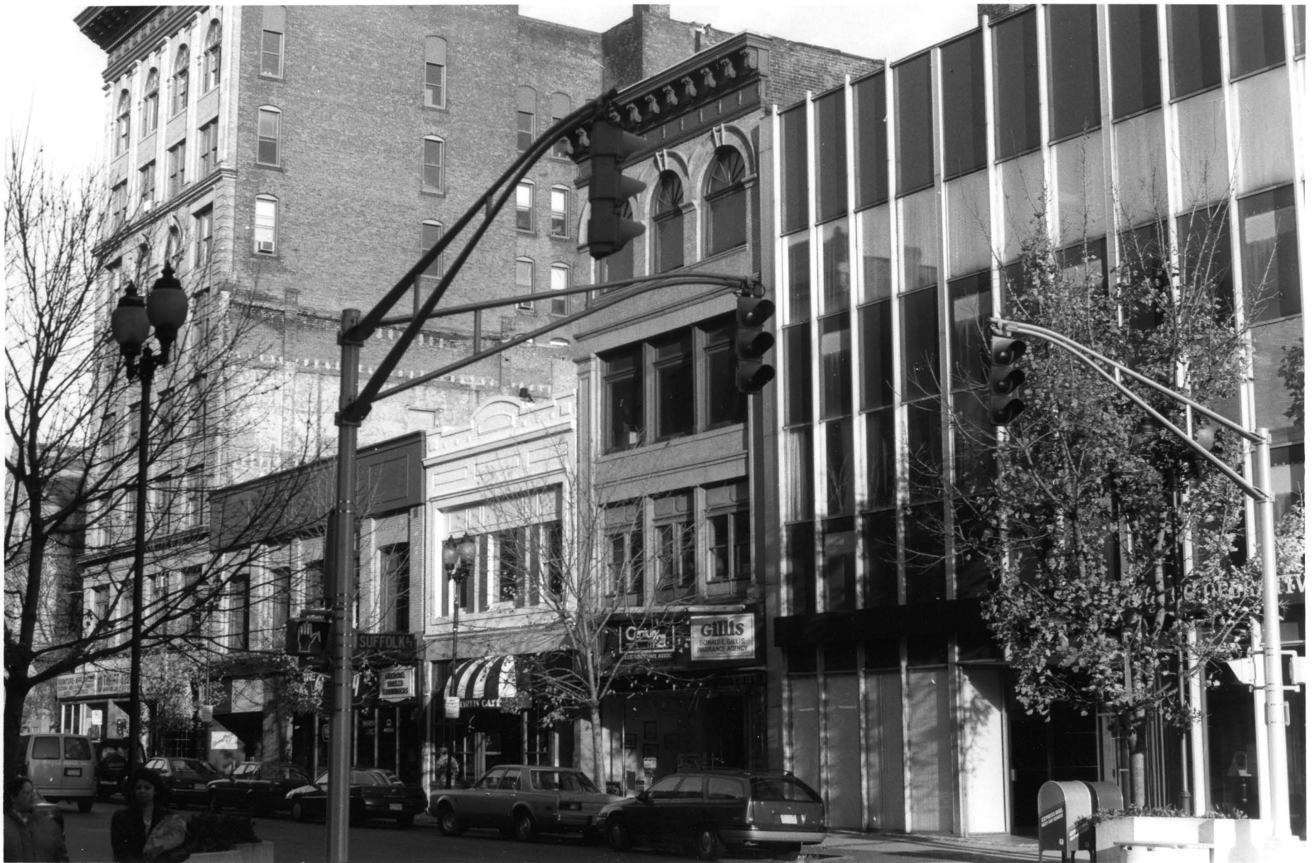
6. View northeast. L to R: 270-276, 278-282, 284, 288-290, 300 High Street. (Photograph: Gregory Farmer, June 1991)
