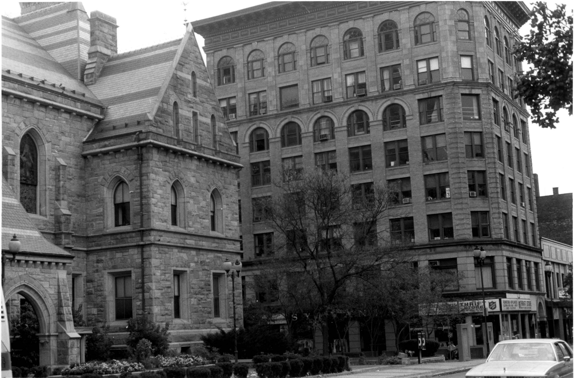
3. View southeast. L to R: City Hall (partial), 270-276 High Street. (Photograph: Gregory Farmer, June 1991)
