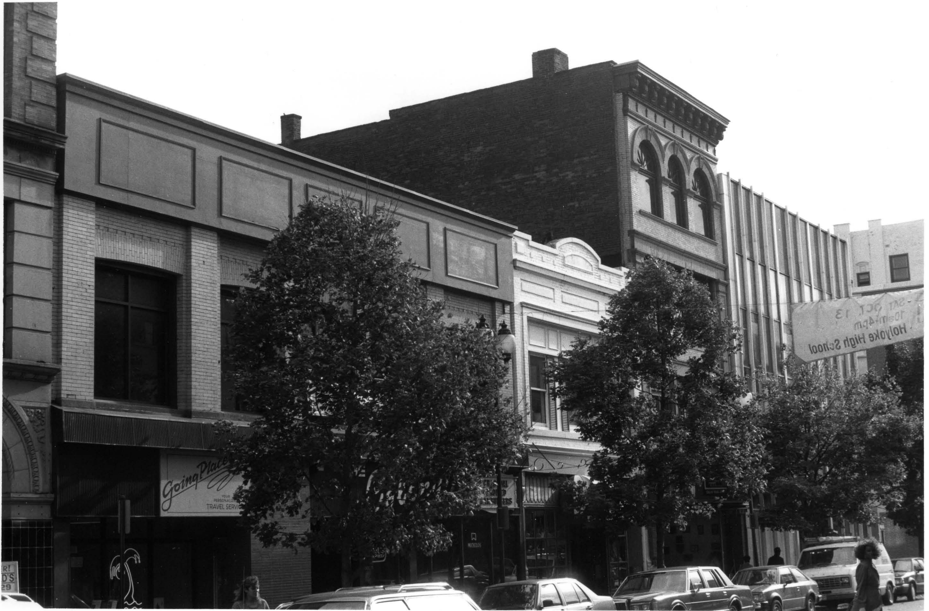
4. View southeast. L-R: 278-282, 284, 288-290, 300 High Street. (Photograph: Gregory Farmer, June 1991)
