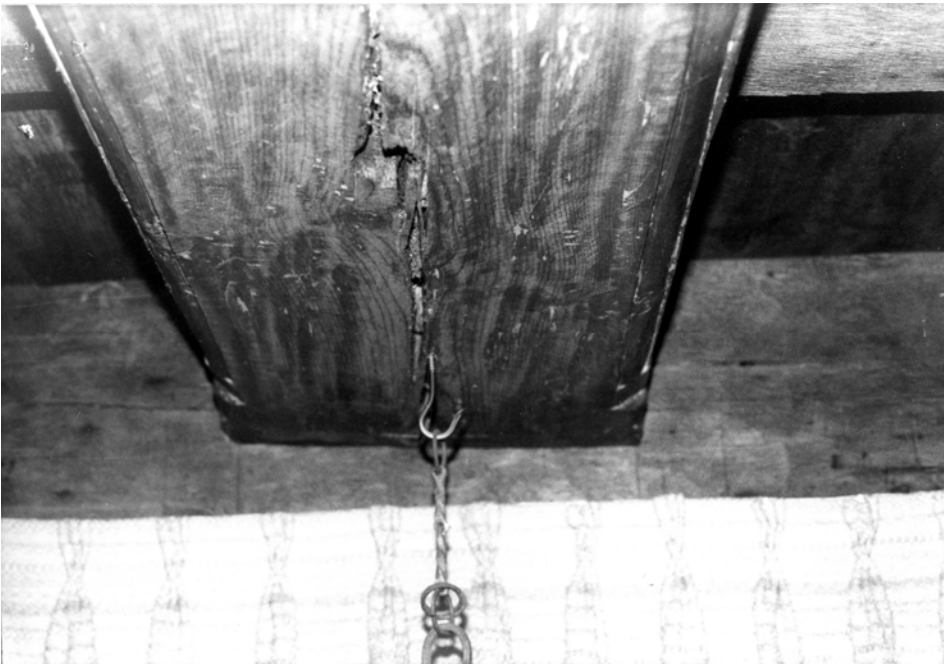
57:18 Summer beam, in east first-floor room
