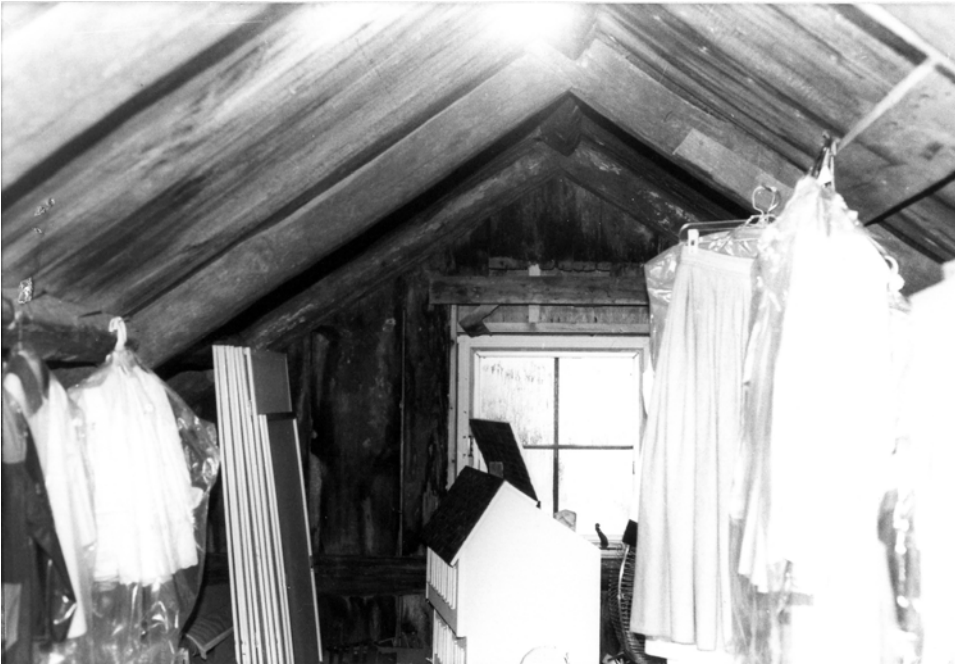
57:27 East end wall in attic showing exposed planking
