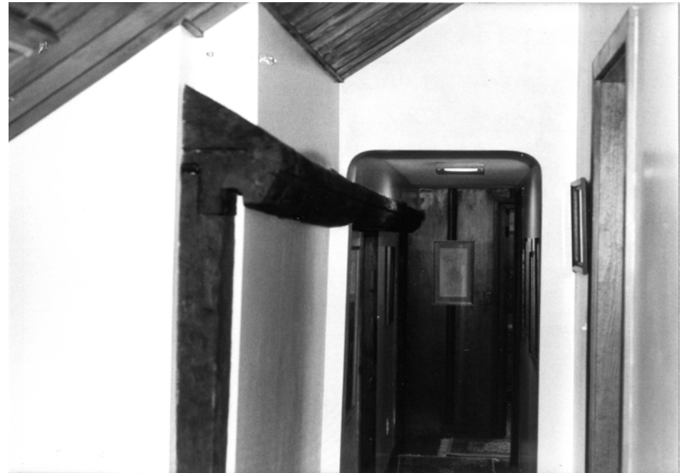
57:24 Cornice molding still in situ on plate cut to receive planks
