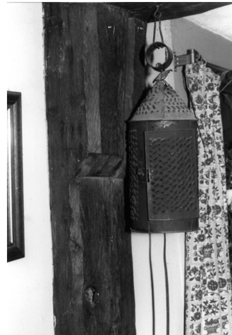
transverse summer beam and post of front wall, right-hand room
