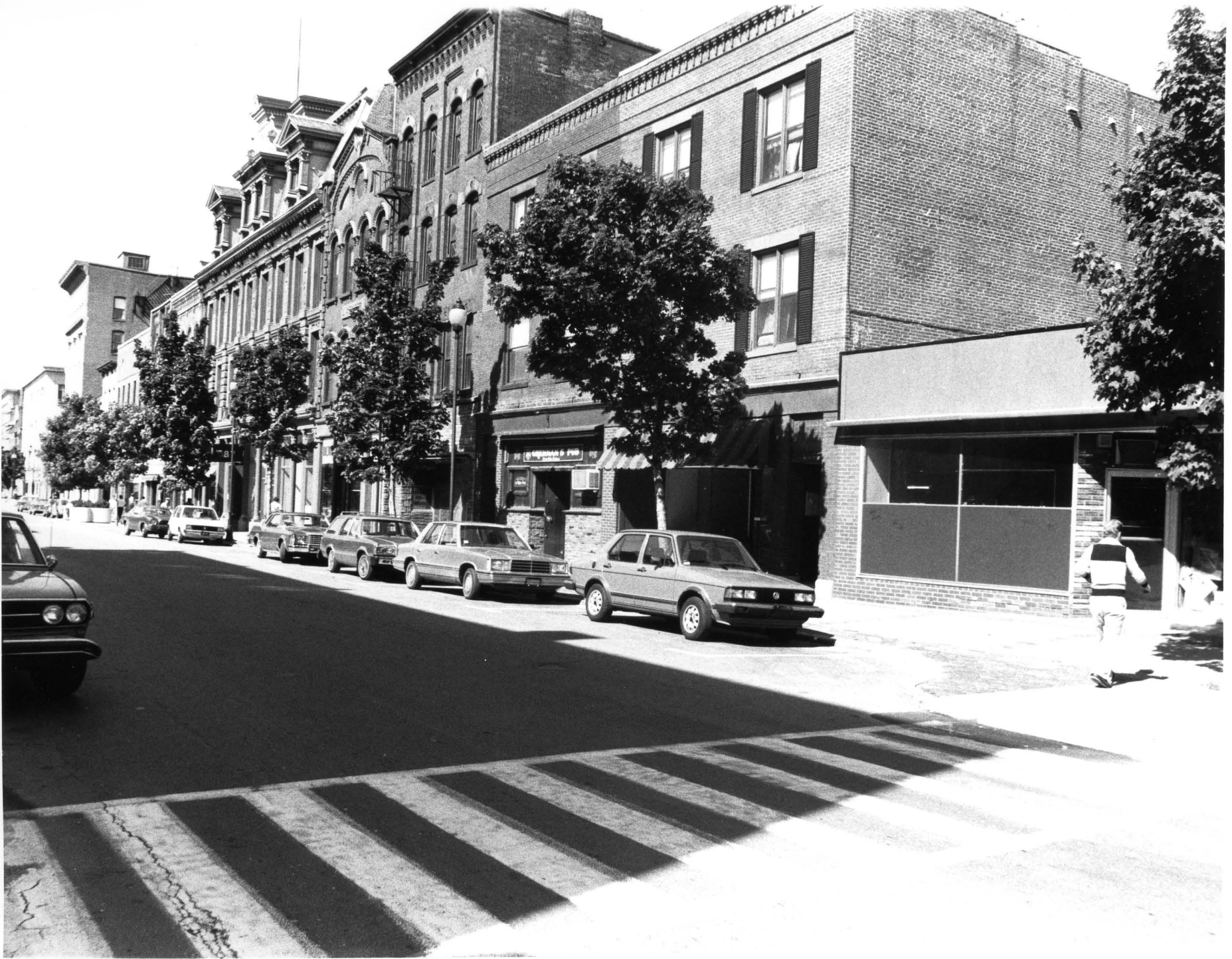
4. West side of High Street, view south from 169/171 High Street. (Photograph: Nora Pat Small, May 1985)
