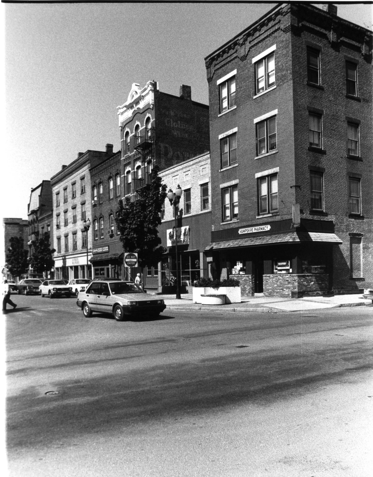
1. West side of High Street, view south from Lyman Street. (Photograph: Nora Pat Small, May 1985)
