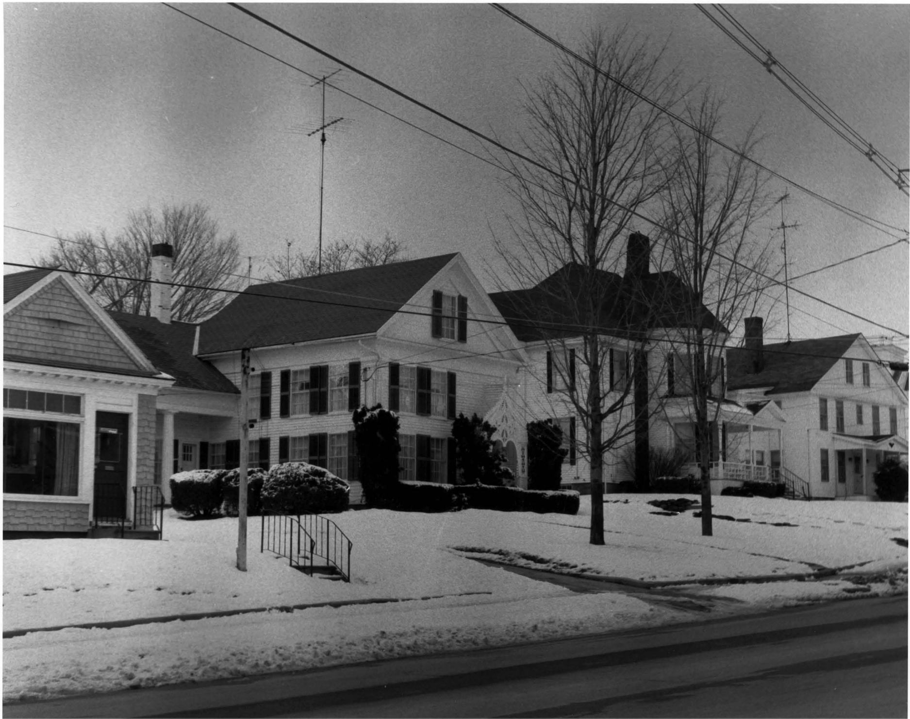
10. [Looking northwest along the west side of Elm Street at, L-R, 20, 22, 26 and 28 Elm Street.] (Photograph: Robert Chandler, winter 1983-84)
