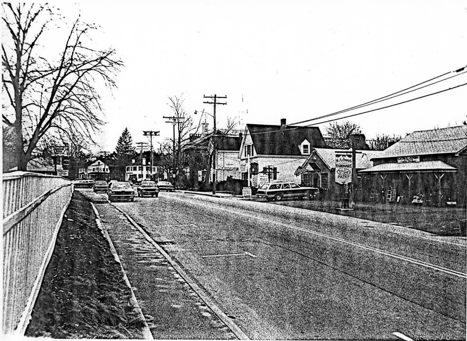
[Photo 2. Main Street looking west: R-L: 695, 687, 683, 673 (Memorial Town Hall), 667, and 661 Main Street. Photocopy, ca. 1981, from an original print supplied for the nomination.]
