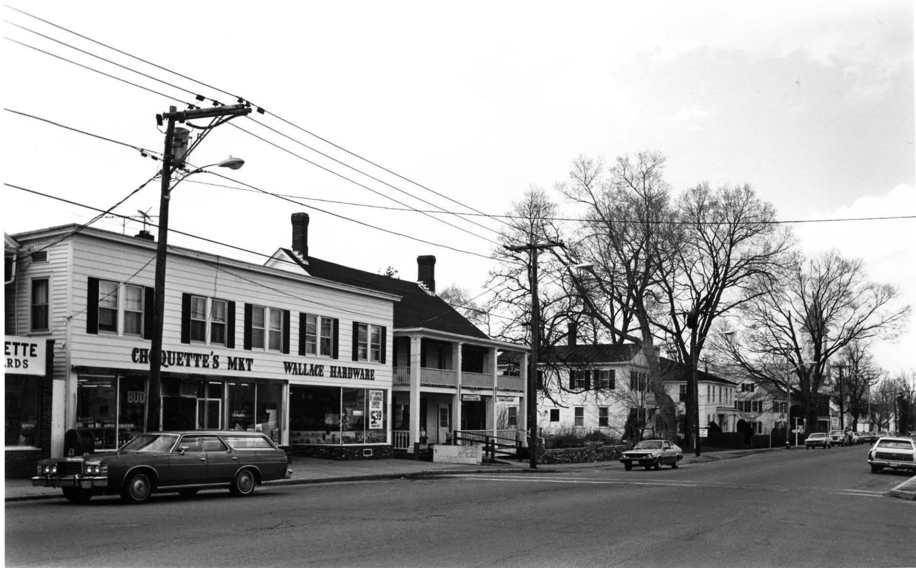
5. L-R (Looking northwest): Cocquettes Mkt (#2), 7 Main; Woodbridge & Clark (#3), 11 Main; Philo Dickinson (#4), 15 Main; Parsons (#5), 17 Main; Wright Bridgman (#6), 23 Main; Bridgman Brick Block (#7), 29 Main; Methodist Church (#8), 31 Main (Photograph: Charles Lennon, 1979)
