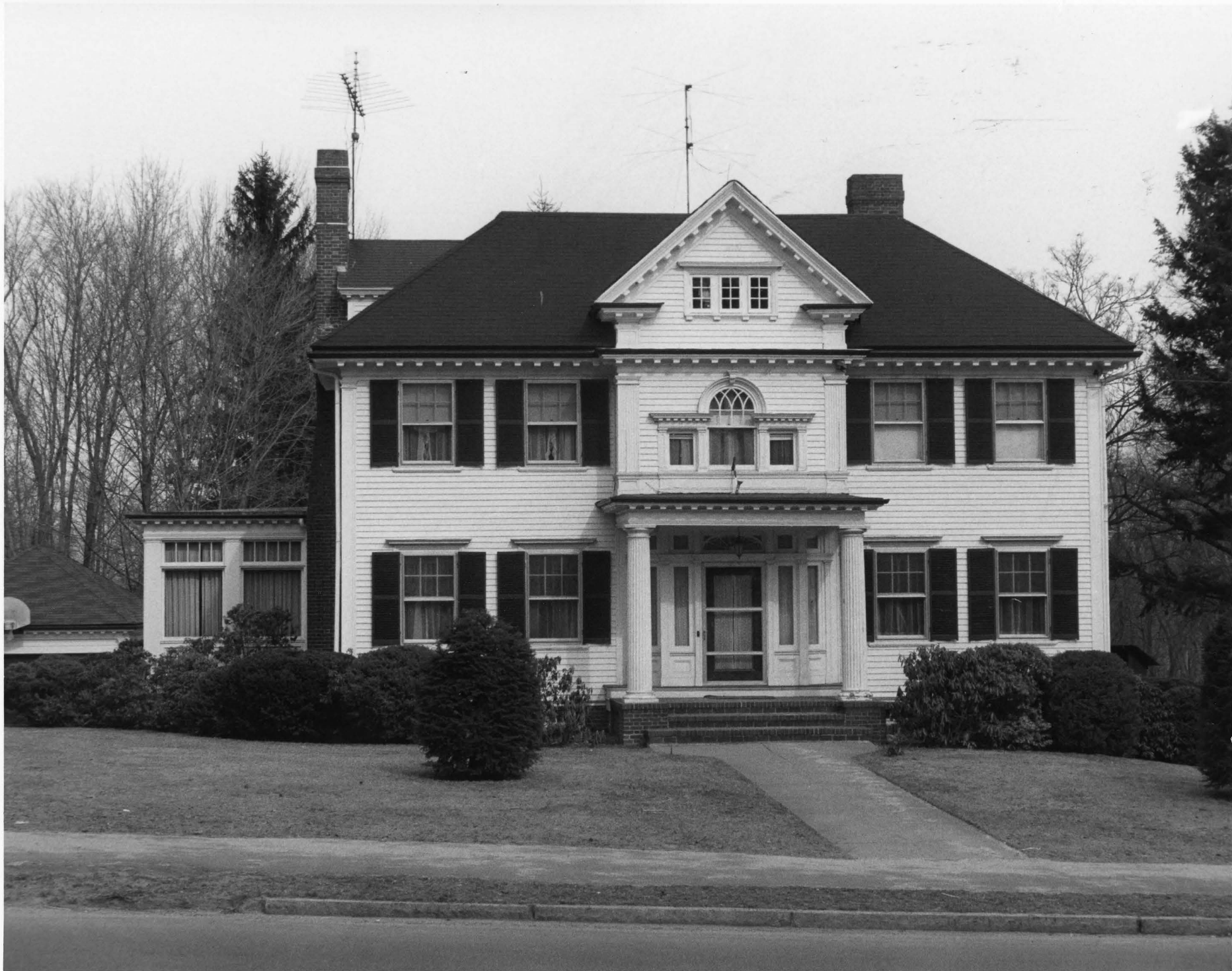
11. Looking from the front of the Bradford College Campus across South Main Street at the facade of the Evans House. (Photo: Ann F. Armstrong, Haverhill Public Library, 1976)
