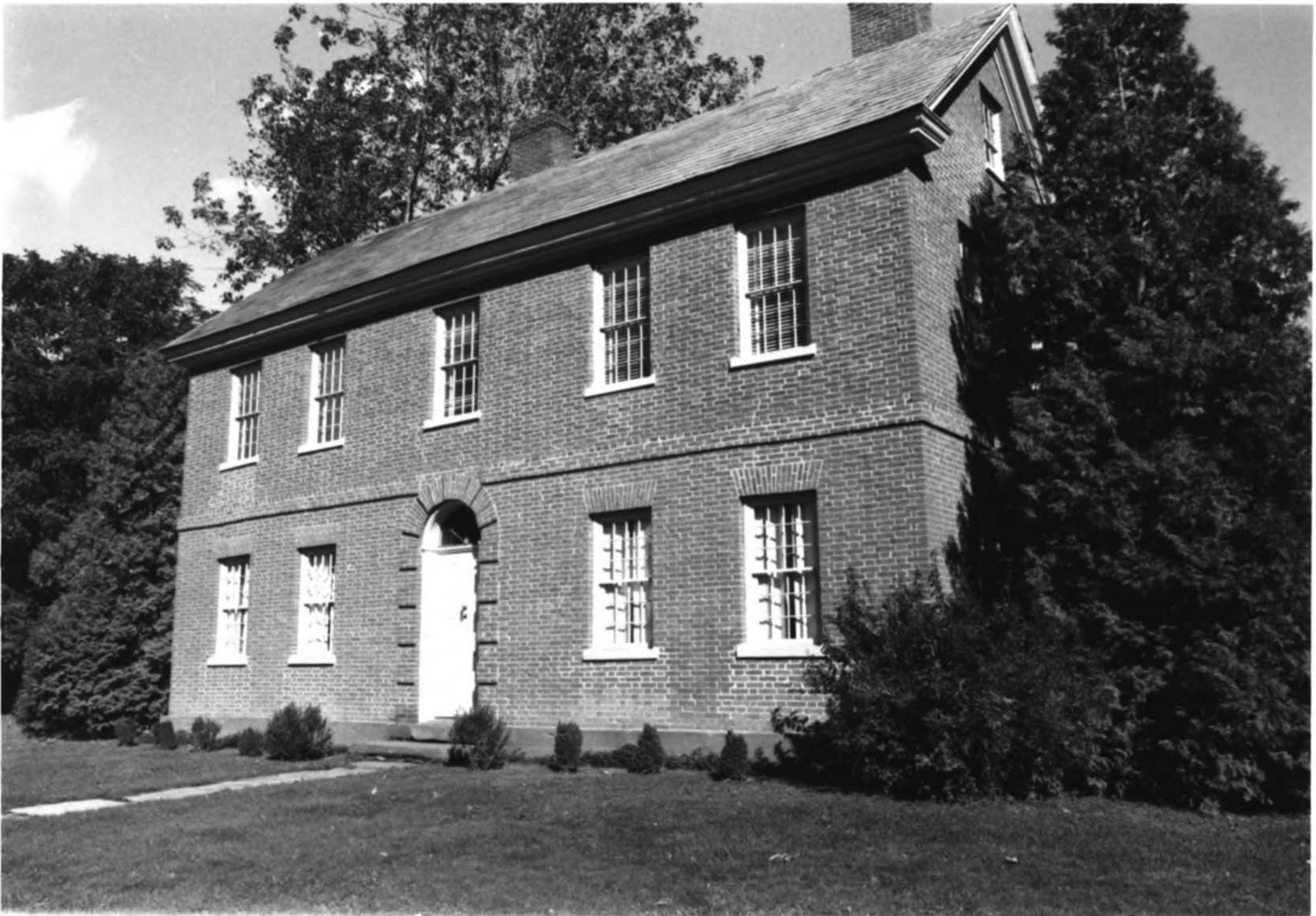
6. Asa Stebbins House, west (front) elevation. (Photographer: Polly M. Rettig, NPS Landmark Review Project, Sept. 1974) Photo from NPS Focus, http://nrhp.focus.nps.gov/
