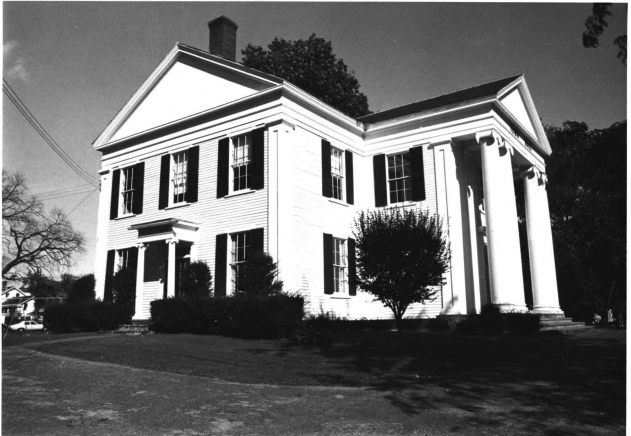
5. West and south (side and front) elevation of Town Hall. (Photographer: Polly M. Rettig, NPS Landmark Review Project, Sept. 1974) Photo from NPS Focus, http://nrhp.focus.nps.gov/
