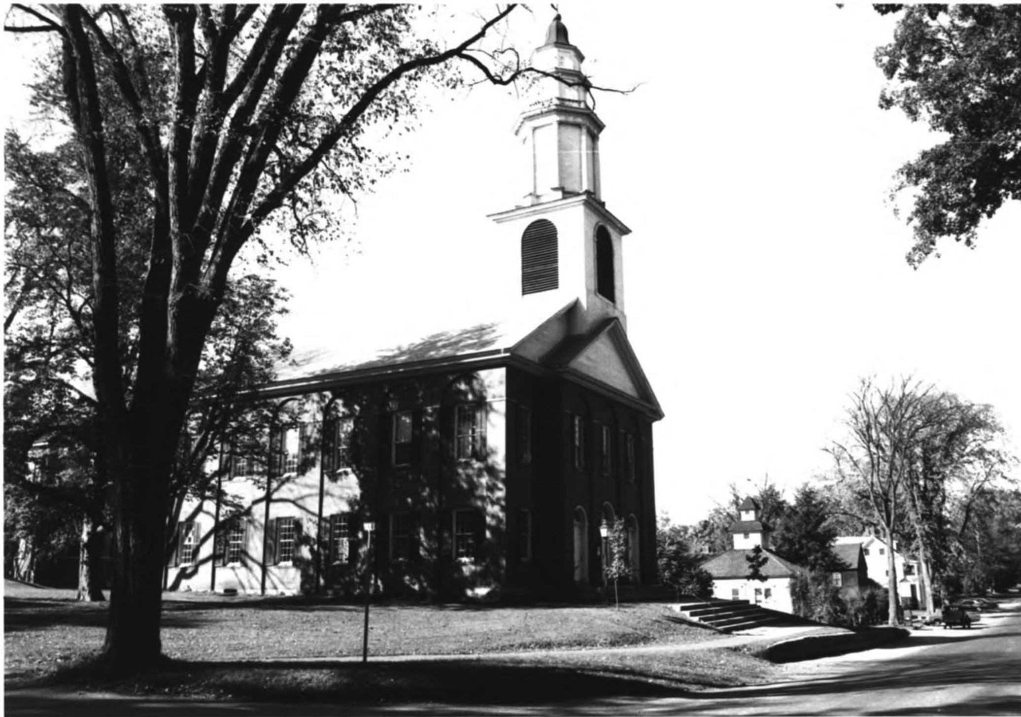
8. Mid-point, west side of "The Street" - north to south (left to right) Brick Church, Post Office, Broom Shop, Deerfield Inn. (Photographer: Polly M. Rettig, NPS Landmark Review Project, Sept. 1974) Photo from NPS Focus, http://nrhp.focus.nps.gov/
