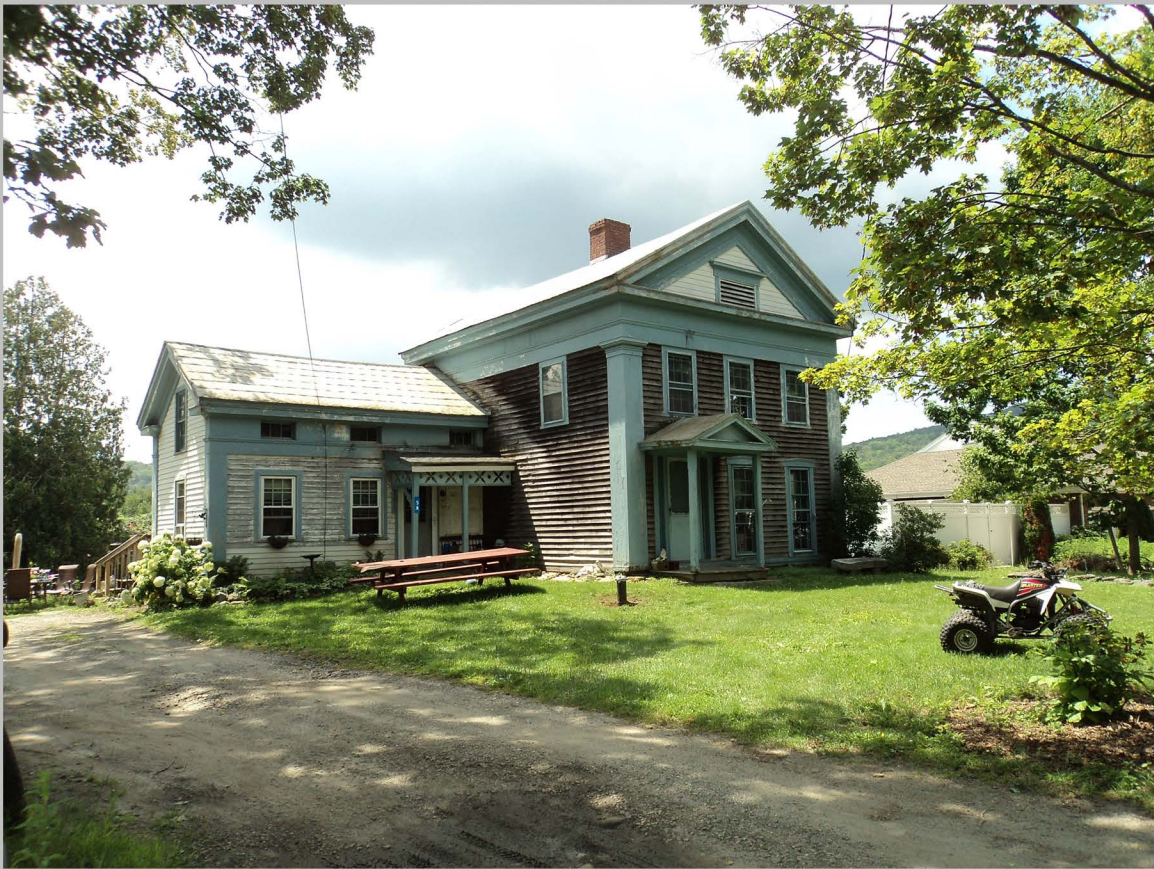
9. 5 Sandisfield Road, Selden & Catherine Allyn House, view to south.
