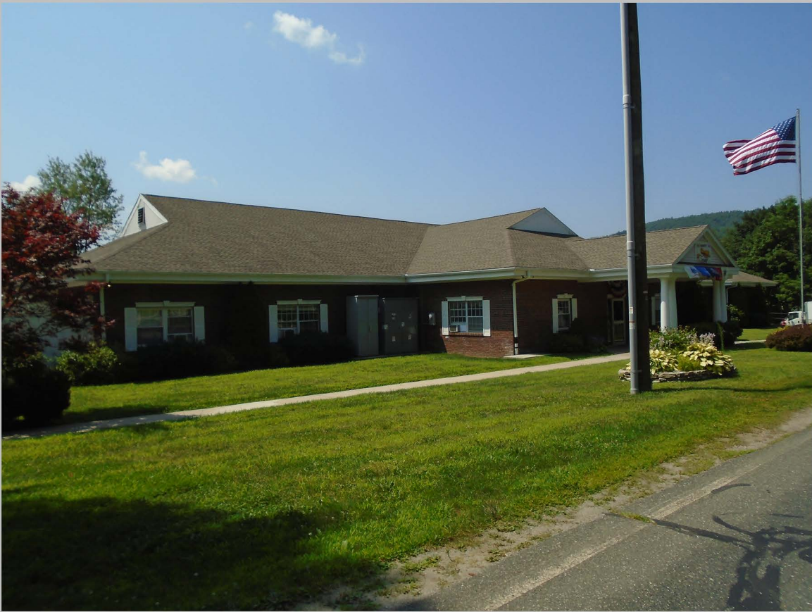
49. 7 Sandisfield Road, Berkshire Rehabilitation Center, view to southwest (July 2019).
