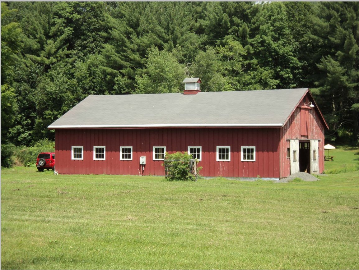
33. 22 Sandisfield Road, barn (ca. 1950), view to northwest.
