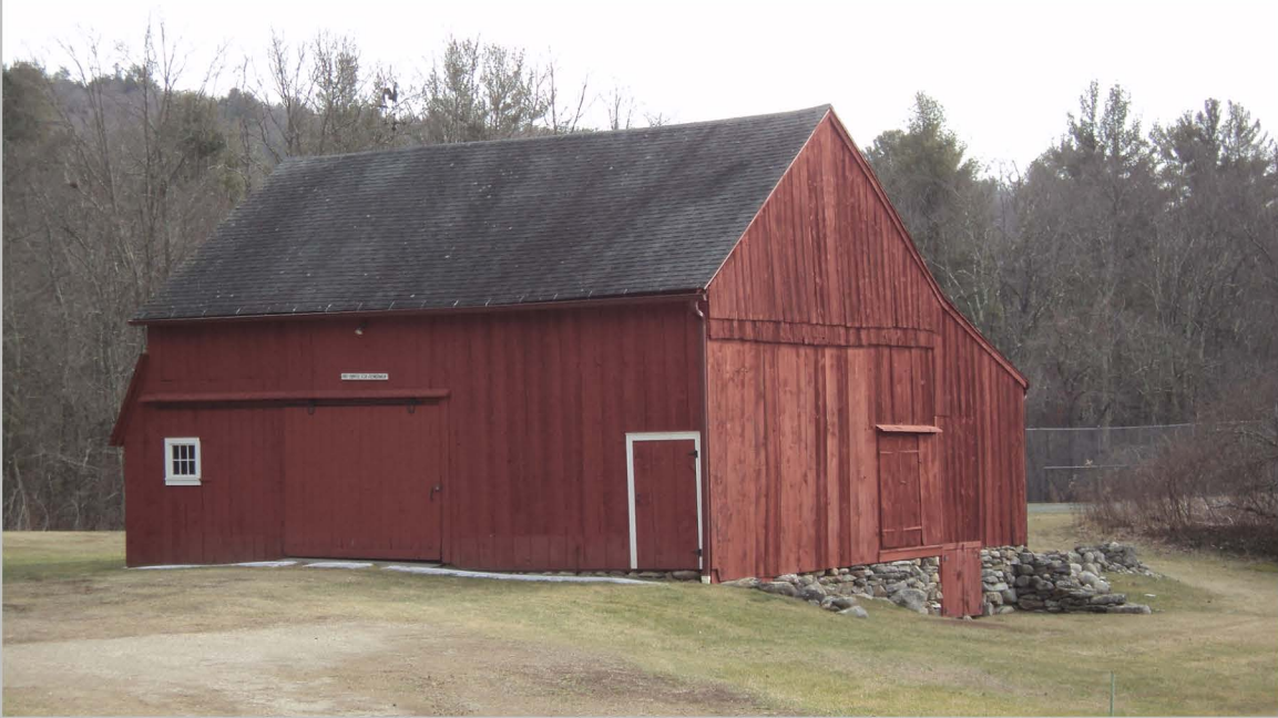
31. 15 Sandisfield Road, Joseph & Mary Denslow Barn, view to southeast (Jan 2016).
