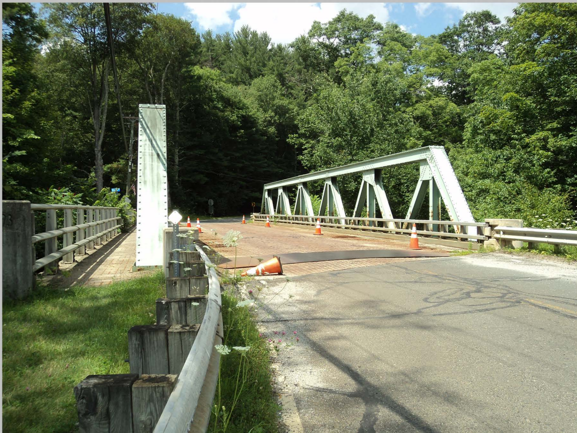
34. Sandisfield Road, Rugg Bridge, view to southwest.
