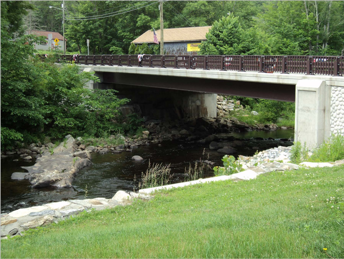
47. North Main Street, Route 8 Bridge, view to north.
