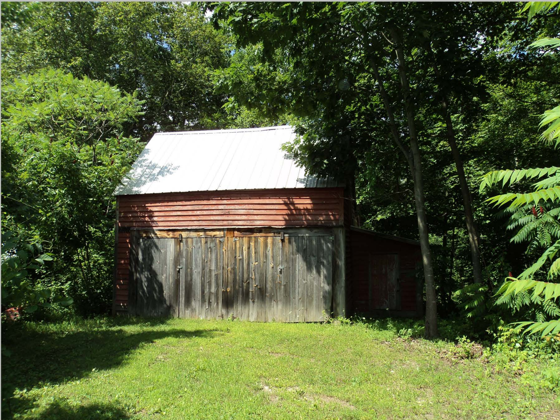
36. 89 South Main Street, Charles Bushnell Carriage Barn.
