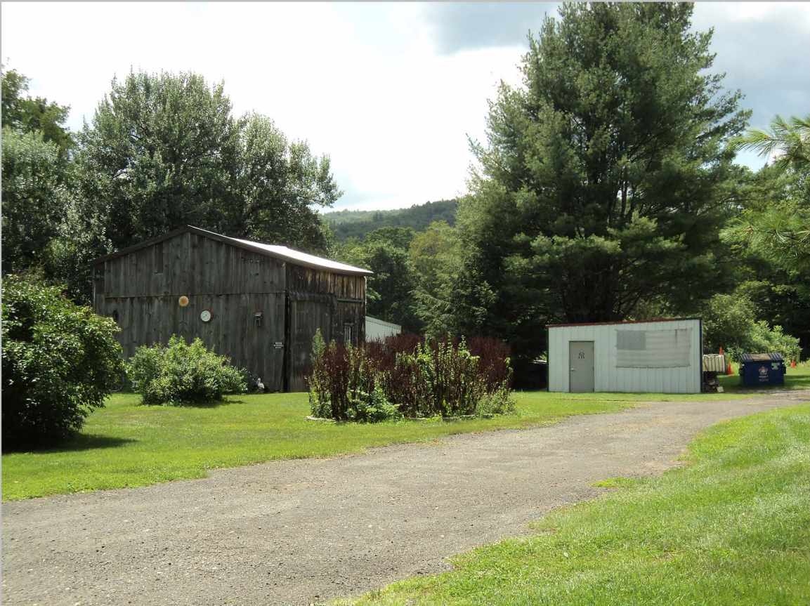
50. 17 Sandisfield Road, Sawmill barn, view to south (Aug 2017).
