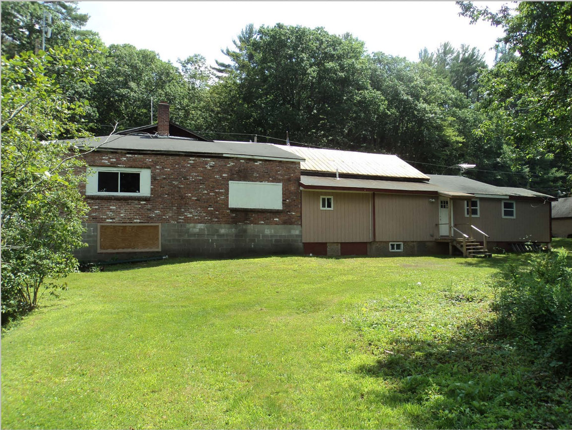
25. 79 South Main Street, New Boston East School/fire station, view to east.
