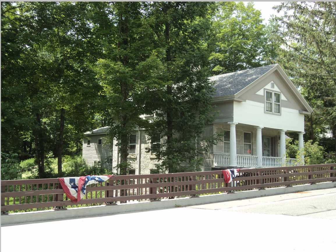
20. 97 North Main Street, Loyal and Abigail Humphrey House, view to south.
