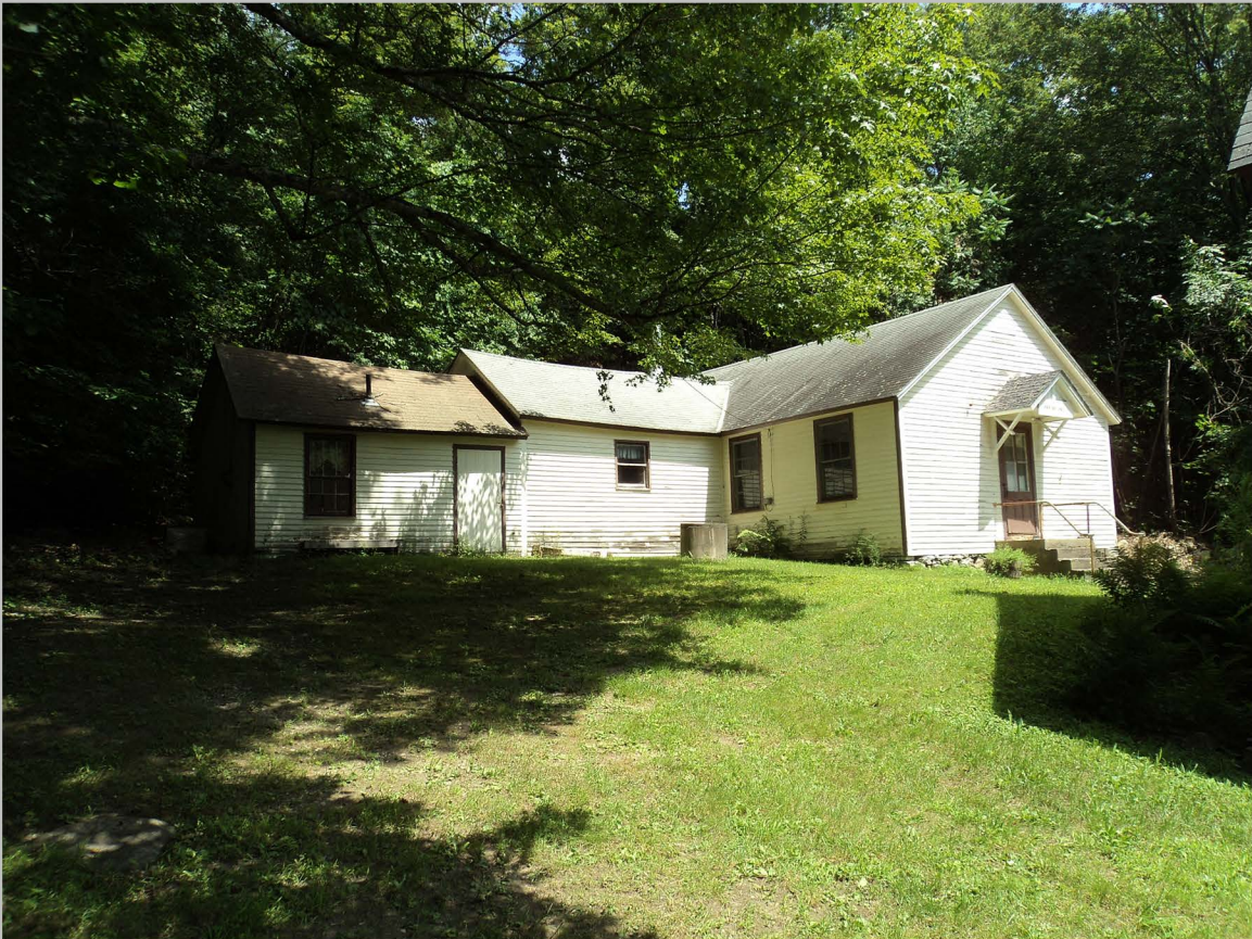
44. 4 Sandisfield Road, New Boston Congregational Church Parish Hall, view to northeast.
