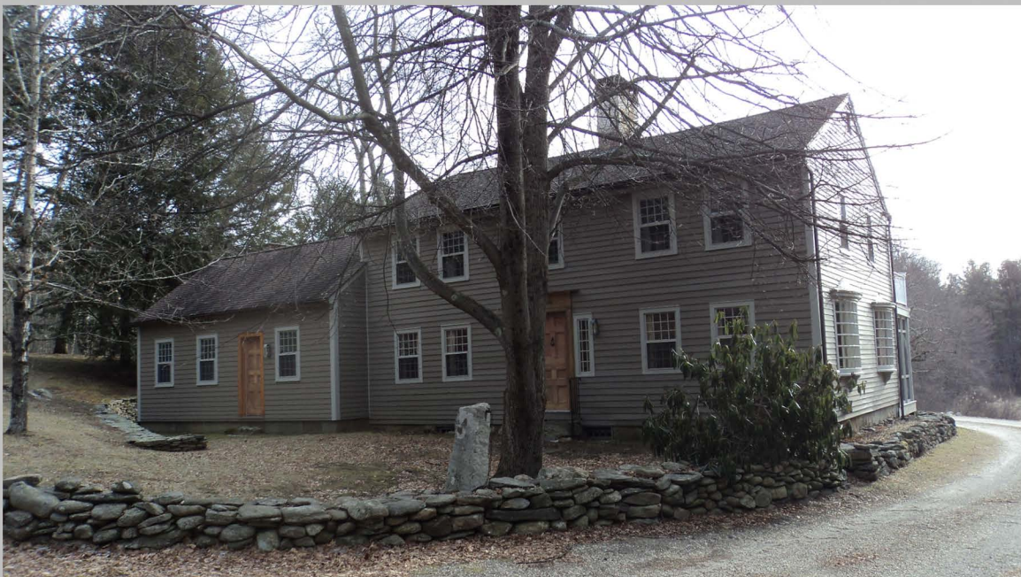
6. 15 Sandisfield Road, Joseph & Mary Denslow House, view to south (Jan 2016).
