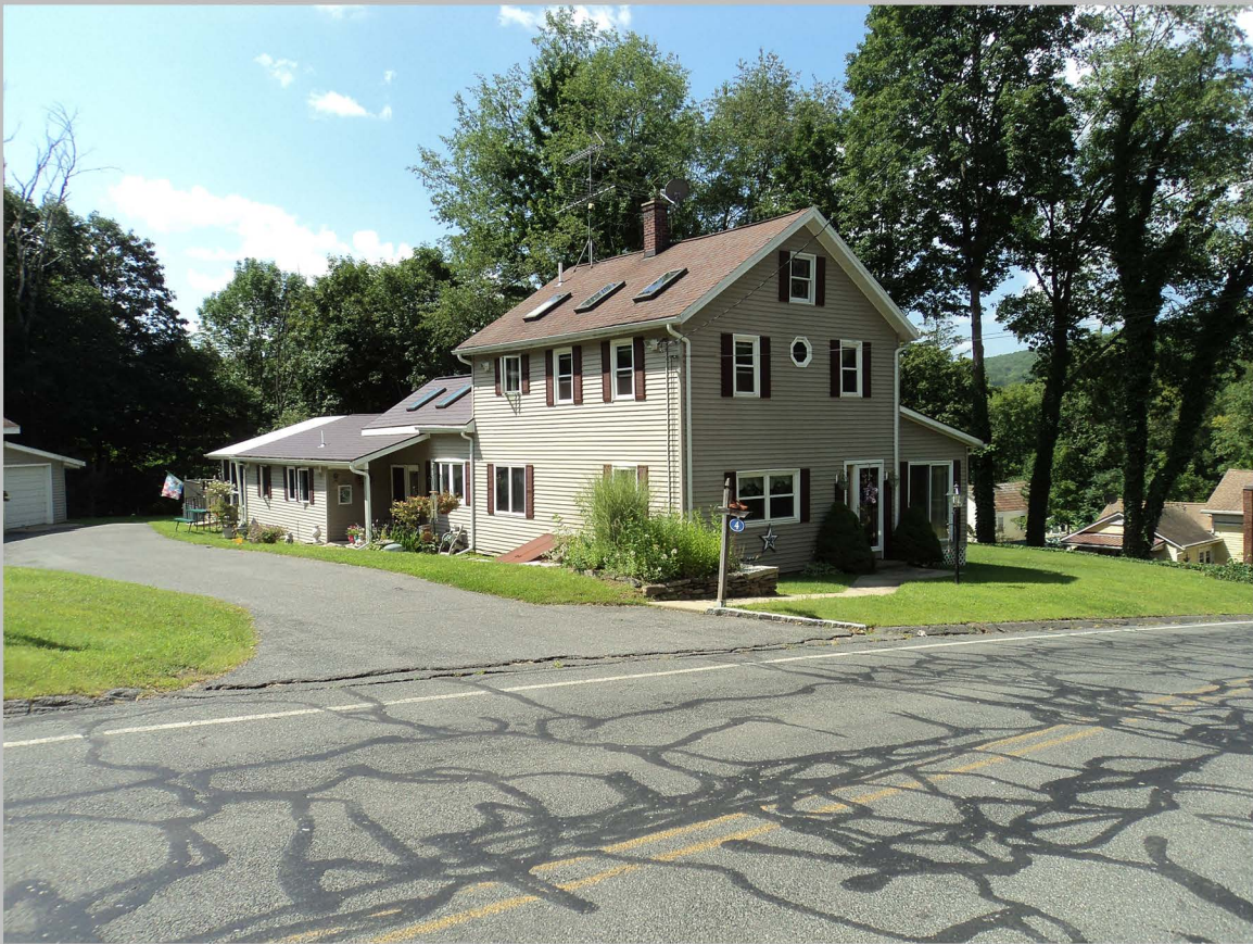
19. 4 Tolland Road, Burrall & Elizabeth Thatcher House, view to southwest.
