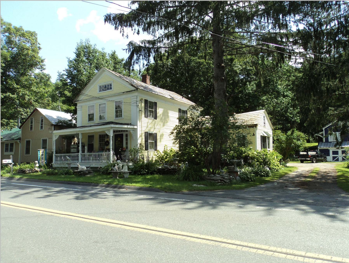
21. 106 South Main Street, Franklin & Louisa Bartholomew House, view to northeast.
