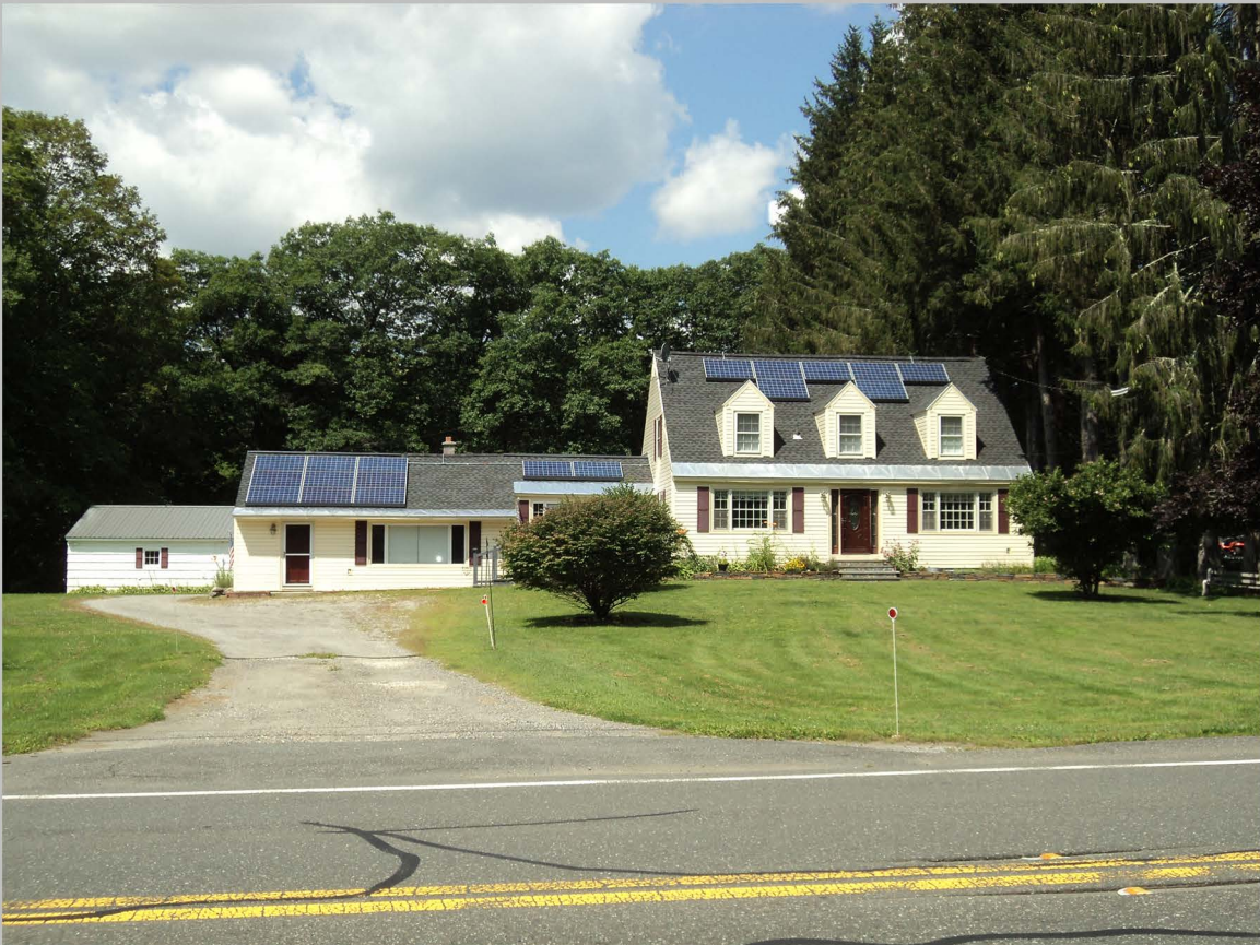
30. 83 South Main Street, George & Mary Lundgren House, view to northwest.
