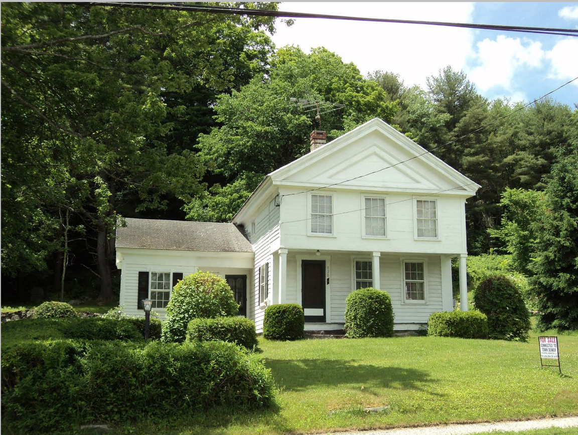
13. Asenata and George Norton House, 120 South Main Road, view to northwest.
