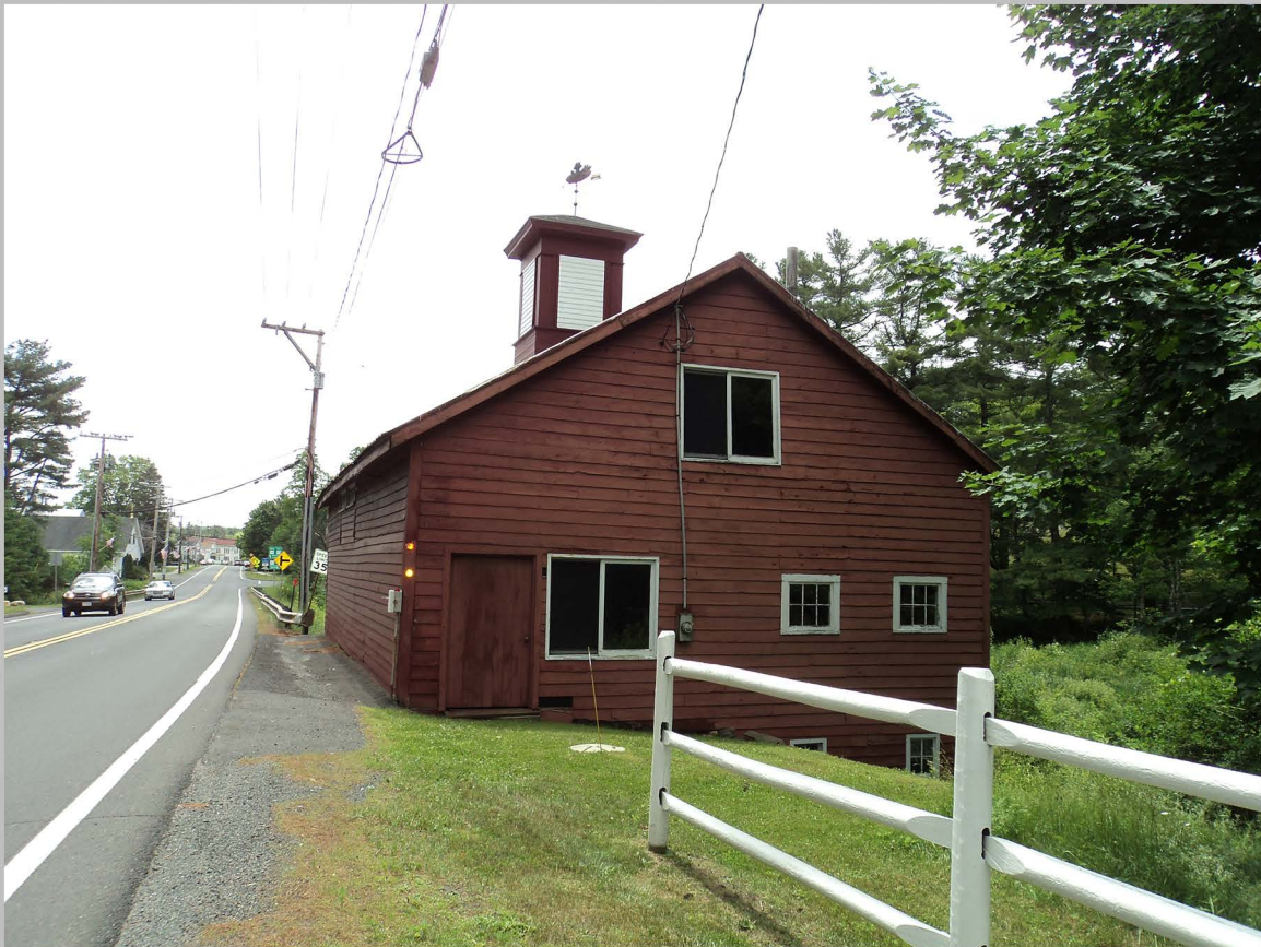
9. Mrs. Almora Merritt's Barn, 137 North Main Road, view to south.
