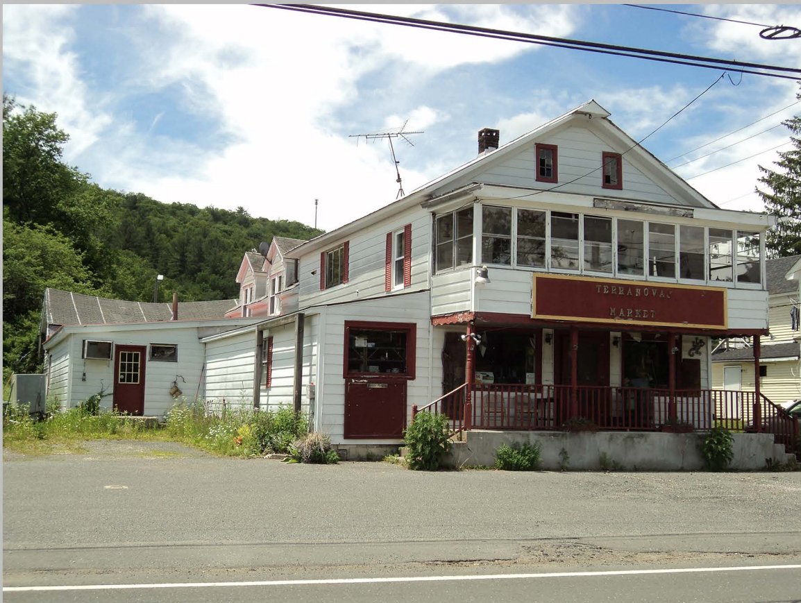
17. Pickett and Sears Store, 14 South Main Road, view to southwest.
