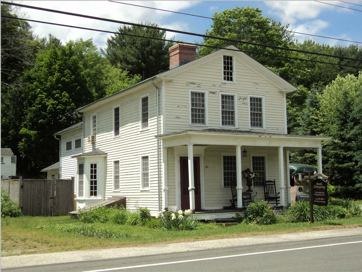
7. L. J. Strickland House 70 South Main Road, view to northwest.
