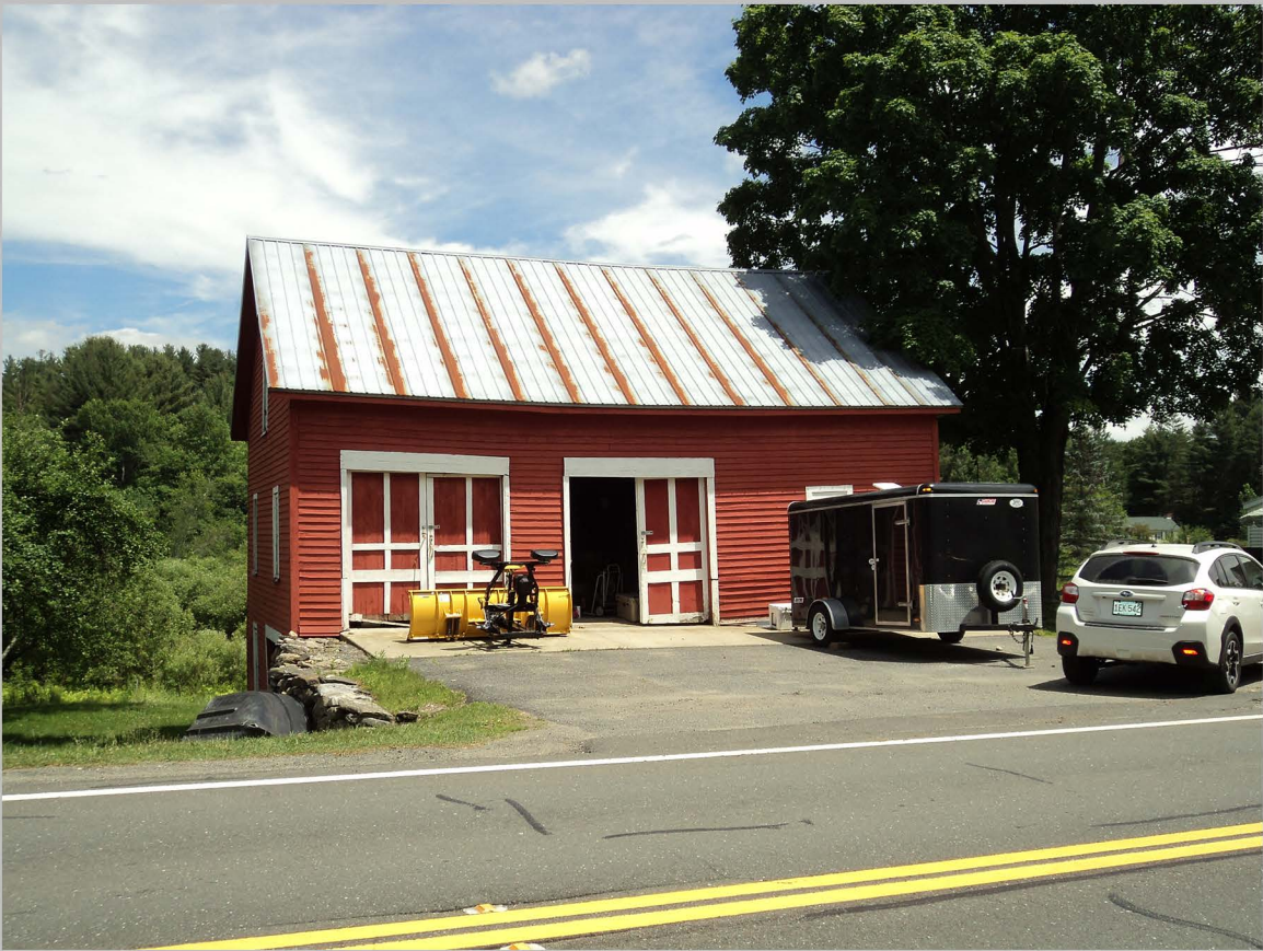
11. Porter and Carter Cabinet Shop, 73 South Main Road, view to southeast.
