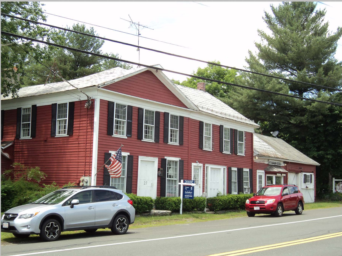
2. Squire Seymour Store, 27 North Main Road, view to west.
