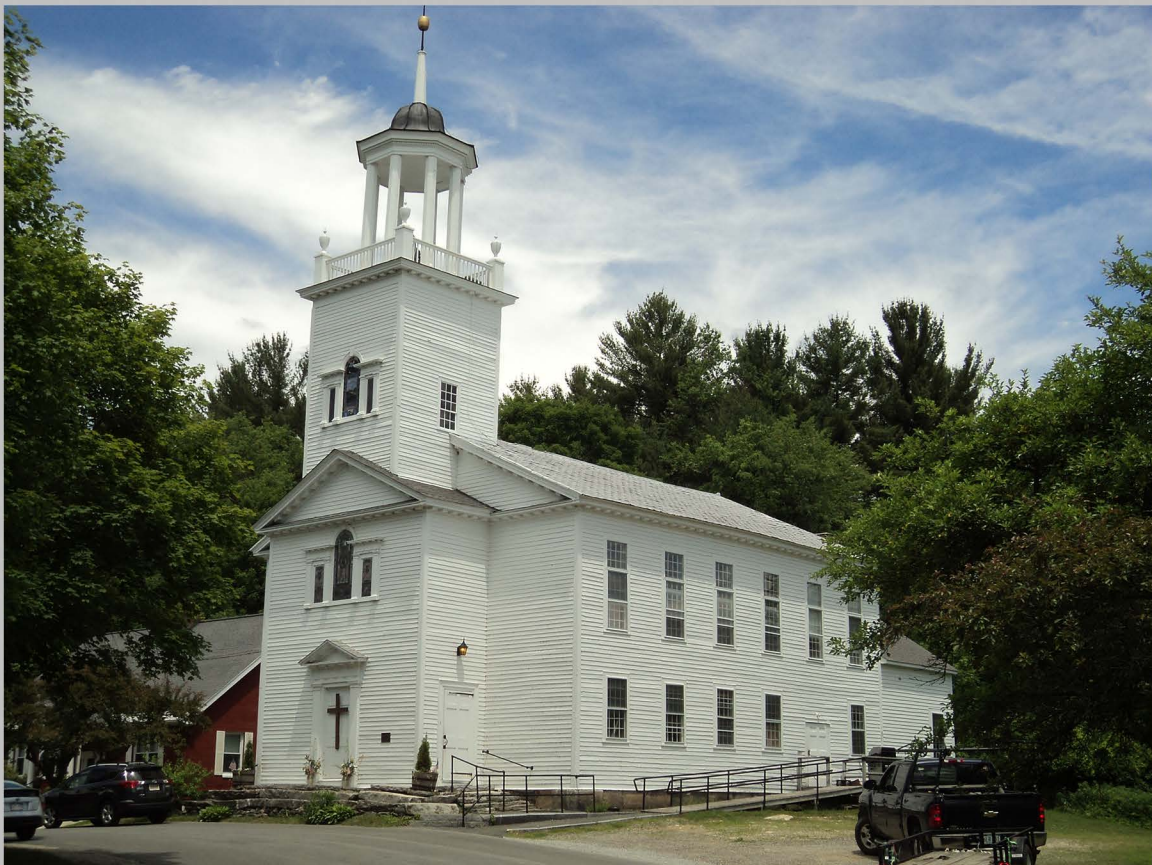
6. Otis First Congregational Church, 46 North Main Road, view to northeast.
