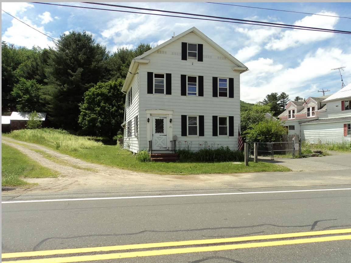
18. Jonathan and Harriet Jackson House, 20 South Main Road, view to west.
