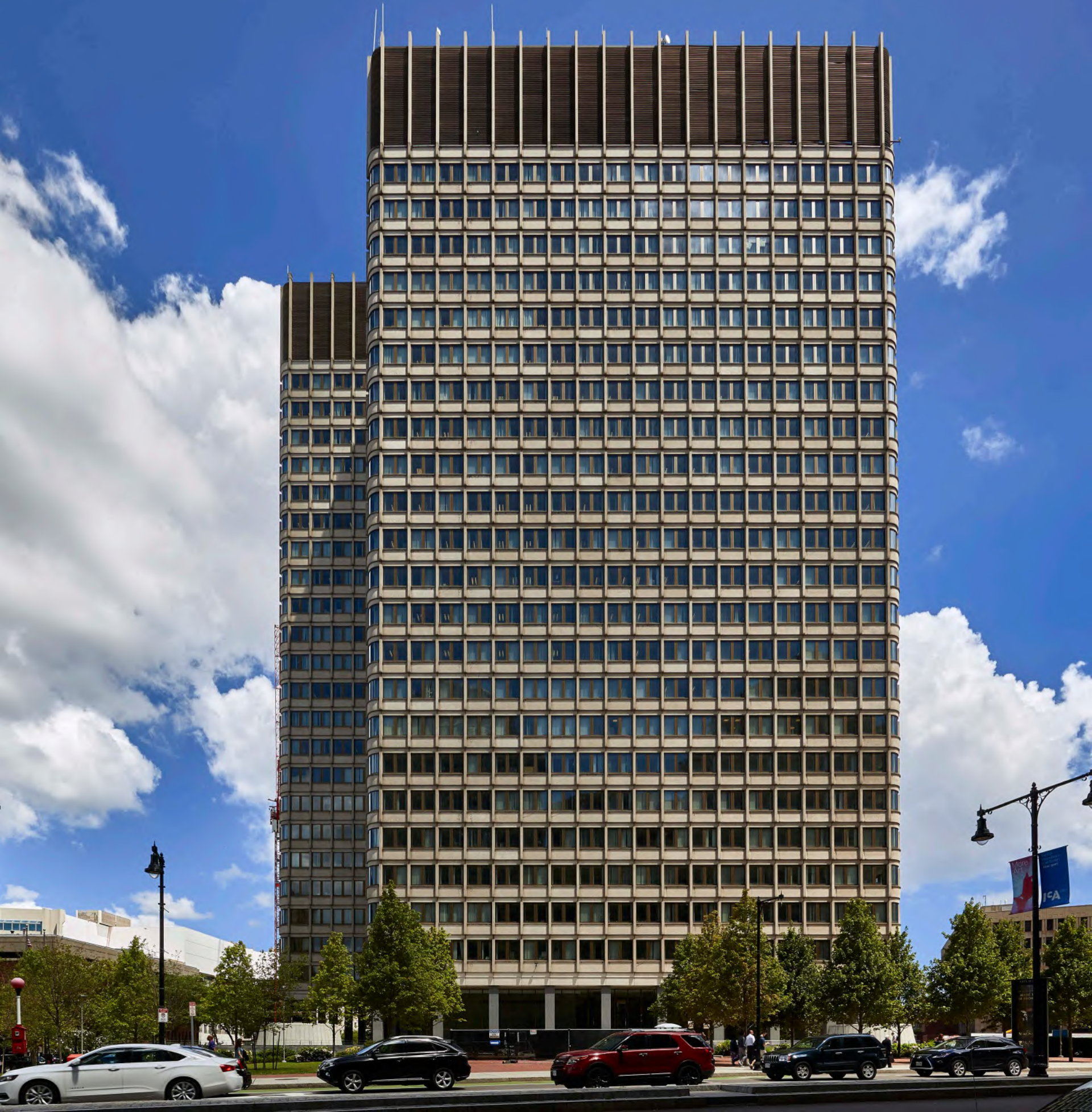
Photo # 10 (MA_Suffolk County_John F Kennedy Federal Building_0010)
