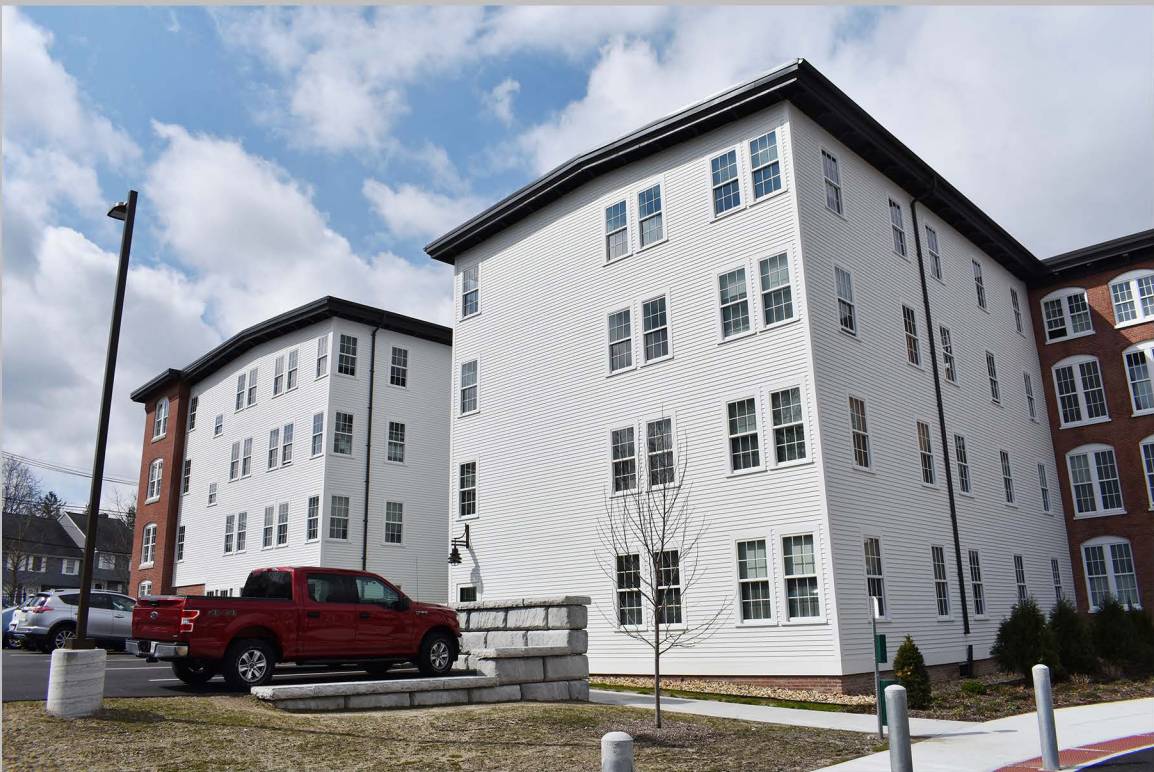
4. View southwest of main factory complex (left to right, Building Nos. 3C, 3, 1A, 1).
