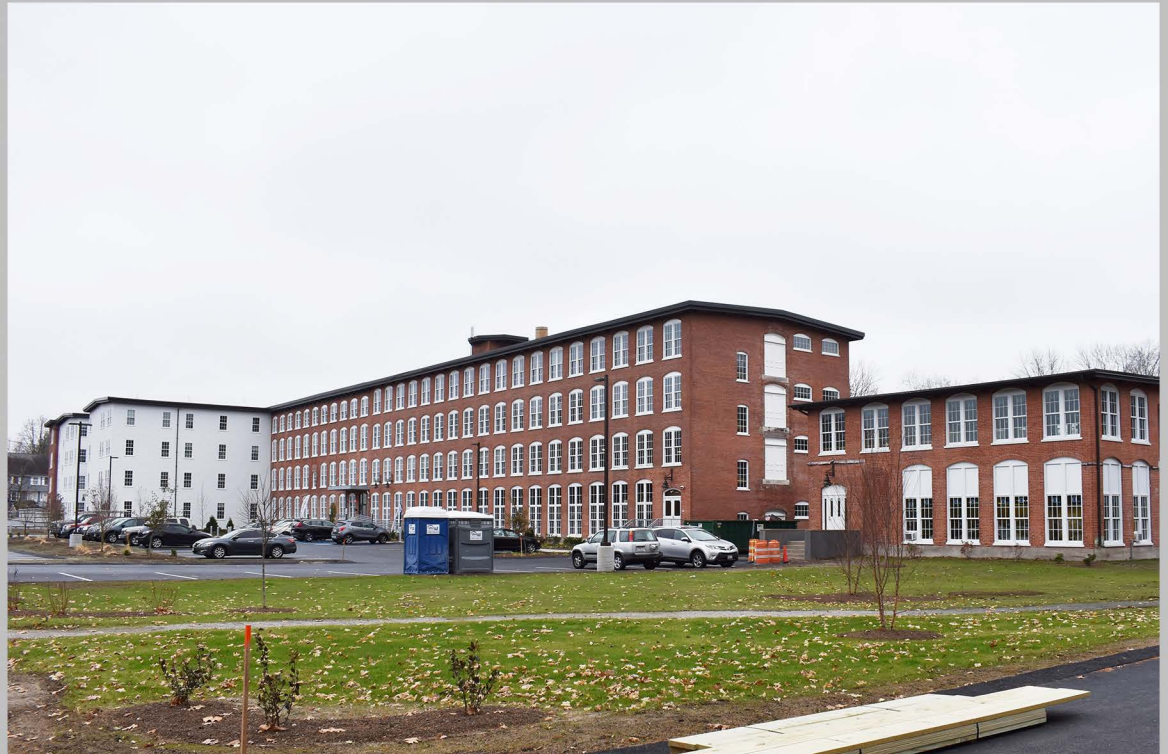
6. View southwest of main factory complex (left to right, Building Nos. 3, 1A, 1, 2, 6).
