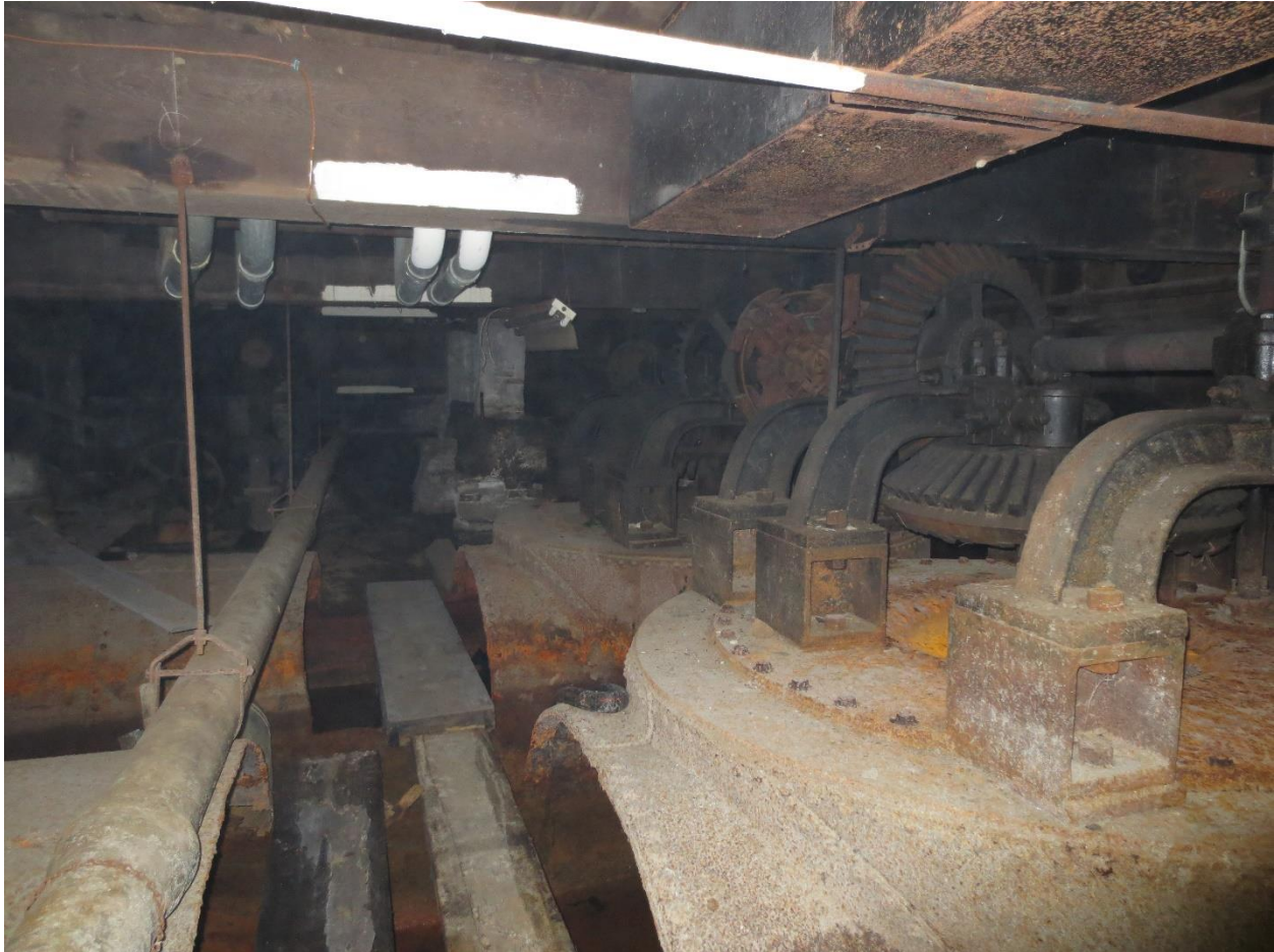
Figure 10 Photograph of the turbines used to generate waterpower for the factory (taken in 2014).
