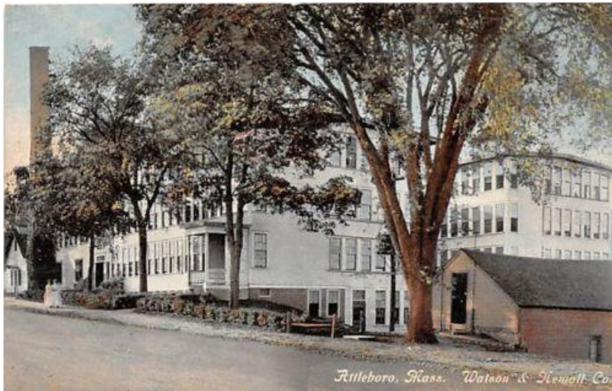
Figure 8. Ca. 1911 postcard. This view shows the south (façade) and east elevations of the Watson, Newell & Company wood-frame buildings from Mechanic Street before the one-bay-deep brick section was added to the façade. (L-R: Building No. 3 and Building No. 1A). A former store house, demolished between 1911 and 1924, is shown at far right. Photograph courtesy of the Attleboro Public Library, Local History Room.
