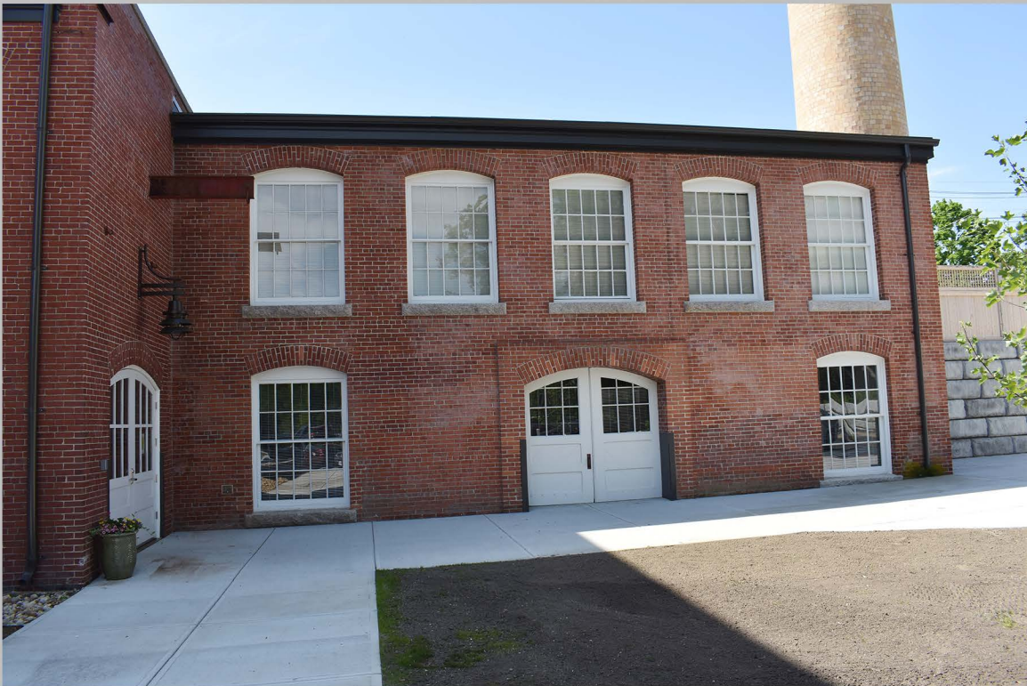
10. View south of Building No. 3B and Smokestack.
