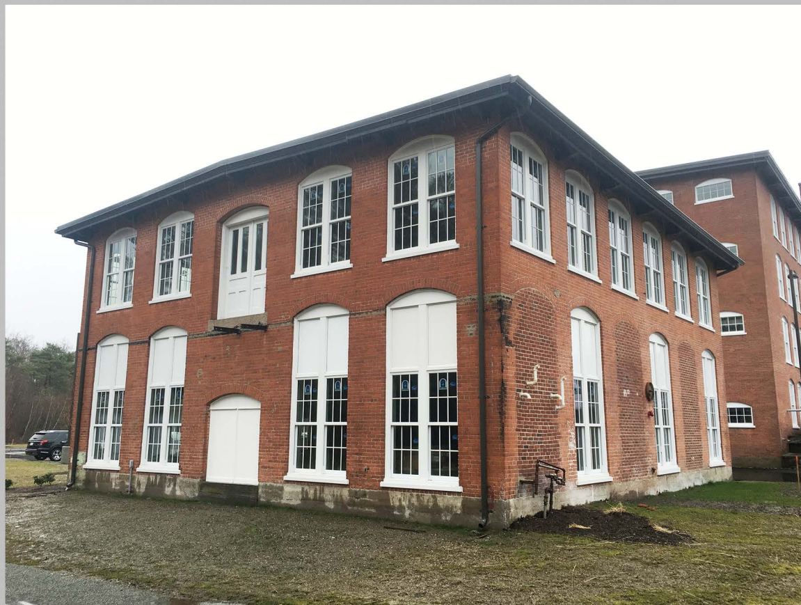
12. View southeast of Building No. 6. Photographed April 2020.
