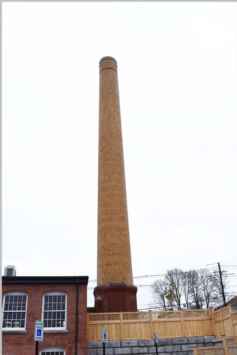
11. View south of Building No. 3B and Smokestack. Photographed November 2019.
