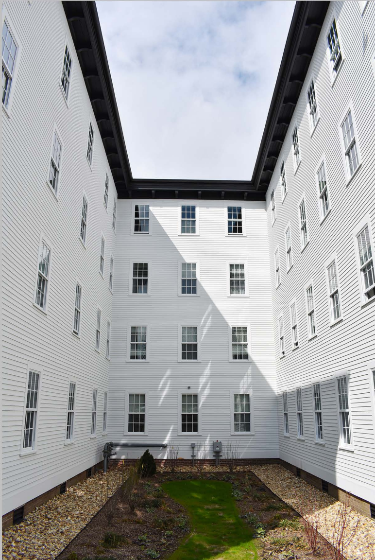
5. View west of main factory complex (left to right, Building Nos. 3, 1, 1A).
