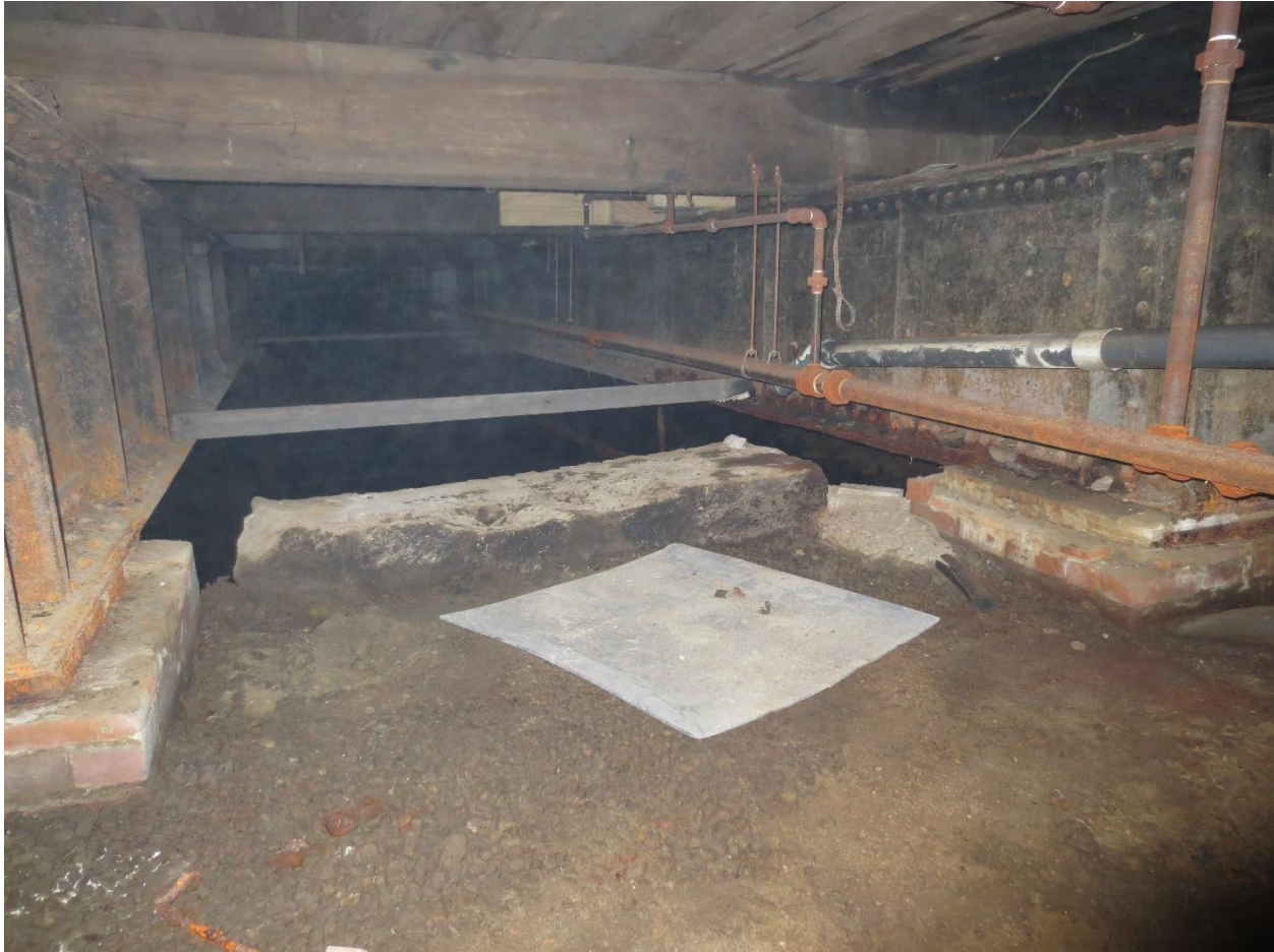
Figure 9. Photograph of former sluiceway beneath Building No. 1 (taken in 2014).
