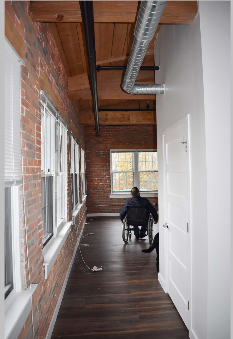
20. View of Machine Shop interior, second floor (Unit 220).
