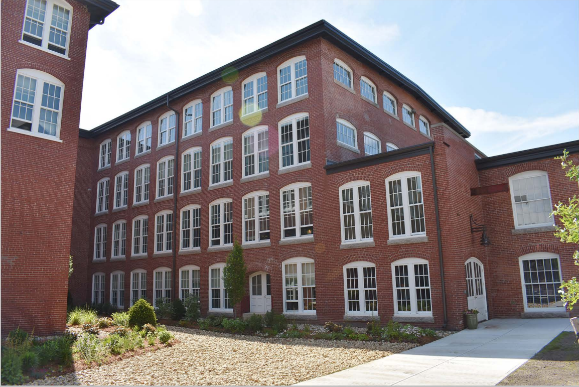
9. View southeast of Buildings No. 3A and 3B.
