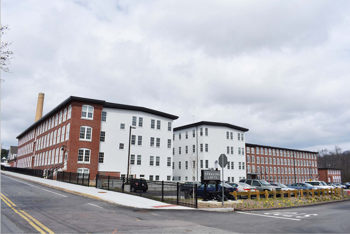
1. View northwest of main factory complex (left to right, Building Nos. 3C, 3, 1A, 1, 2, 6).
