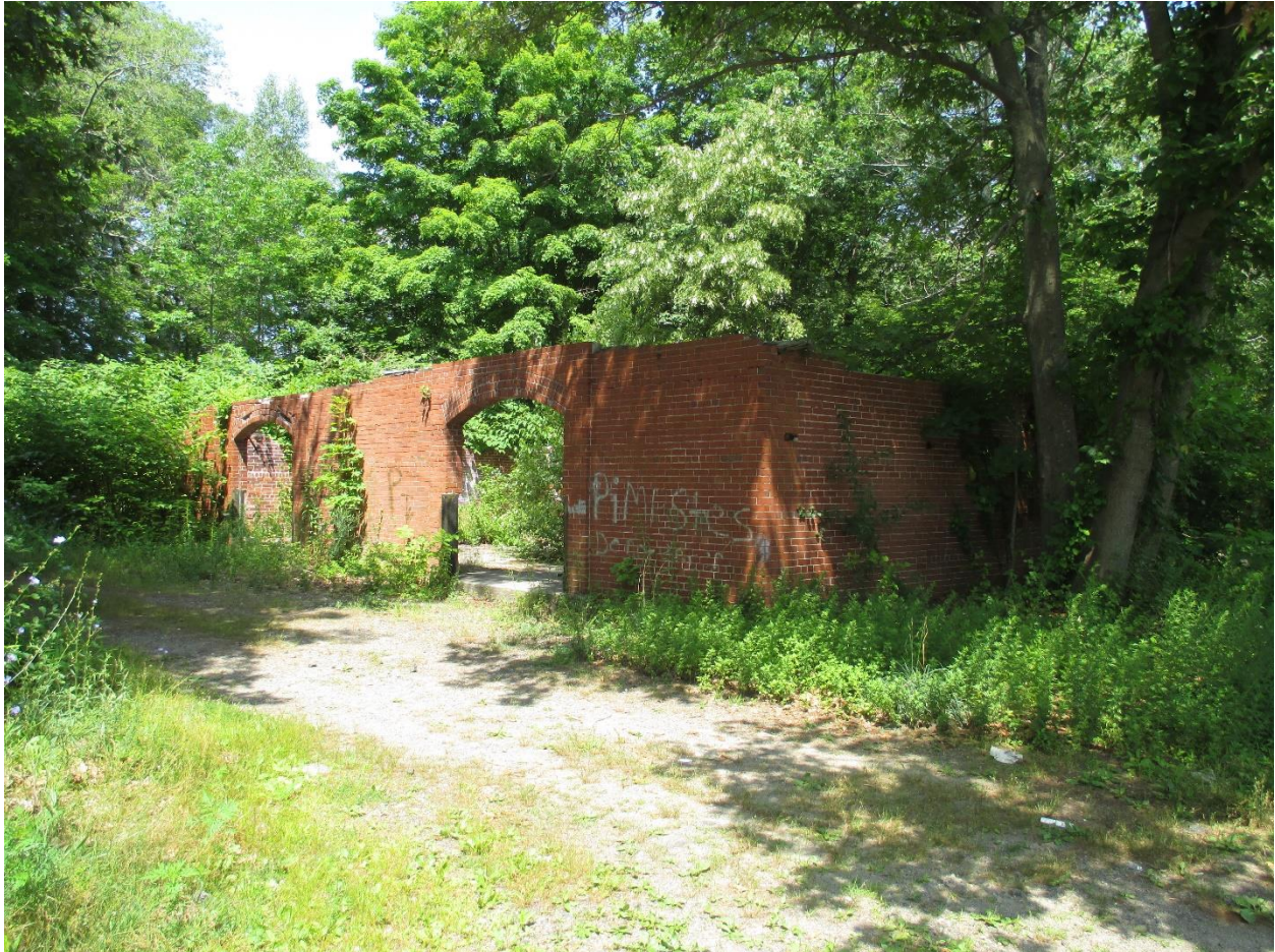
Figure 11 Photograph of the storage building remains before demolition (taken in 2014).
