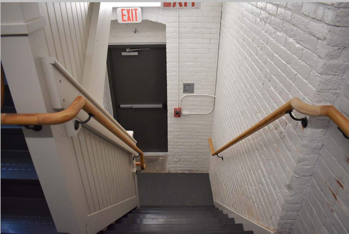
16. View of Tower stair, Building No. 1 interior.
