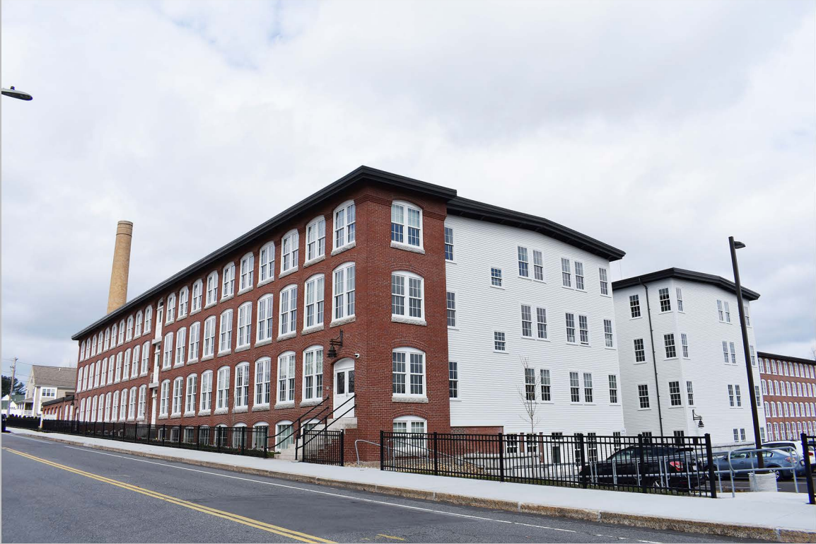
3. View northwest of main factory complex (left to right, Building Nos. 3C, 3, 1A, 1).
