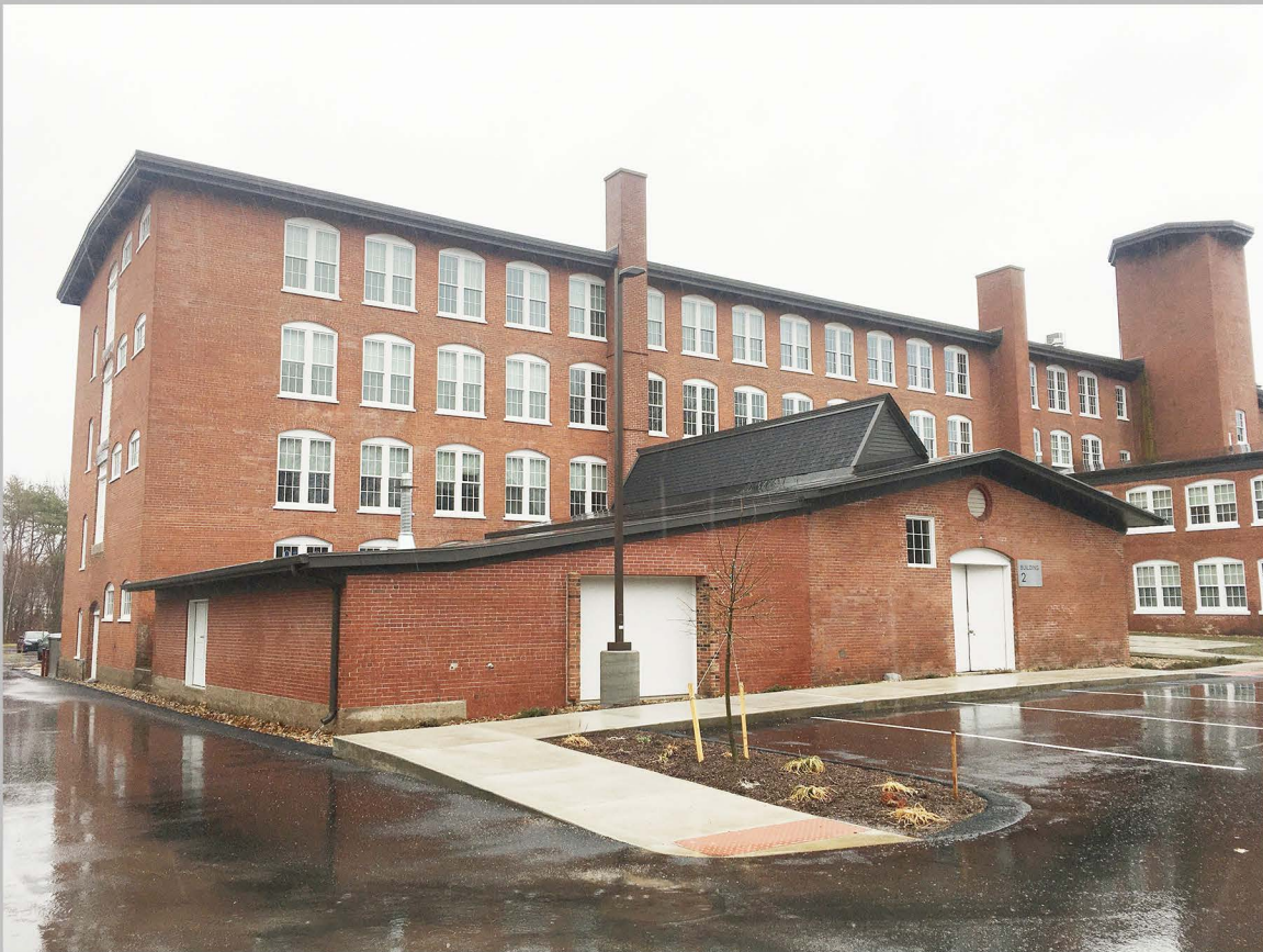
7. View southeast of main factory complex (left to right, Building Nos. 2, 4A, 4, Machine Shop, Tower). Photographed April 2020.
