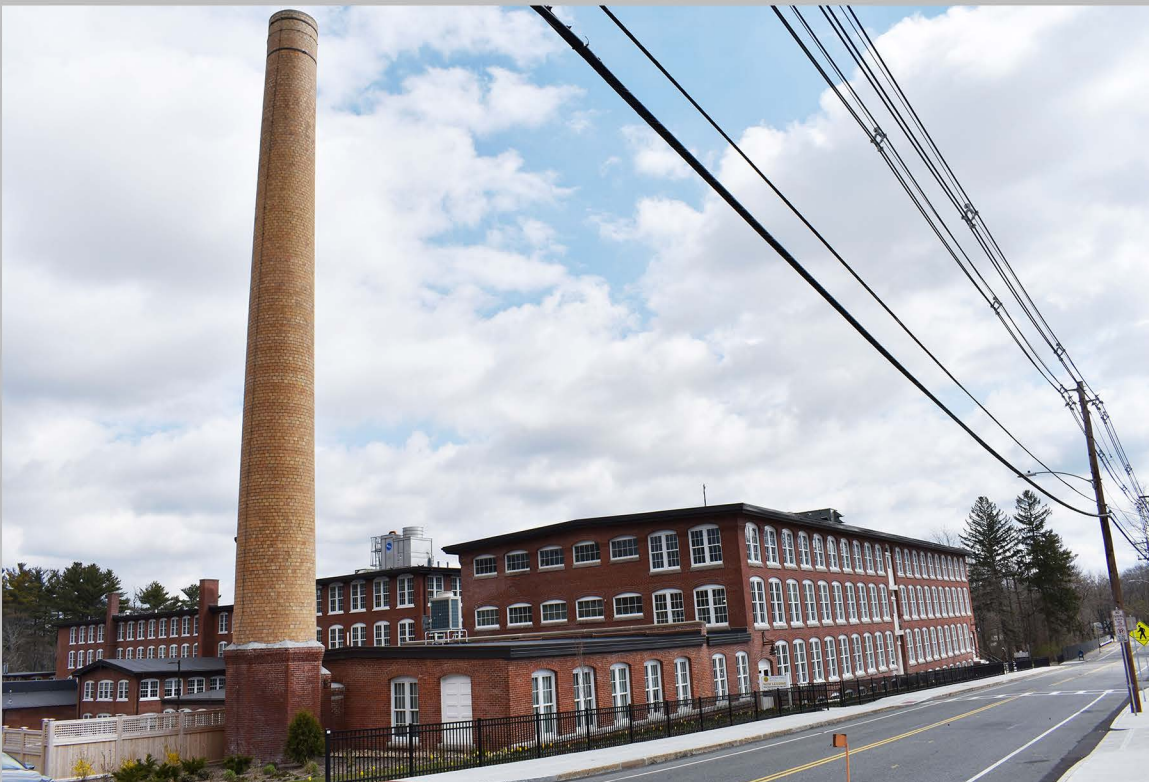
2. View northeast of main factory complex (left to right, Building Nos. 2, 4, Machine Shop, 1B, Smokestack, 3B, 3C).
