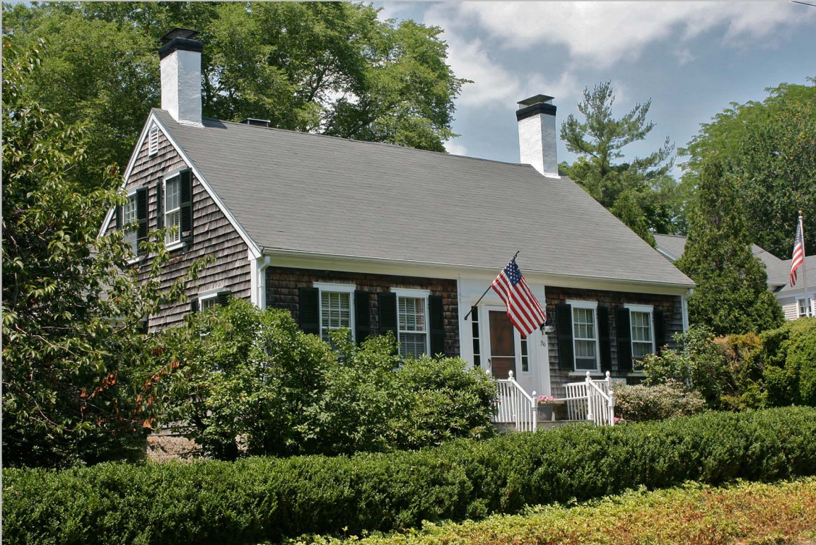
5. 36 Cove Street. Camera facing northwest.
