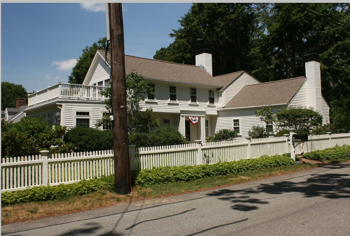
2. 22 Cove Street. Camera facing northwest.
