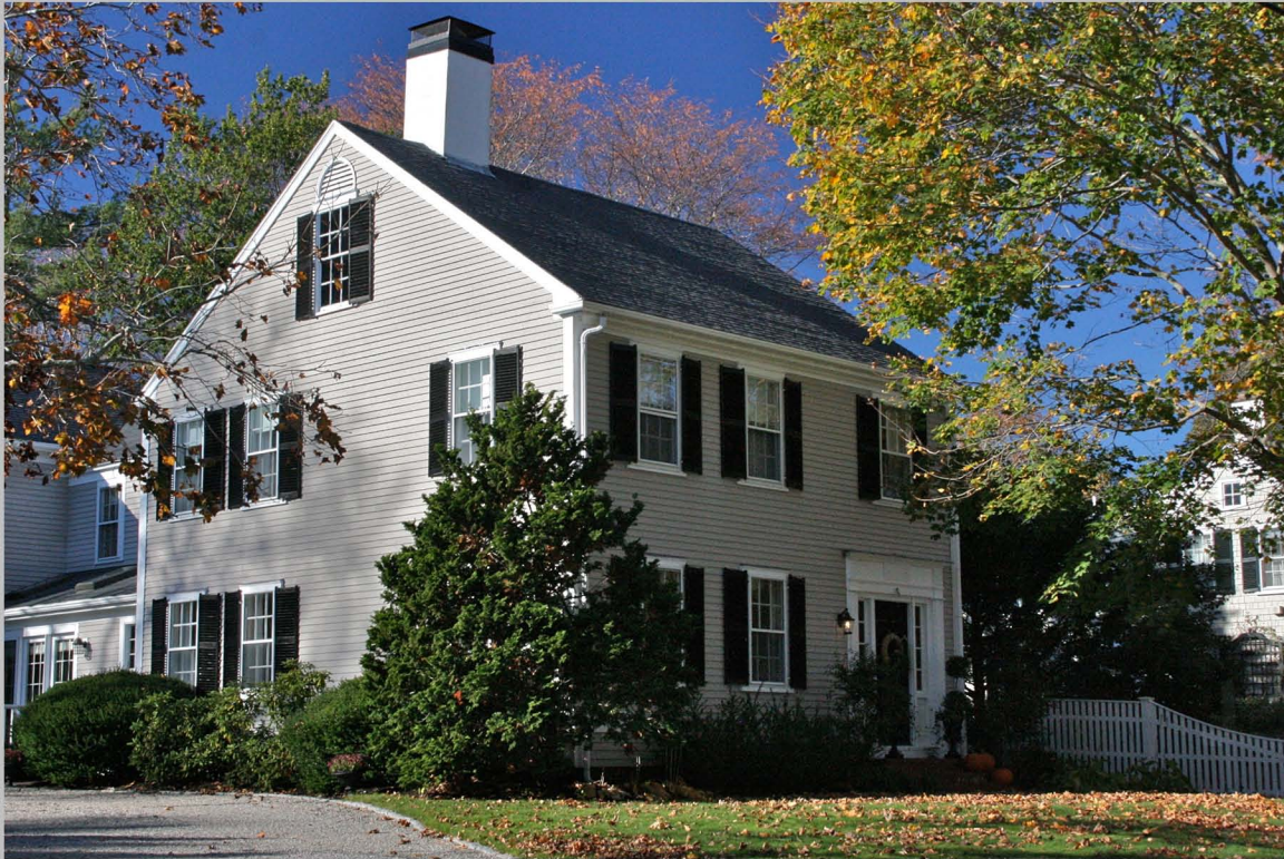
7. 42 Cove Street. Camera facing northwest.
