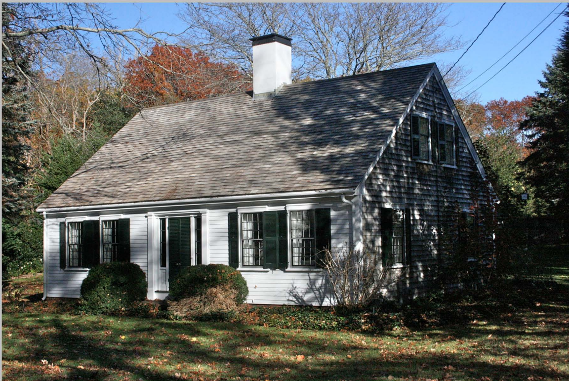
8. 47 Cove Street. Camera facing northeast.
