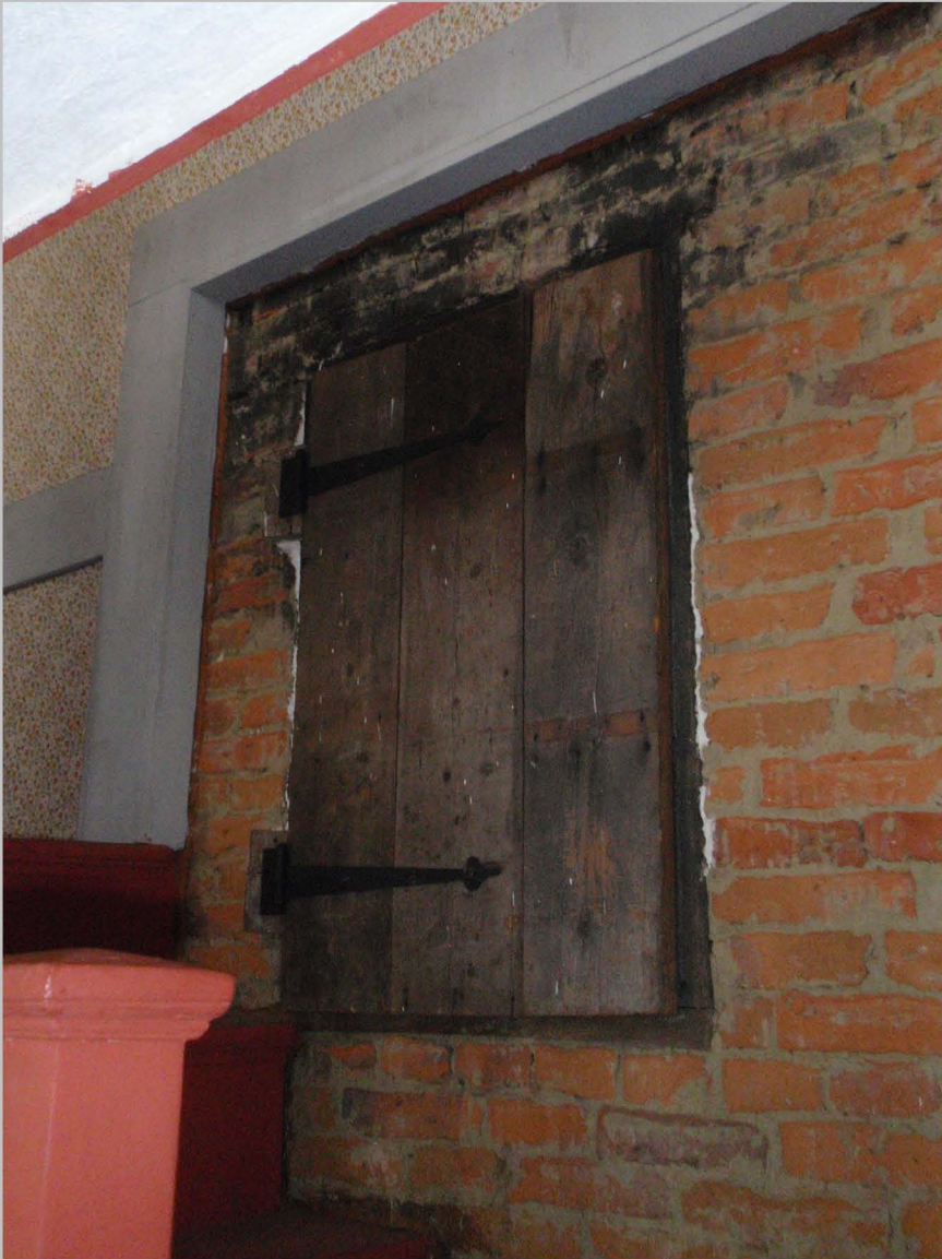
9. Detail of reproduction smokeroom door, camera facing northwest. (March 2013)
