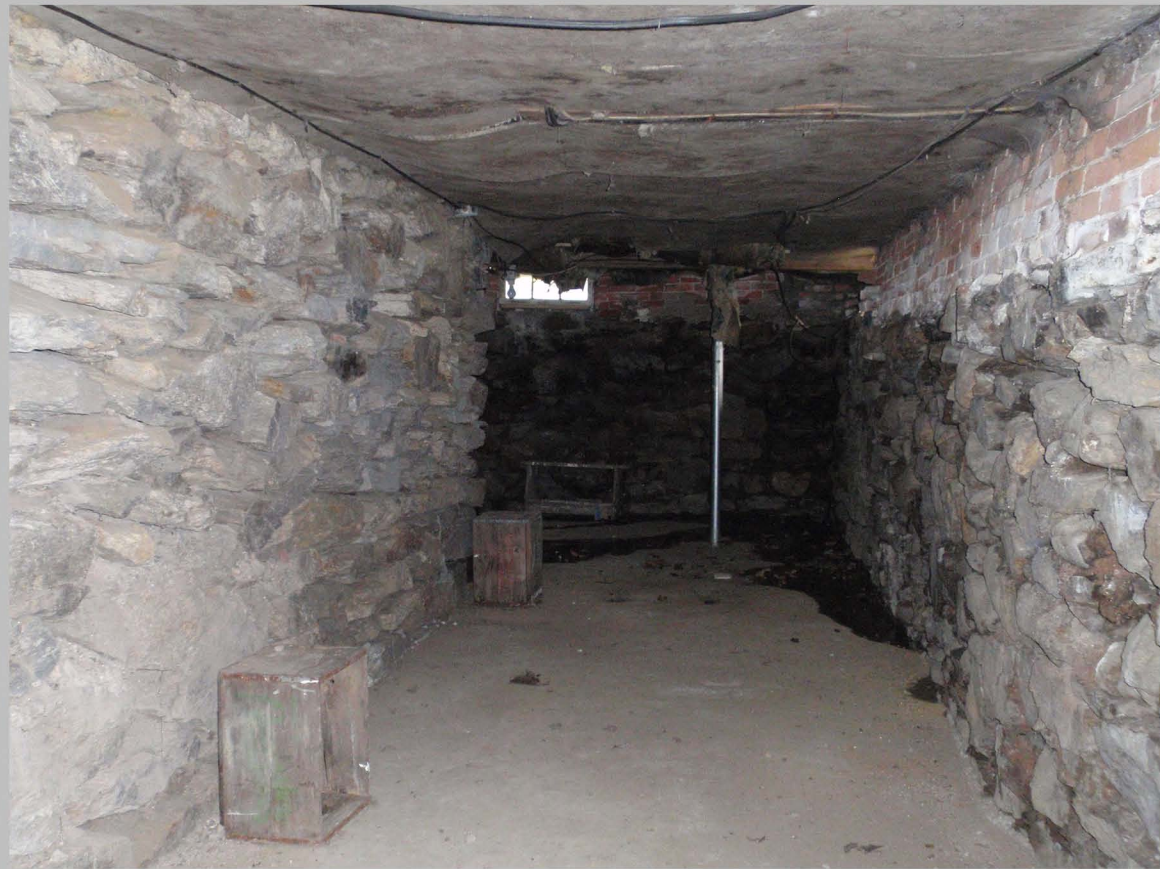
8. South side of basement showing chimney base (left) and foundation (right), camera facing east. (March 2013)
