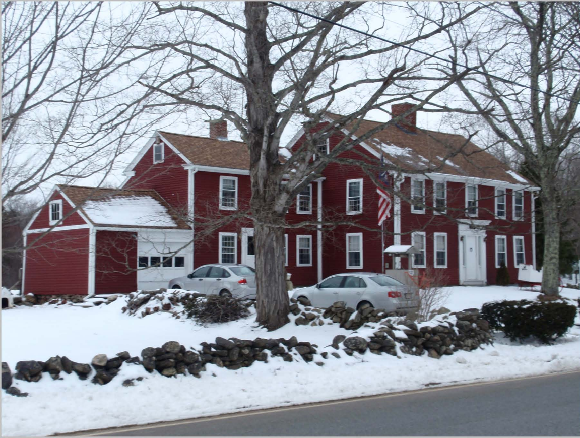
1. South (façade) and west elevations, camera facing northeast. (March 2013)
