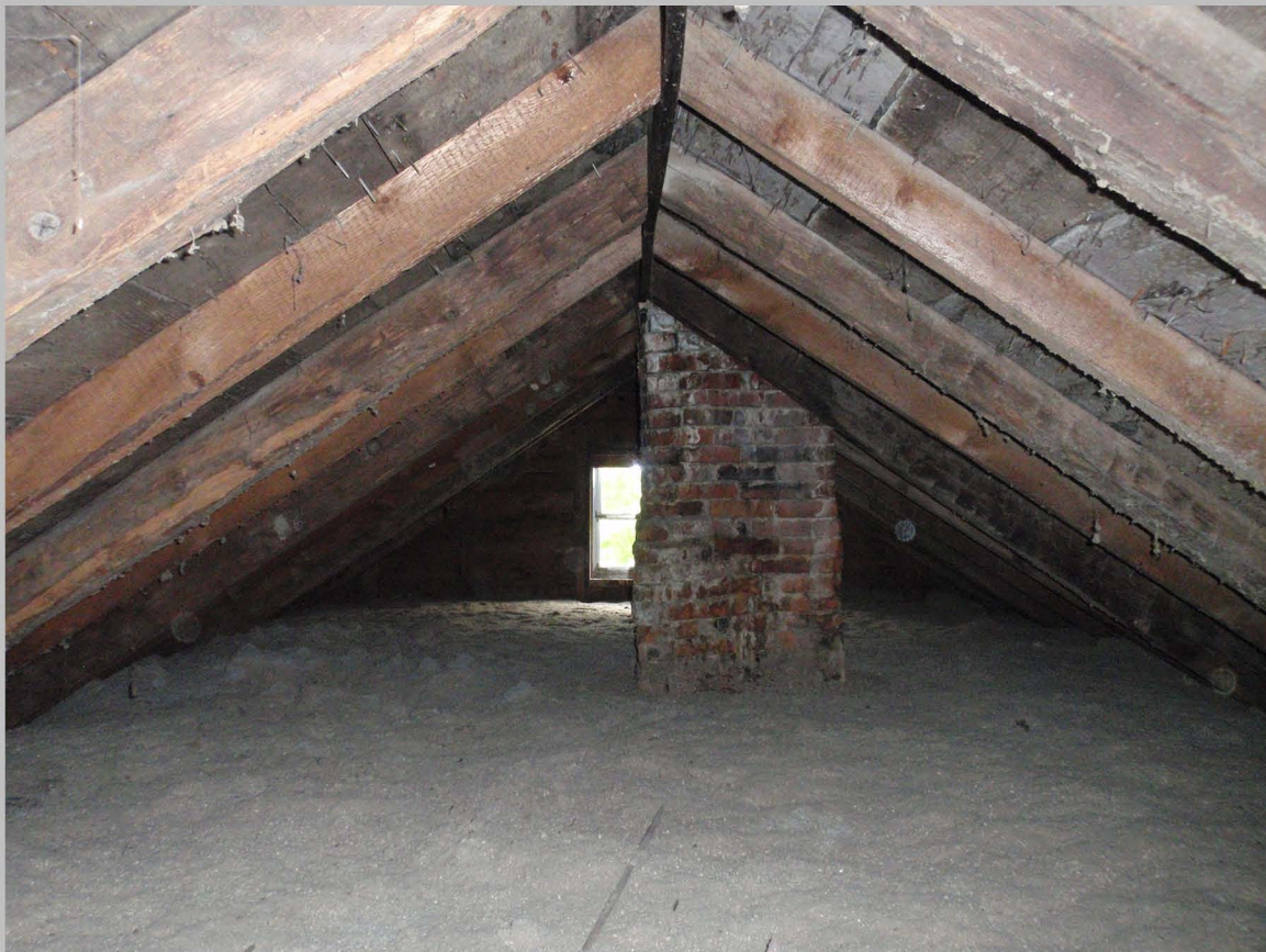
20. Attic/crawl space above the west wing, camera facing west. (May 2013)
