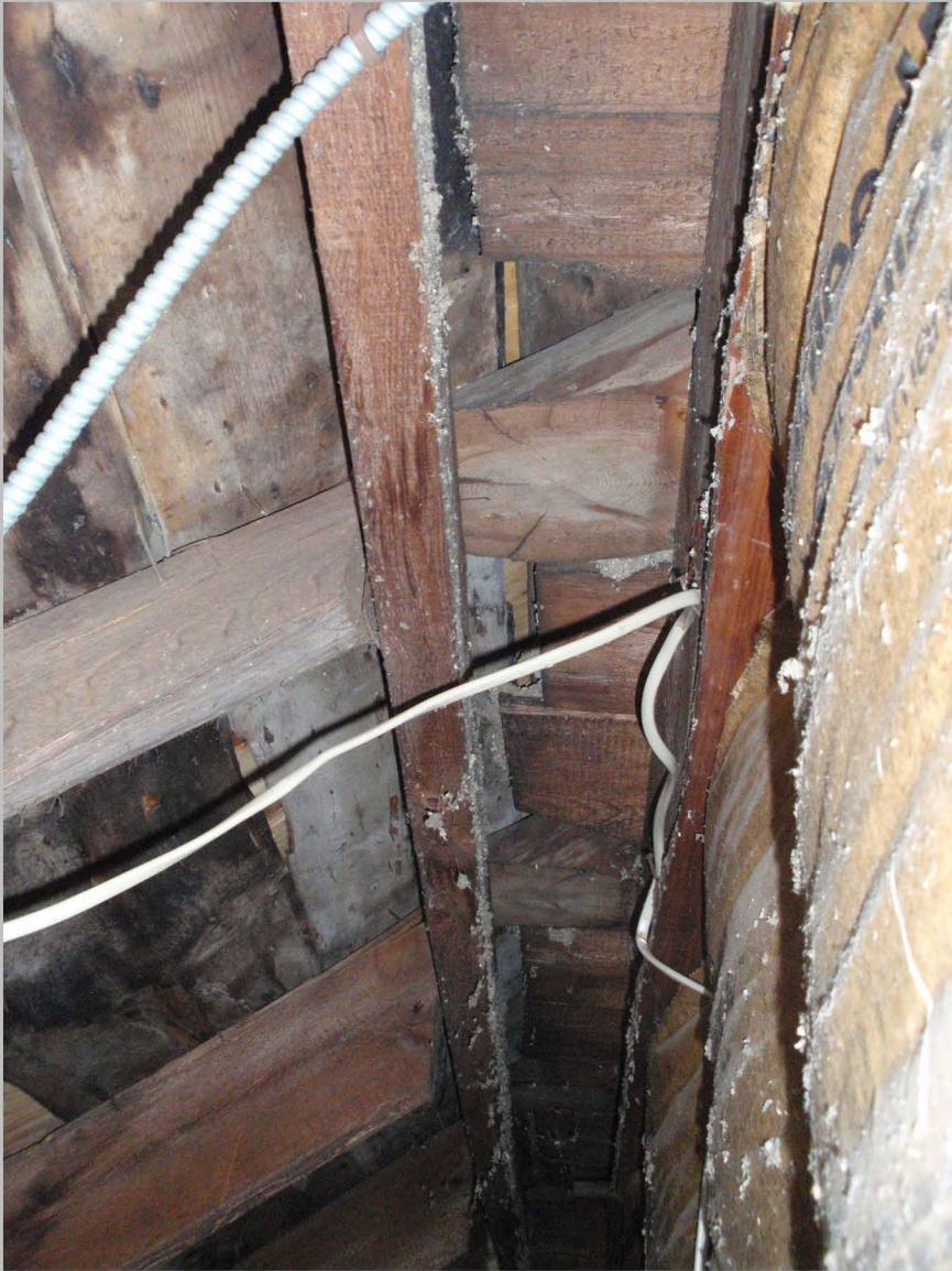
21. Construction in the eastern lean-to showing the rafters of the main body ending (right) and the addition of the lean-to rafters (left), camera facing east. (March 2013)
