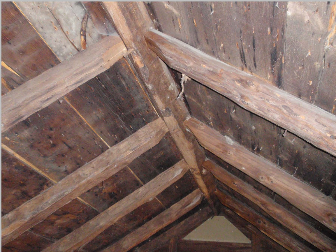
18. The five-sided ridgebeam in the attic, camera facing west. (May 2013)
