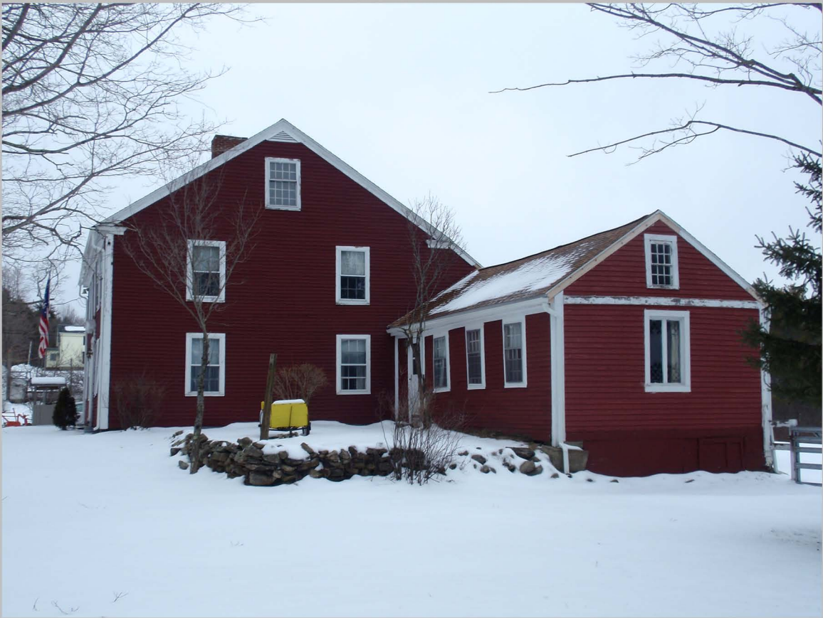
3. East elevation, camera facing west. (March 2013)
