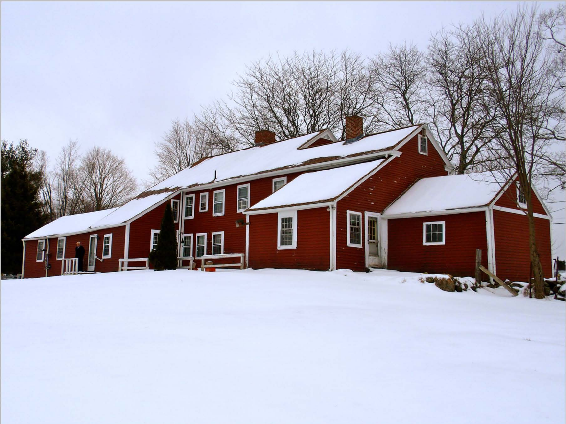
4. North (rear) and west elevations, camera facing southeast. (March 2013)
