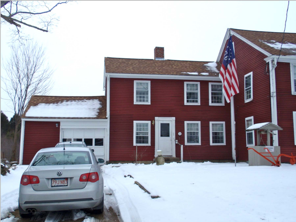
6. South (façade) of west wing and garage, camera facing north. (March 2013)
