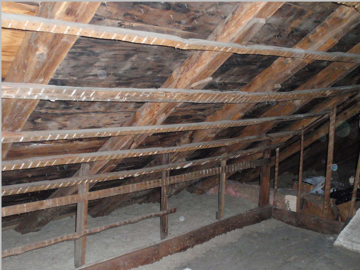
16. Framing of the eastern half of the attic in the main block of the house (horizontal boards since removed), camera facing southwest. (March 2013)
