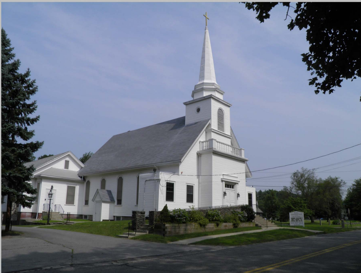
11. Berkley Congregational Church, 13 South Main Street, looking northwest, showing the east façade and southern elevation. The Trinitarian Congregational Chapel (1848, left) and the Methodist Episcopal Church (1875, right) were moved to this site and joined together in 1904.
