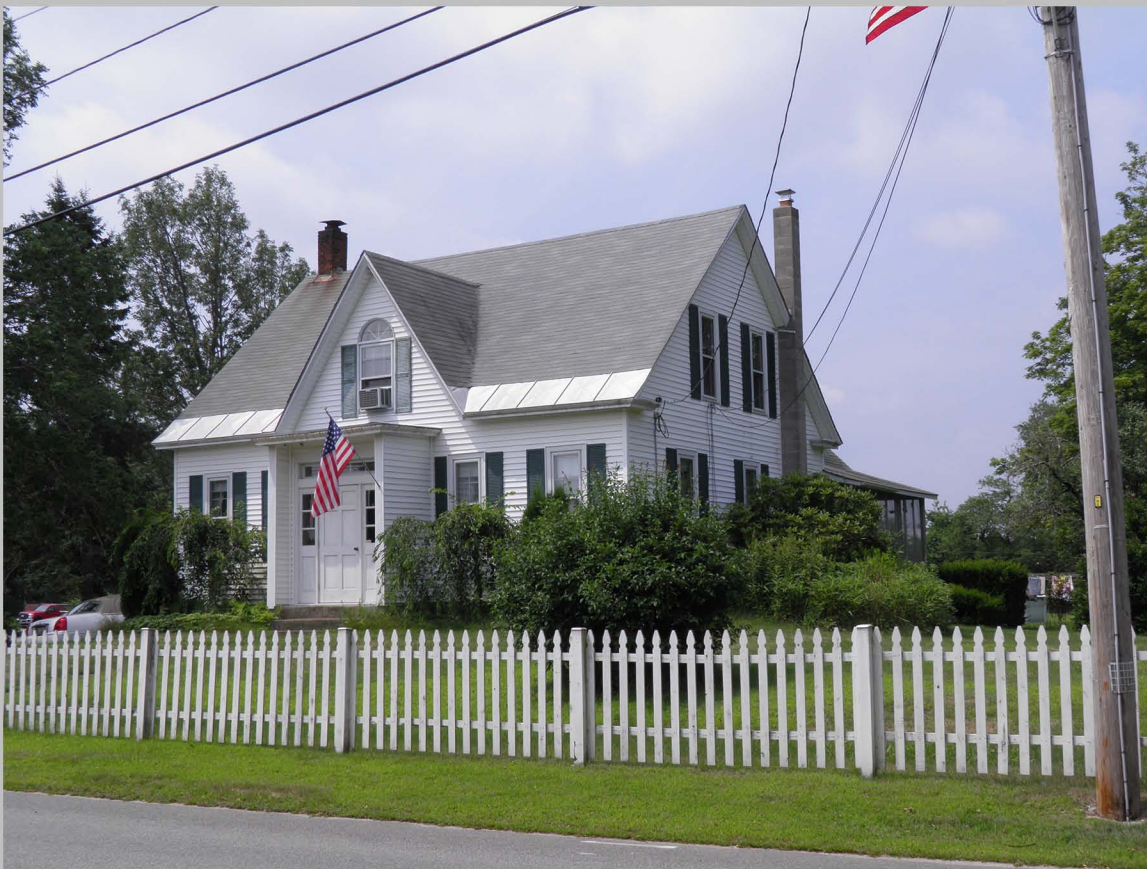
9. Colby-Townley House, 7 North Main Street, looking southwest, showing the east façade and northern elevation.
