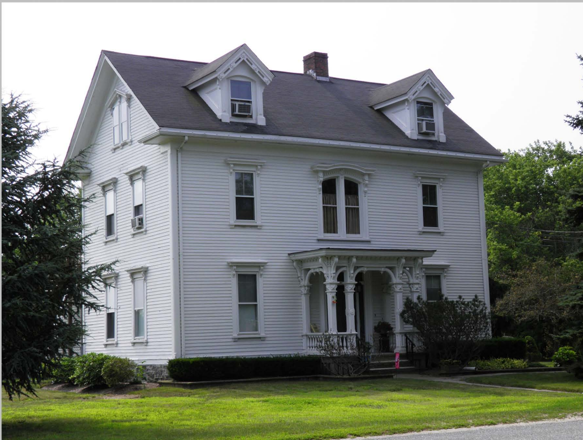
4. Porter-Pitts House, 9 Porter Street, looking east, showing west façade and north elevation.
