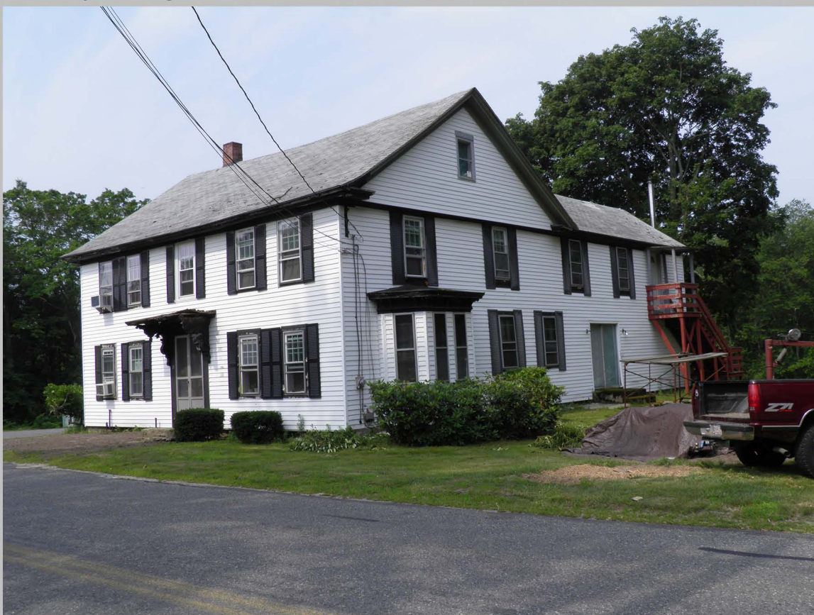
12. Hathaway-Leach House, 21 South Main Street, looking southwest, showing the east façade and the northern elevation.
