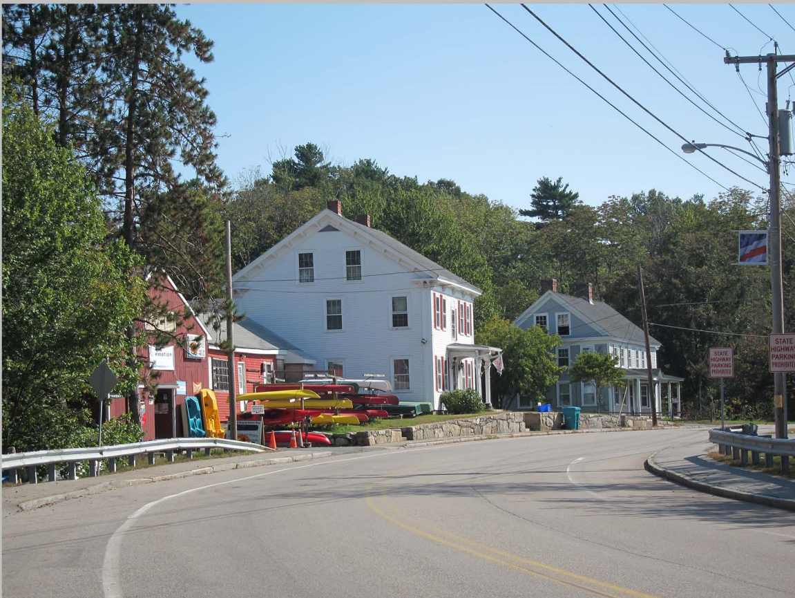
10. 10 and 12 Milford Street, looking east (Sept. 2011)
