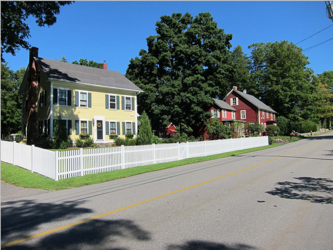
11. 20 and 22 North Main Street, looking north (Aug. 2011)
