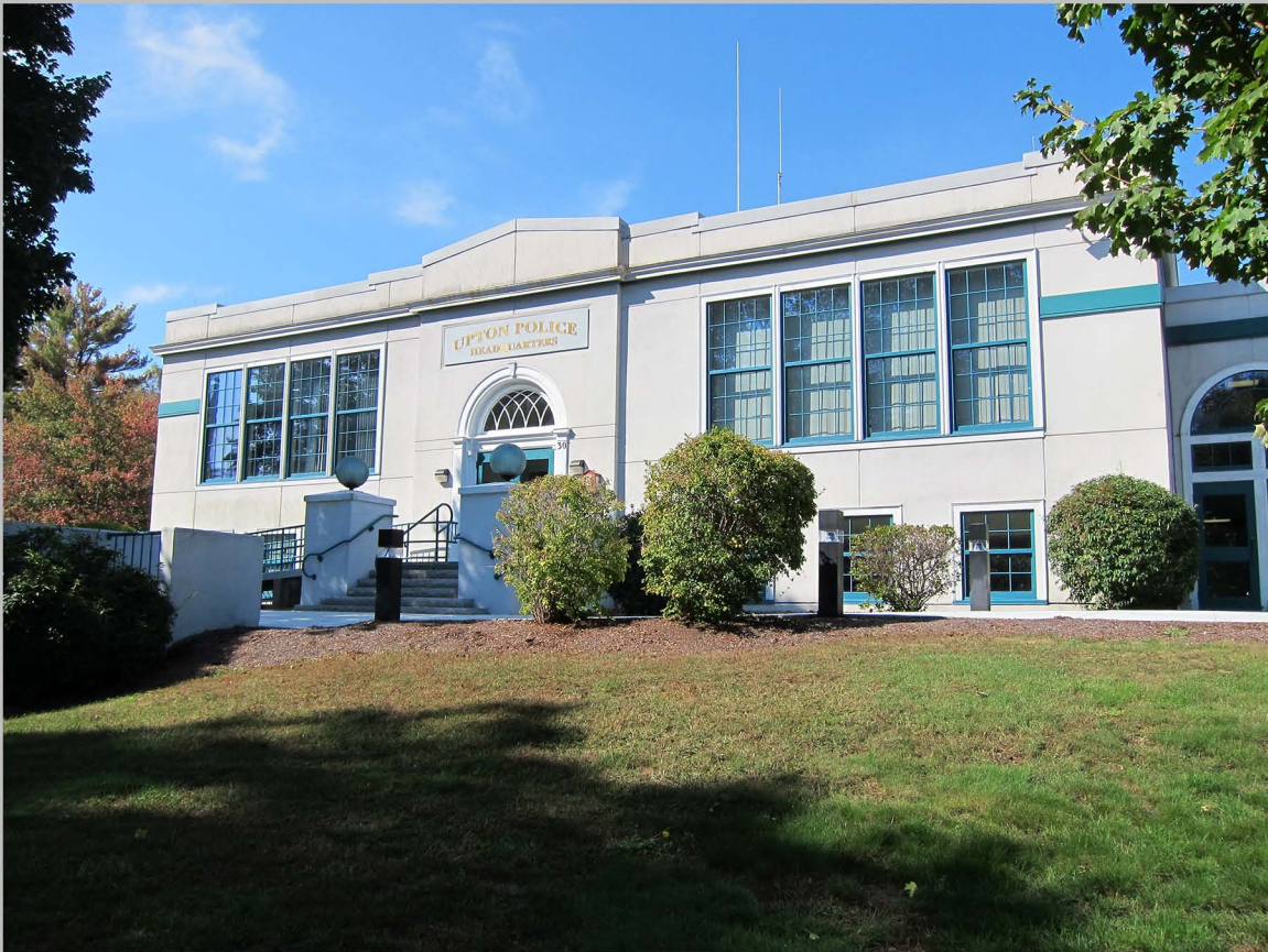
9. Ball School/Police Station, 30 School Street, looking west/southwest (Sept. 2011)
