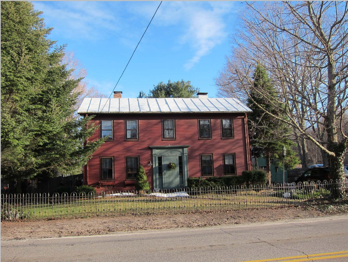
17. 10 Pleasant Street, looking south (Mar. 2011)
