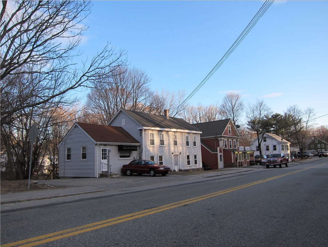
13. 8, 10, 12 Main Street, looking south/southwest (Mar. 2011)
