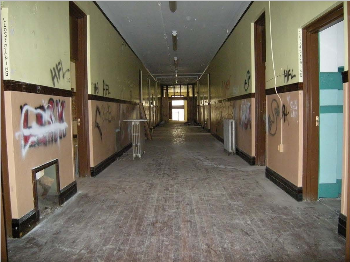
20. View north, second-floor corridor
