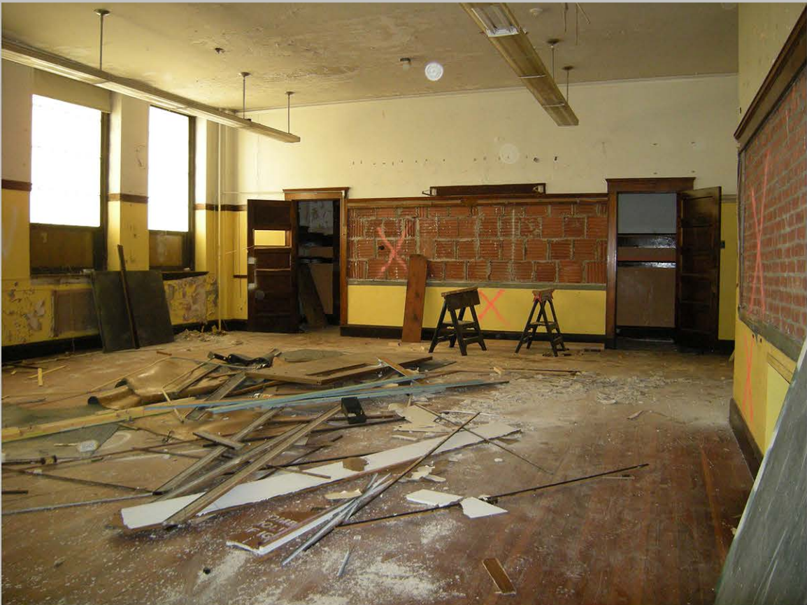
18. View southeast first-floor classroom, typical
