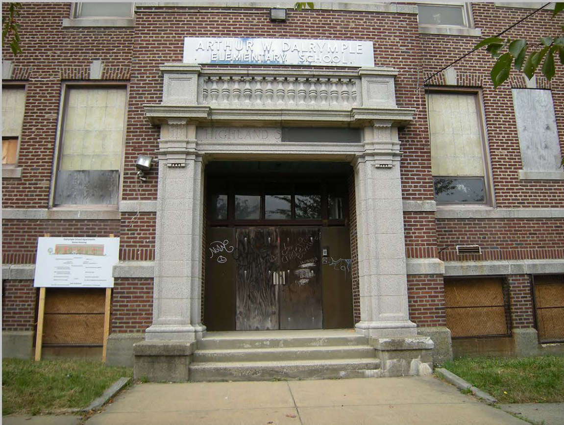
5. East elevation, main entrance, "Highland S" visible at the frieze
