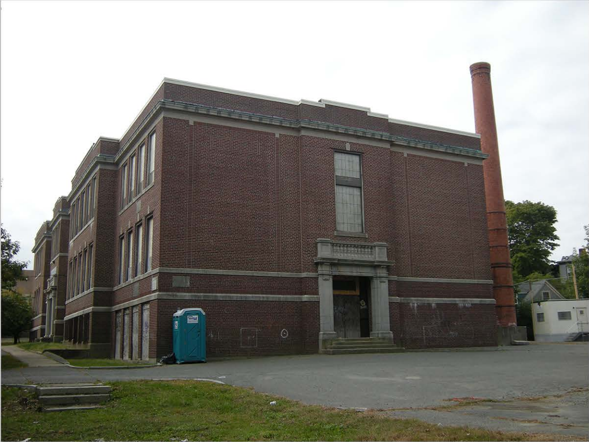
7. North elevation, north addition (1929)
