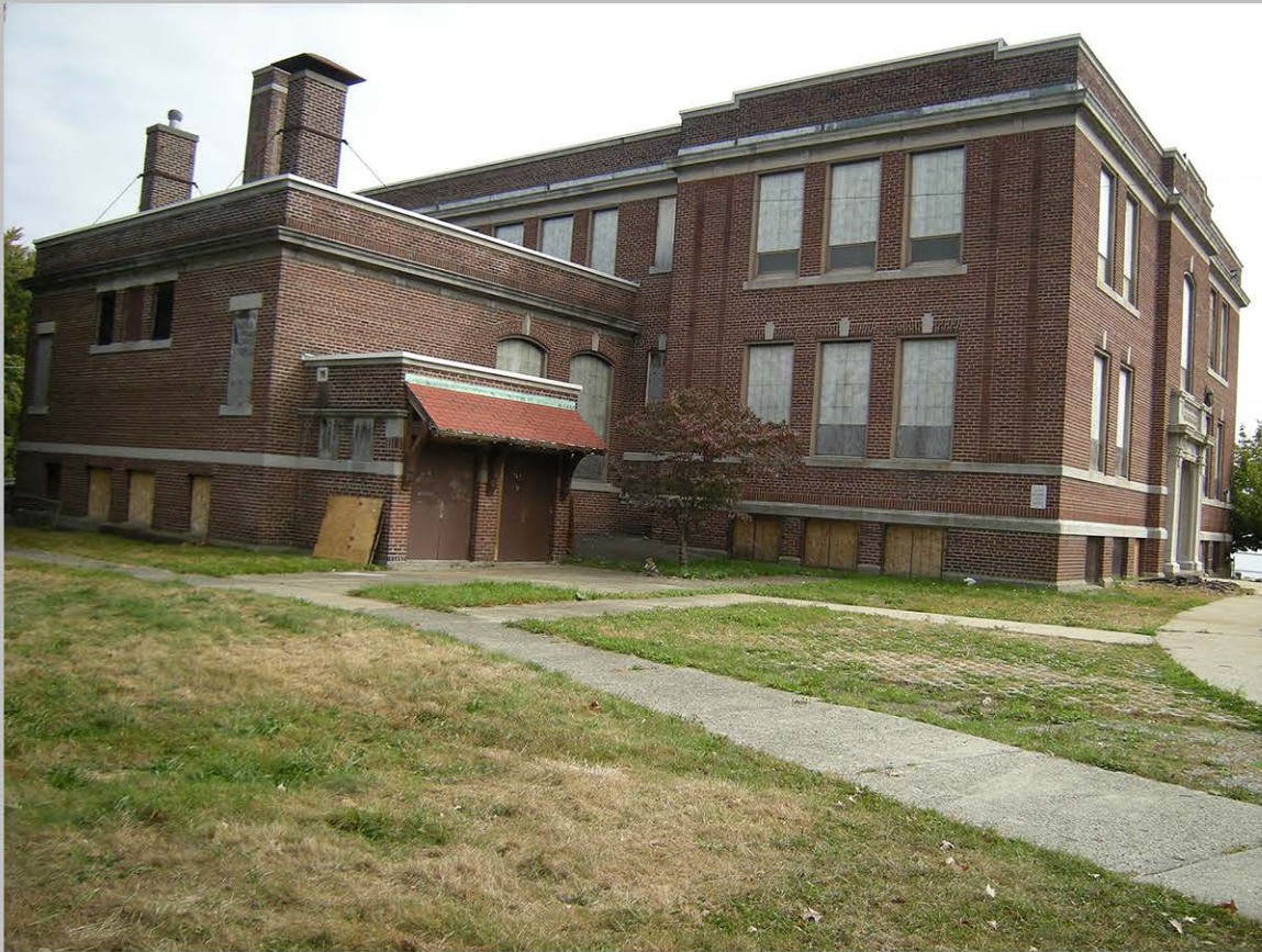
11. West and south elevations auditorium
