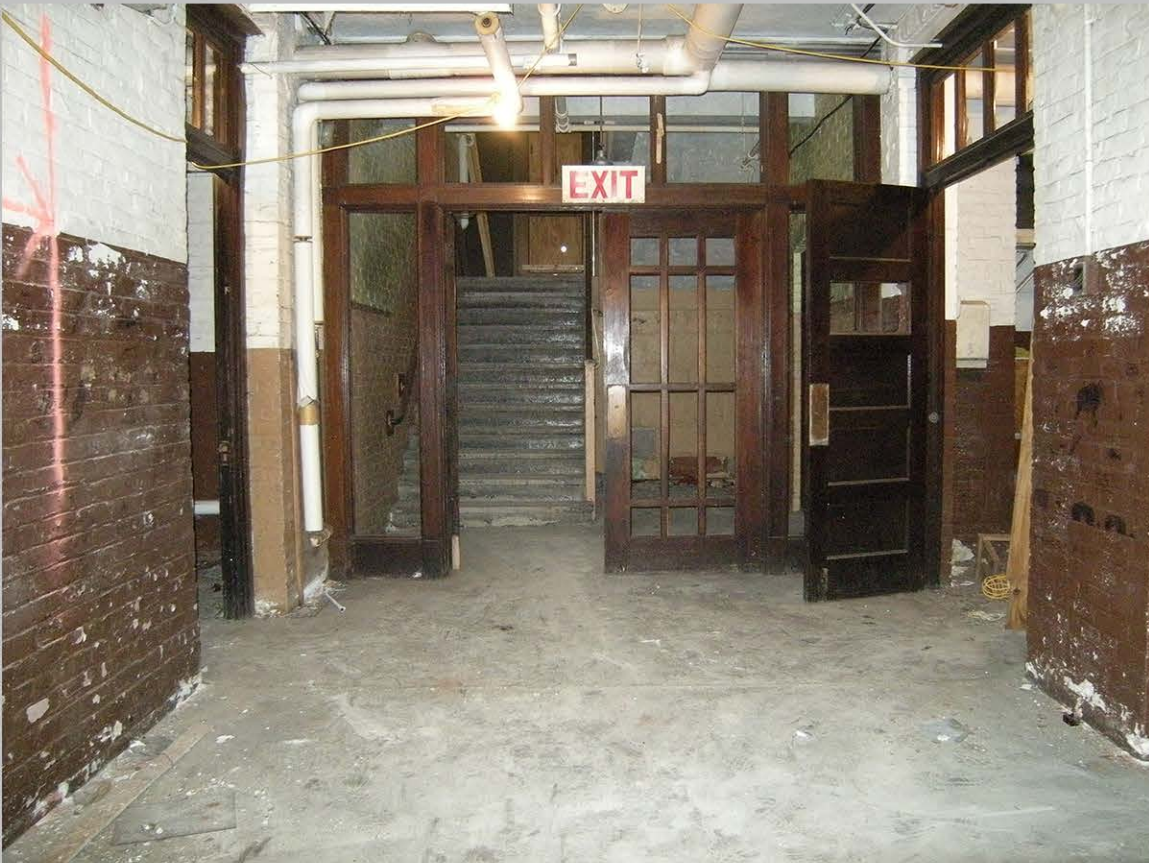
24. View south at basement showing fire partition and transoms
