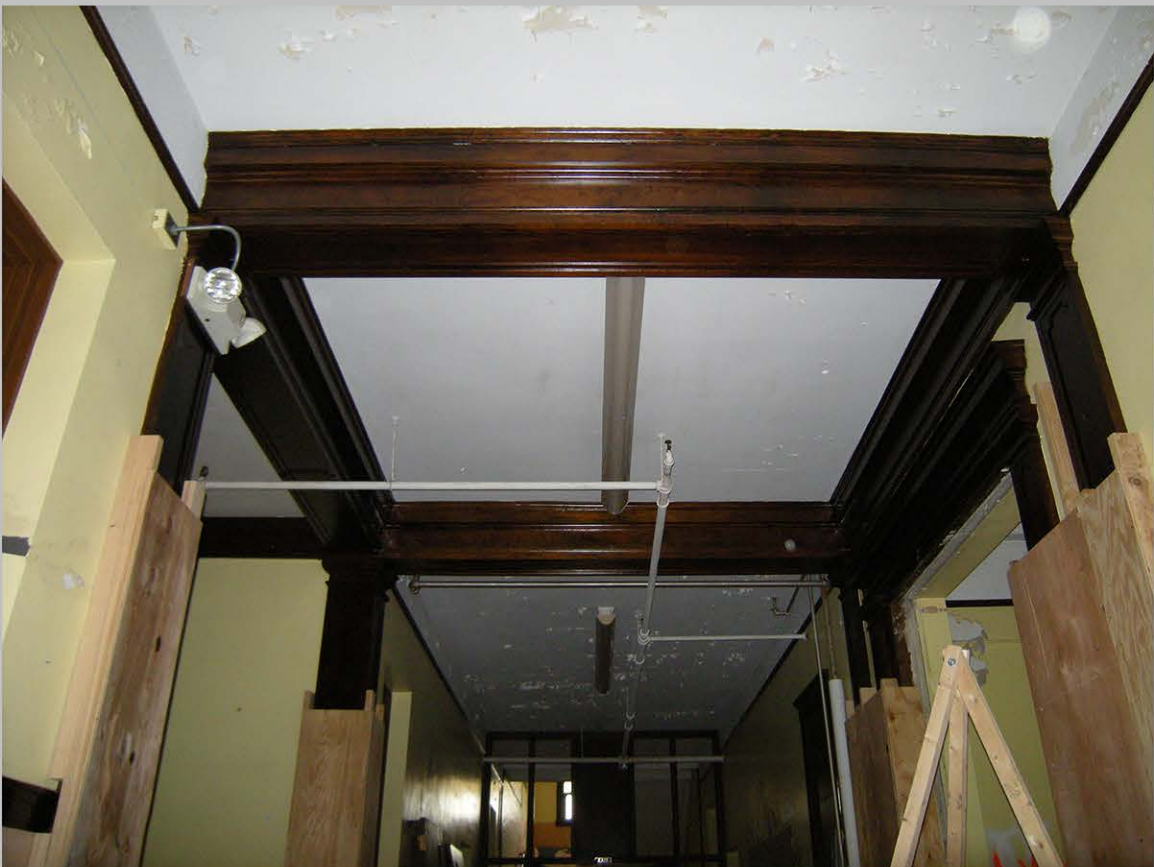
16. Paneled wood beams, pilasters and cornice at entrance, first-floor corridor
