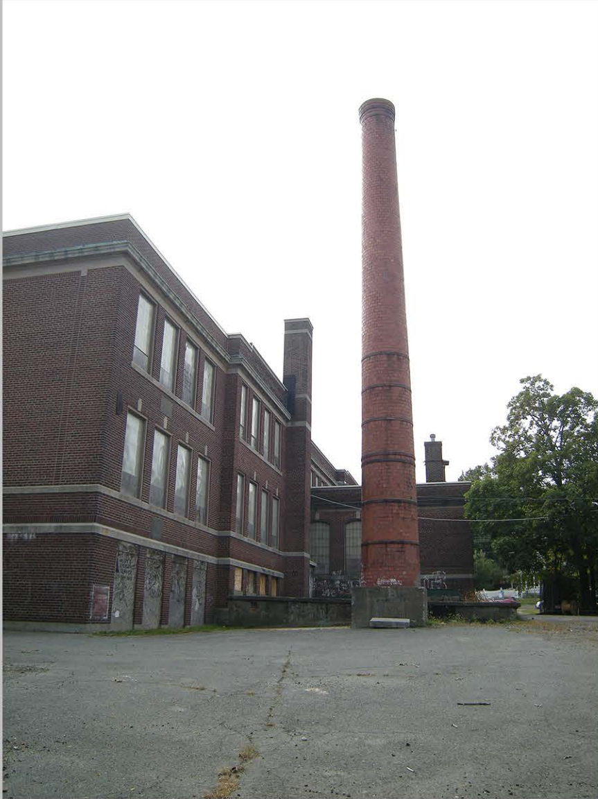
9. North elevation, round chimney, boiler room behind chimney at grade
