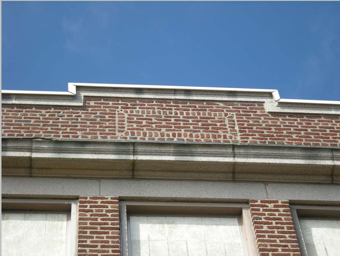
13. Brick panel detail in parapet above main entrance, typical
