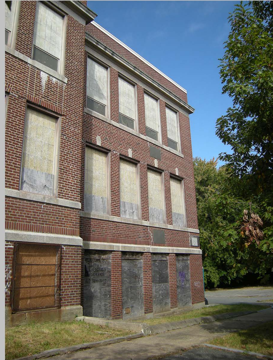
4. East elevation, north addition (1929)
