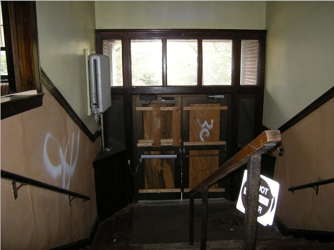
15. Interior view east at main entrance with original transom
