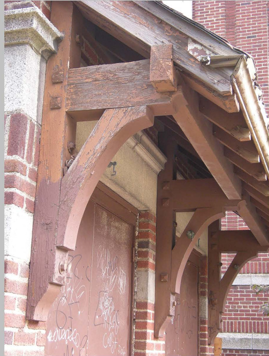
12. Detail, Arts & Crafts-style brackets supporting pent-roofed canopy at auditorium entrance
