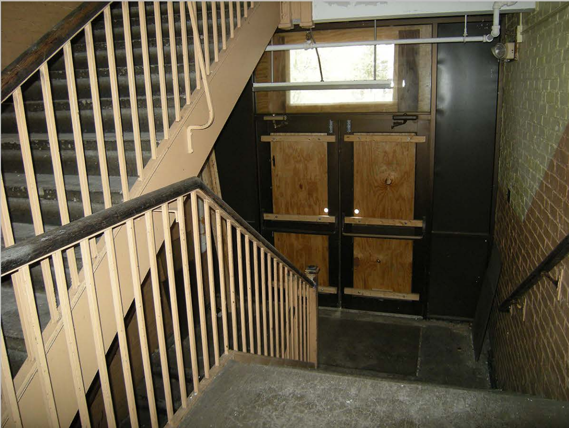
23. View south toward landing, south stair first floor to basement
