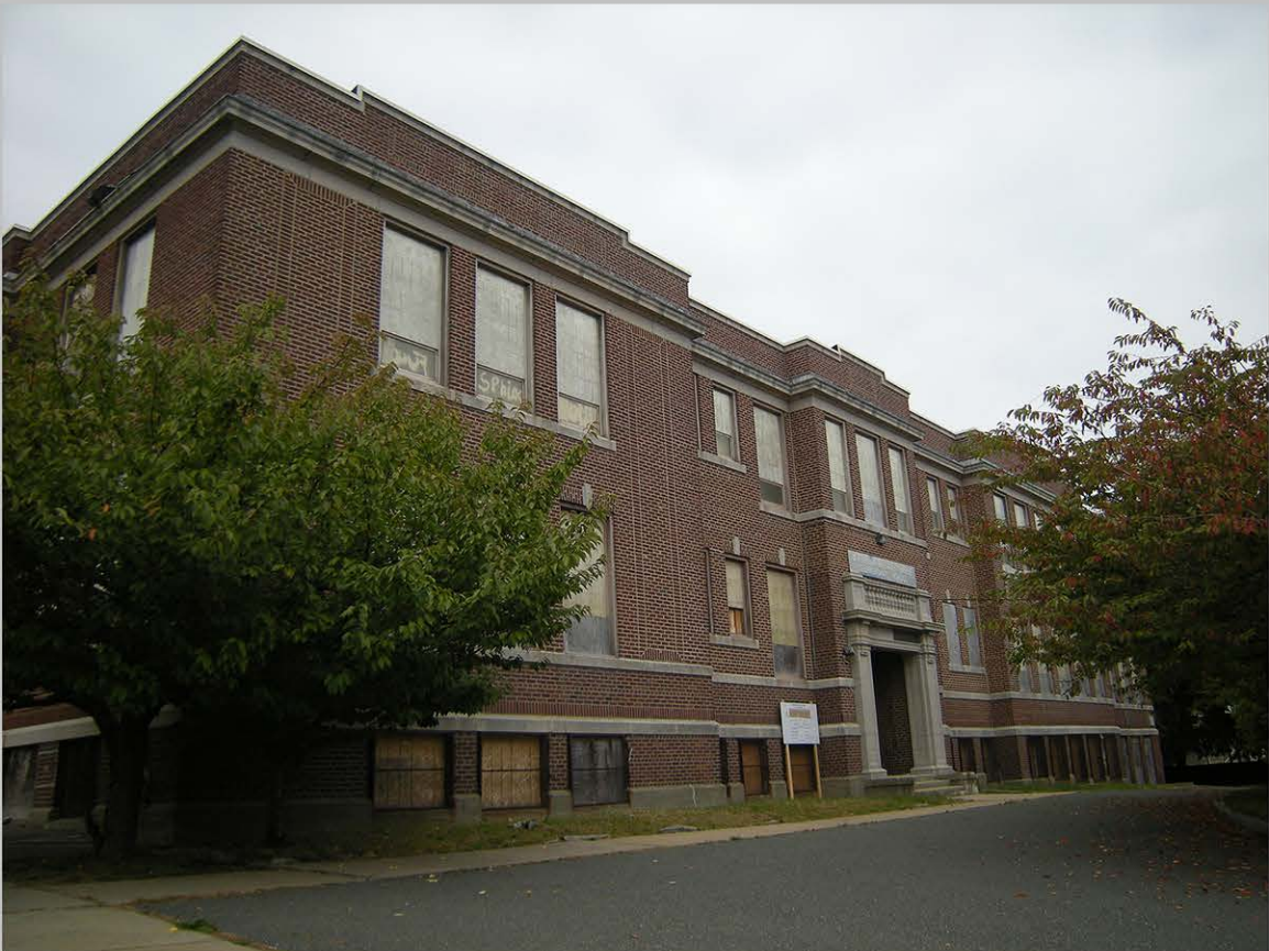
2. East elevation, main building. Brick pattern work visible
