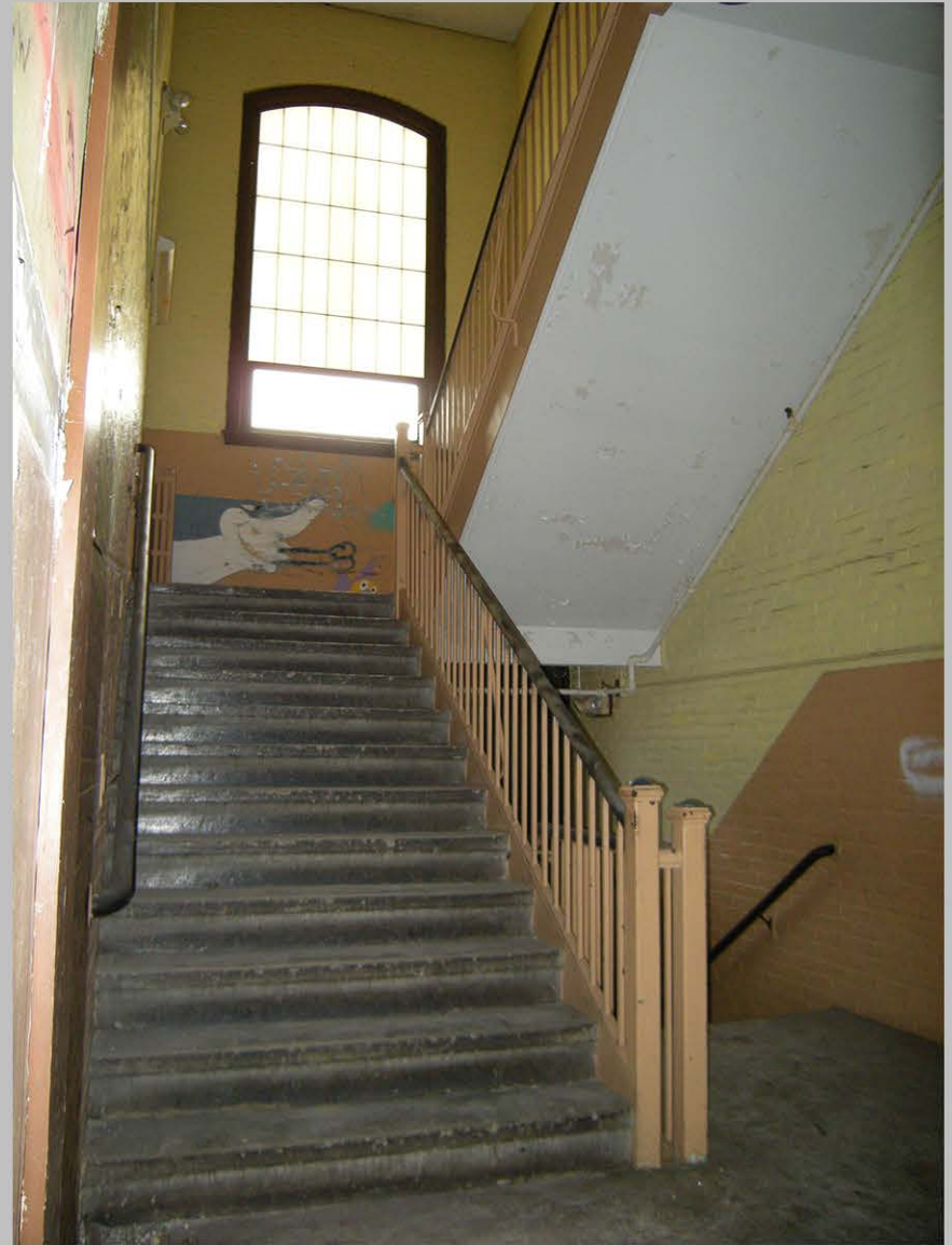
22. View south at south stair, first to second floor
