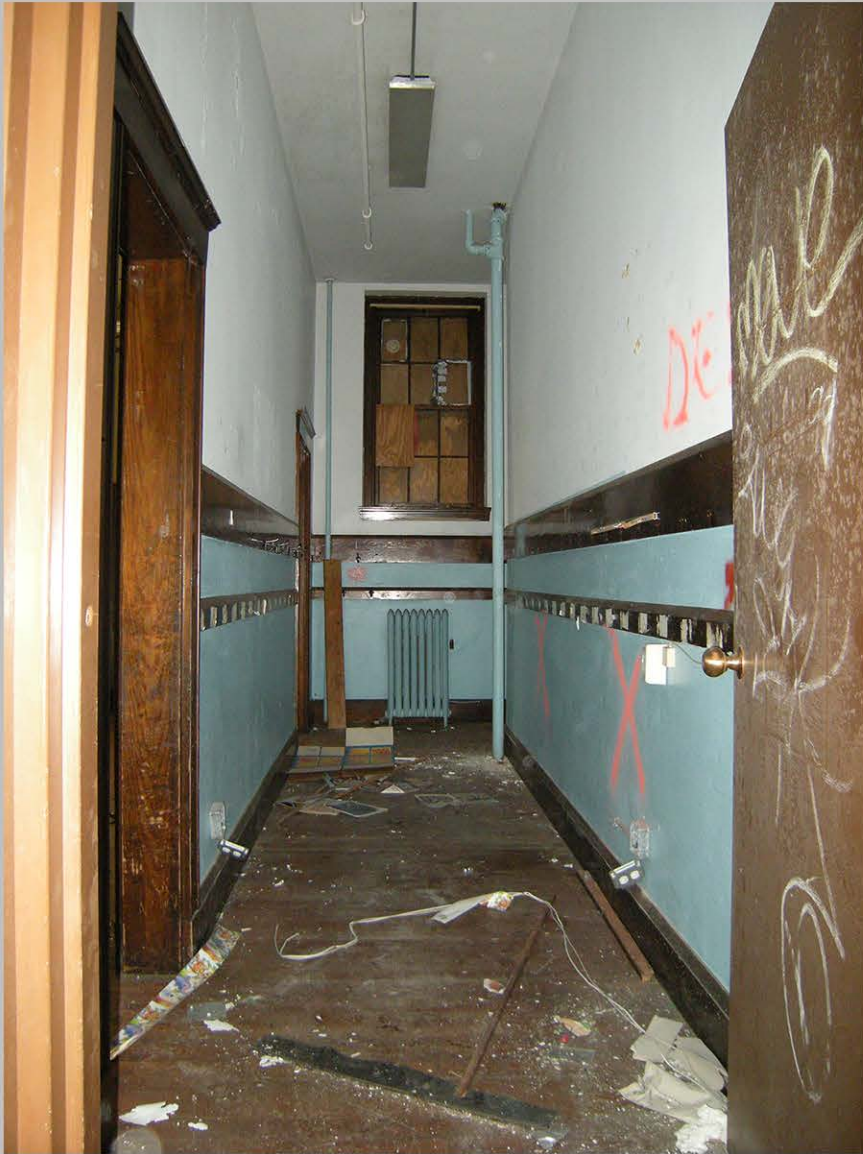
21. View west, second-floor coat room, typical
