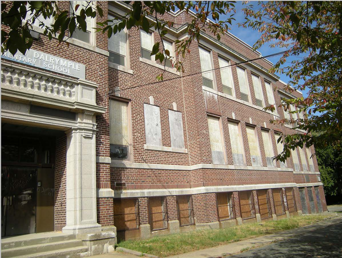
3. East elevation, main building, north end, view of bay added later
