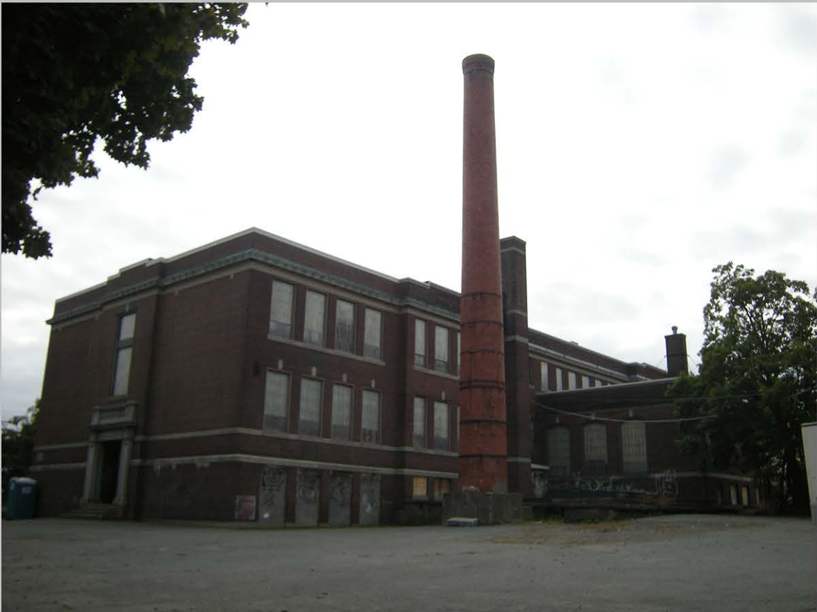
8. North and west elevations, north addition to the left, round chimney at the center
