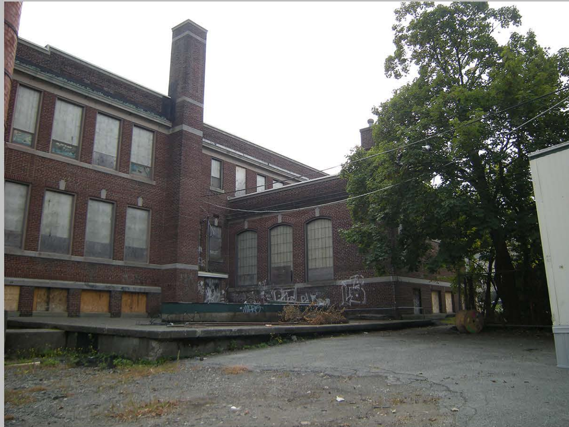
10. West elevation main building and north elevation auditorium. Paneled brick chimney with beltcourses at center
