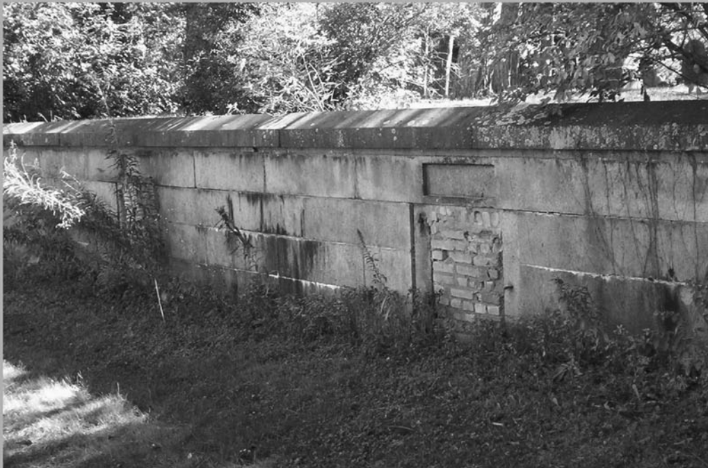
3. Tombs in western wall, view to NE (Photographer: Philip Bergen, September 2007)
