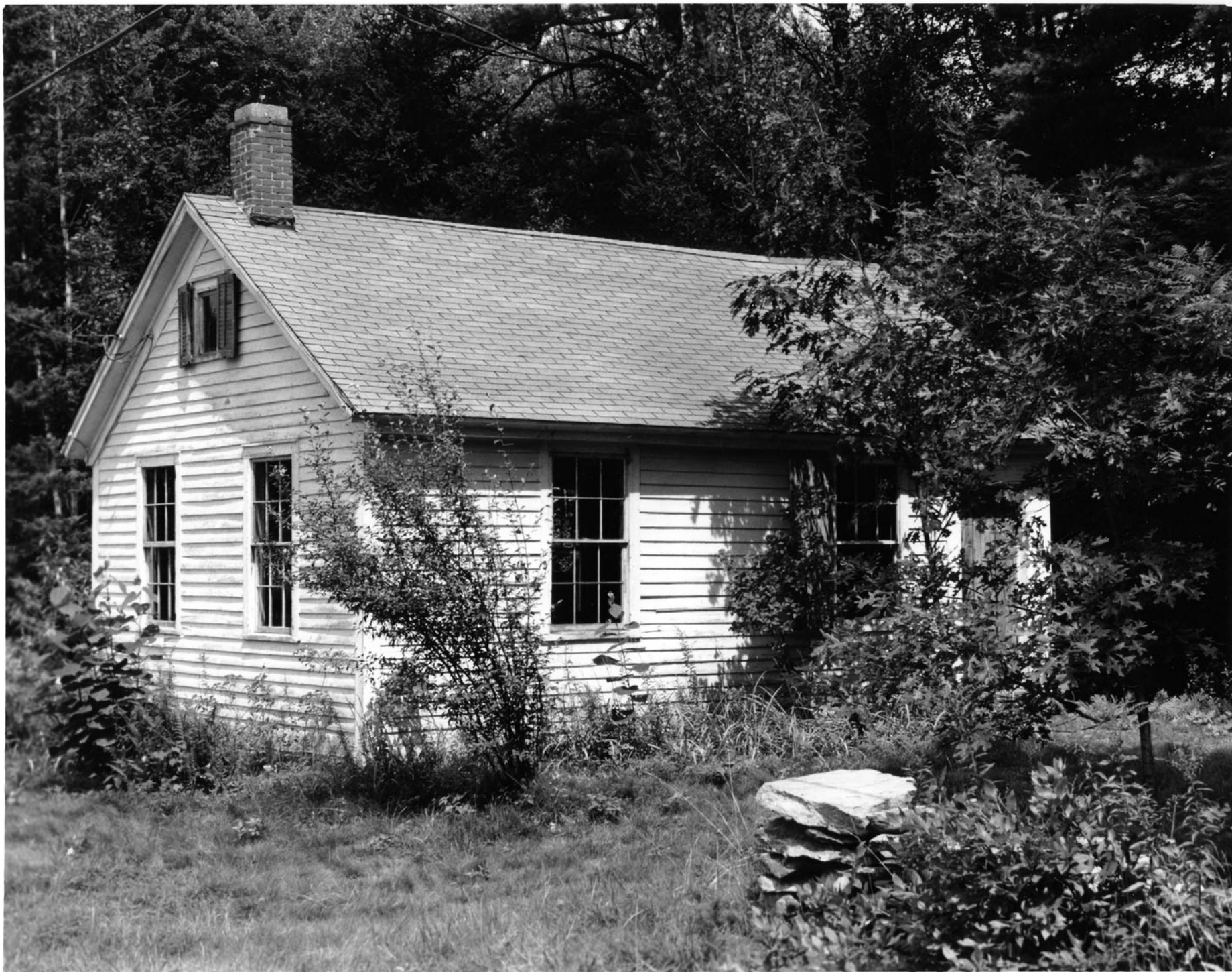
1. South School, Façade (south) and west elevation (Photographer: John Shershin, August 2004)
