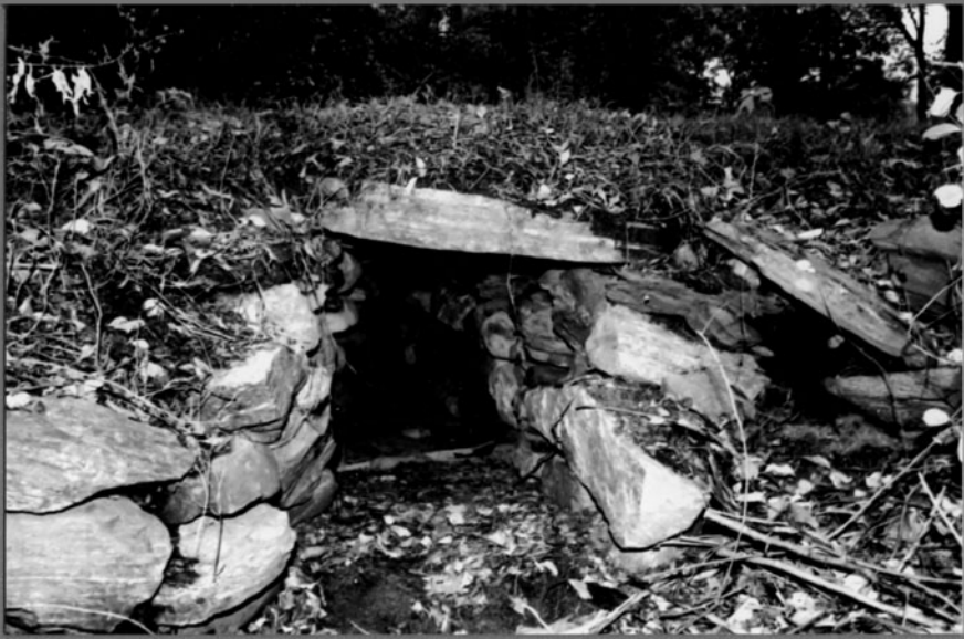
16. 604 Hill Road. Silas Wetherbee Farm: cow pass under farm lane, looking north
