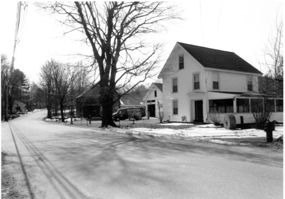
10. 828 Hill Road, Reuben Mead Draper House, ca. 1851: looking south
