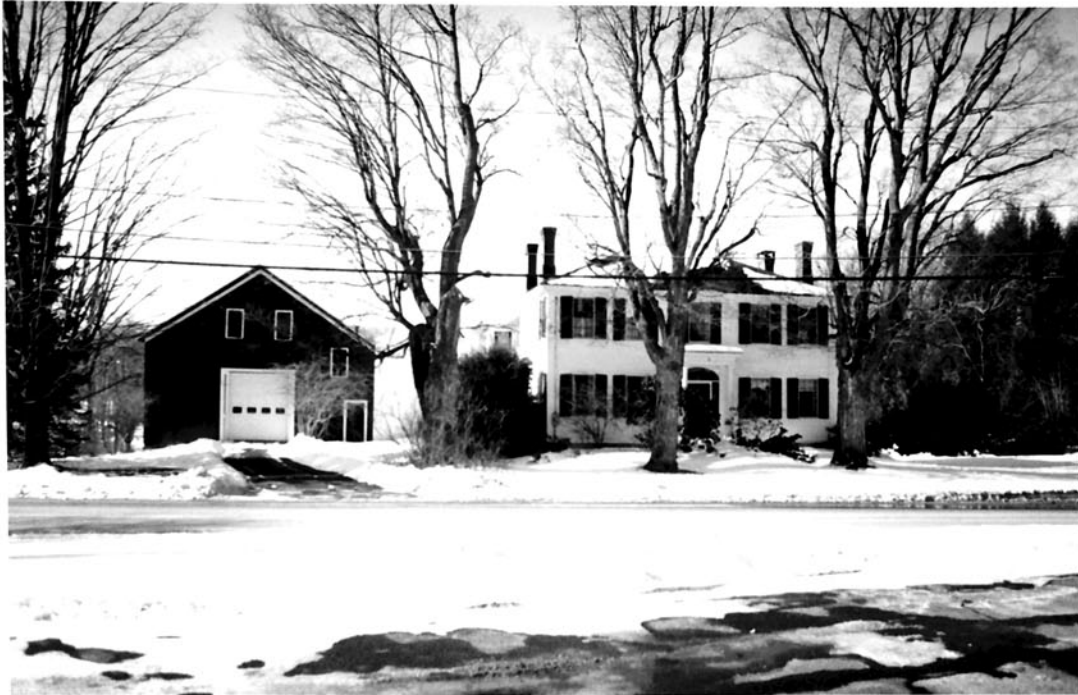
5. Bliss-Brown House, 9 Warren Road, looking W (Photographer: Bonnie Parsons, February 2004)
