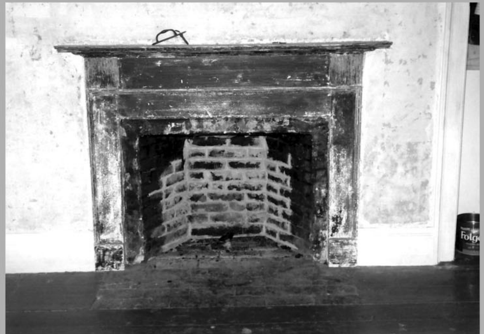
20. Interior, second floor, east room, west view
