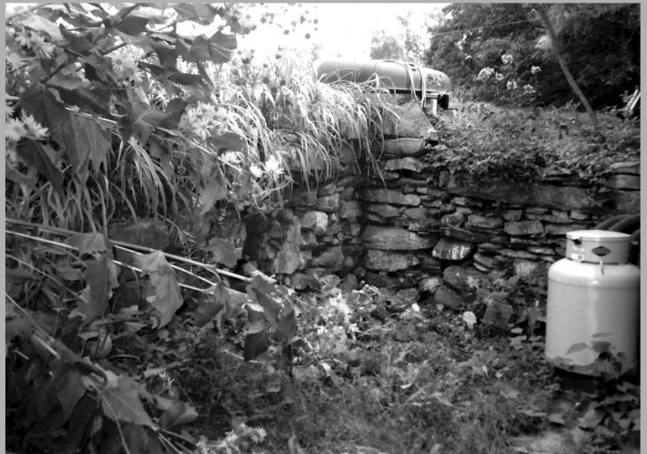
23. L-shaped stone wall, north side, east view
