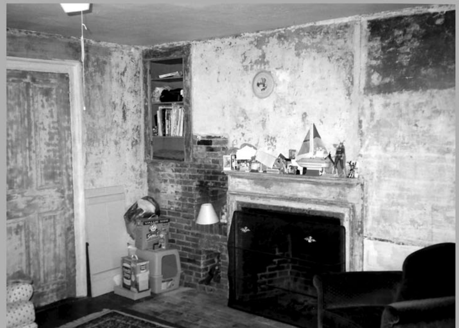
12. Interior, first floor, west room, northeast view
