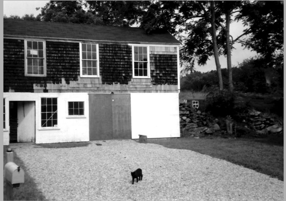
6. East addition, south elevation, north view
