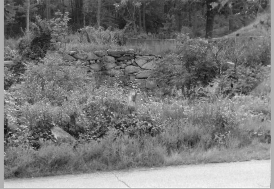
2. Barn foundation, south side, Martins Pond Road, south view
