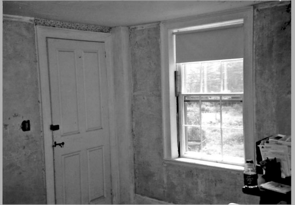
19. Interior, second floor, west room, southeast view
