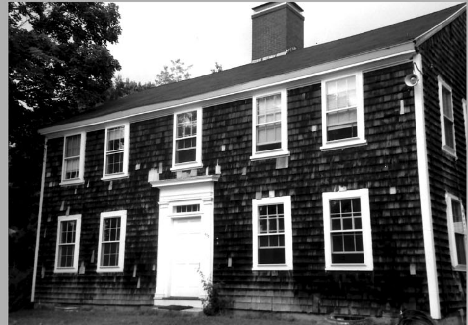
4. South elevation, north view
