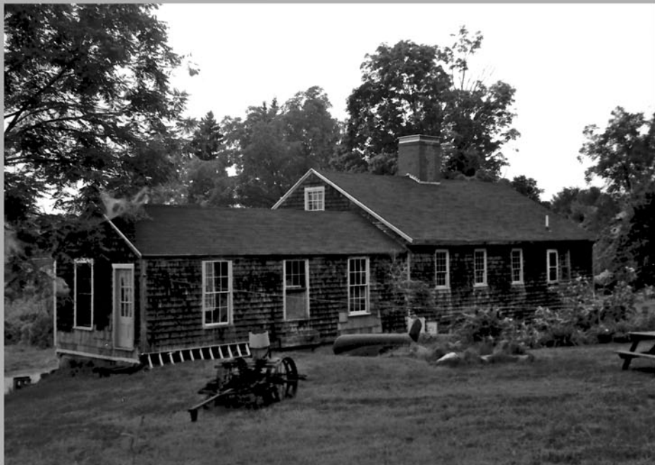
8. North elevation, south view
