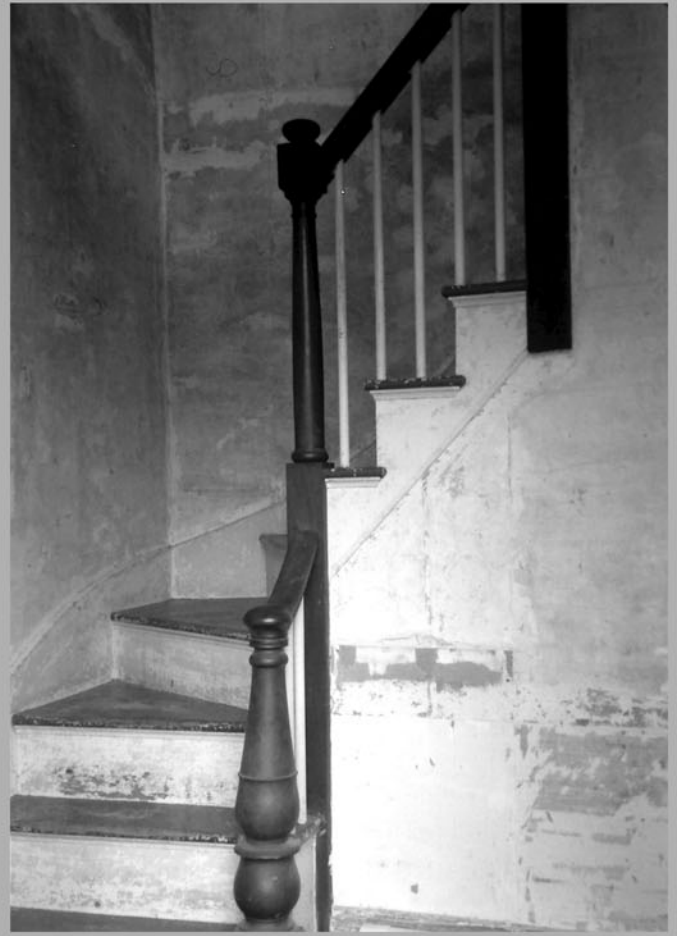
13. Interior, first floor, front hall, north view
