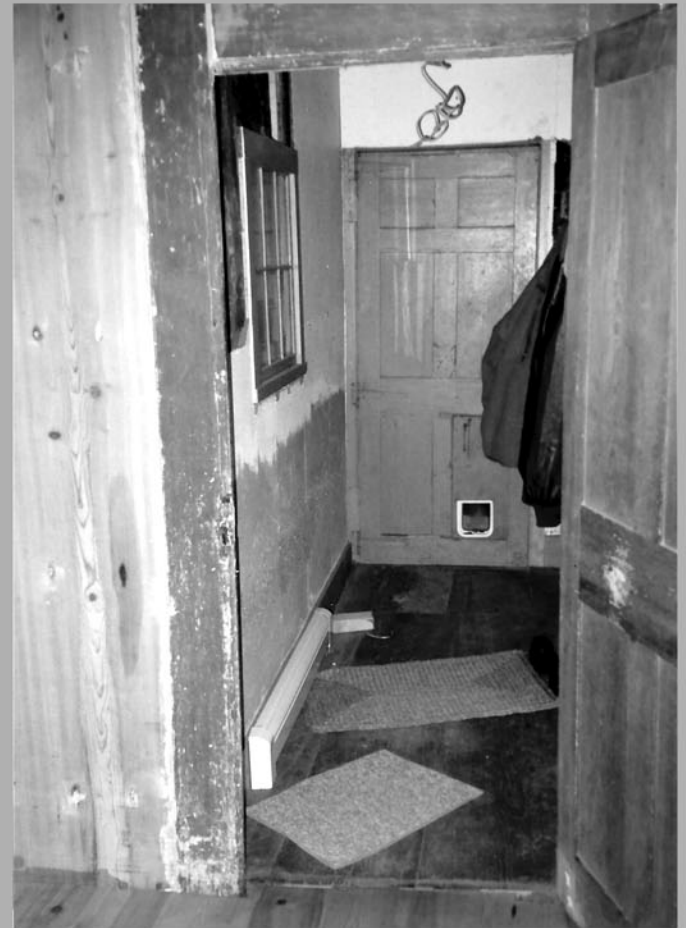
17. Interior, second floor, east room, northwest view
