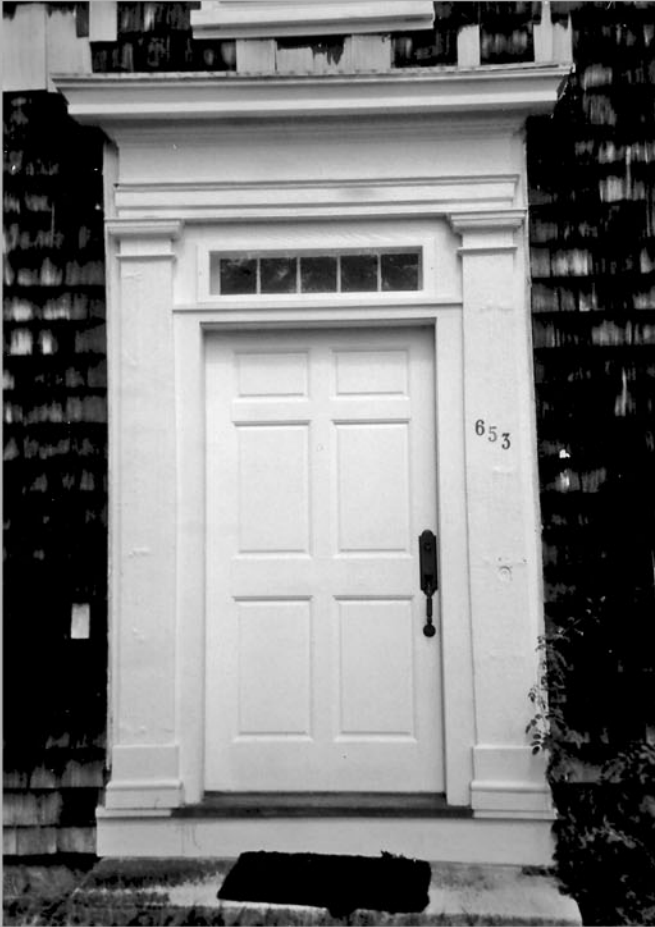
5. South elevation, front door, north view
