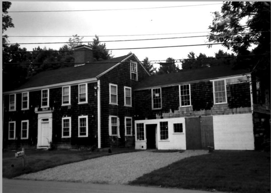
3. South elevation, north view
