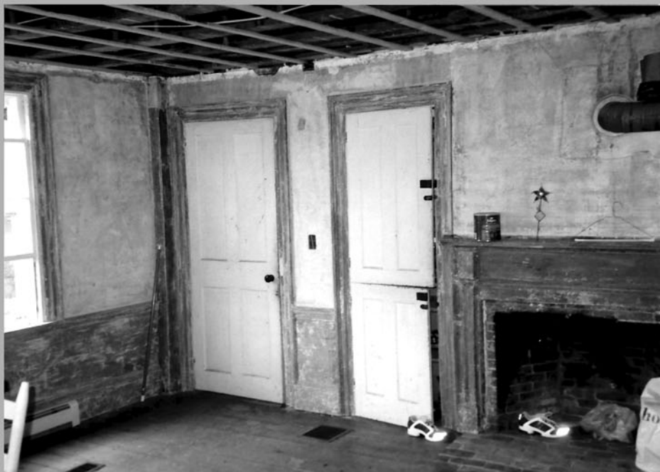
10. Interior, first floor, west room, northeast view
