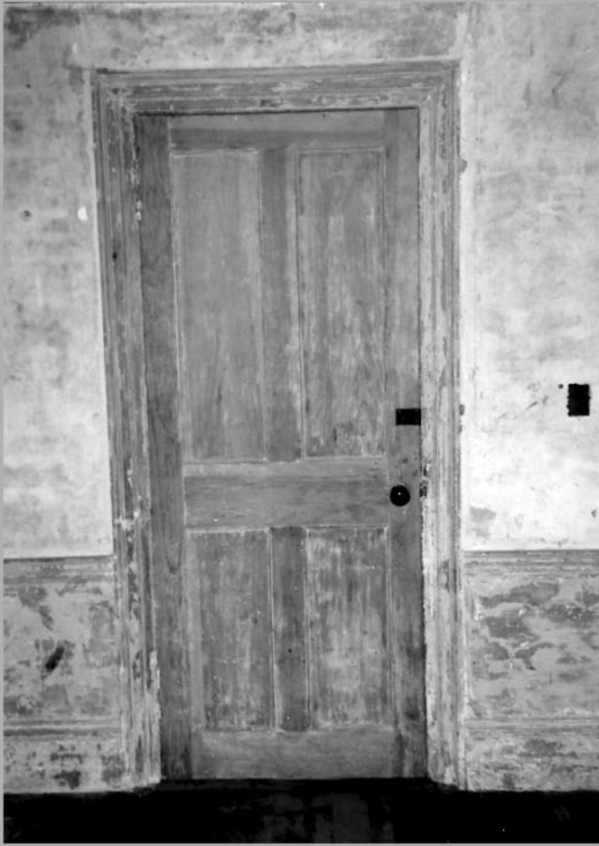
11. Interior, first floor, east room, north view
