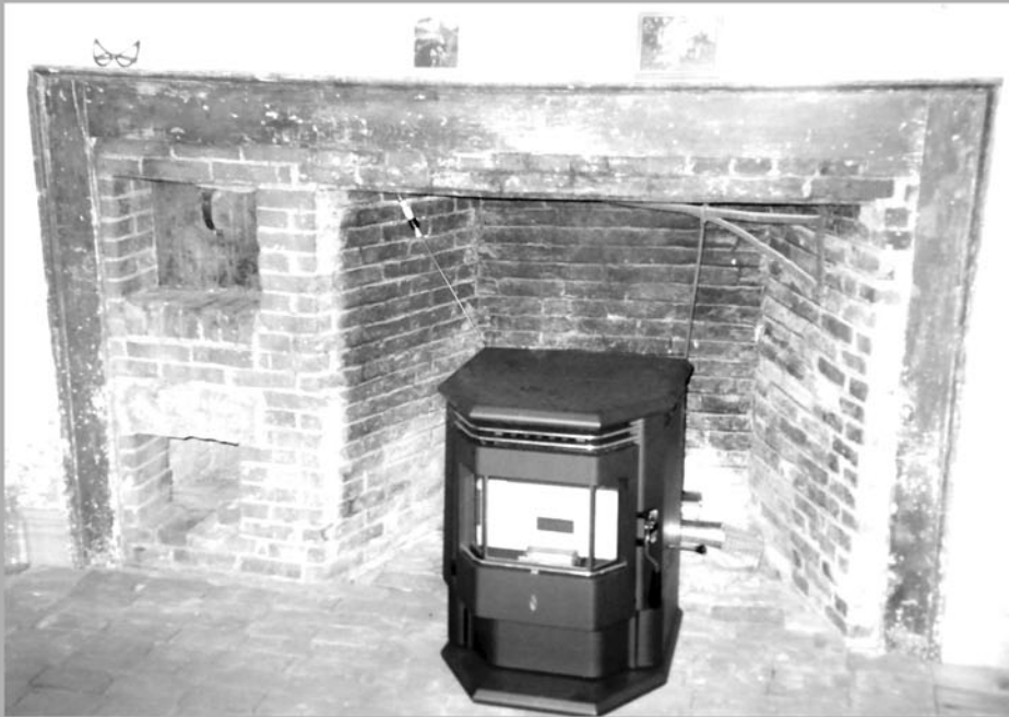
15. Interior, first floor, north room, fireplace
