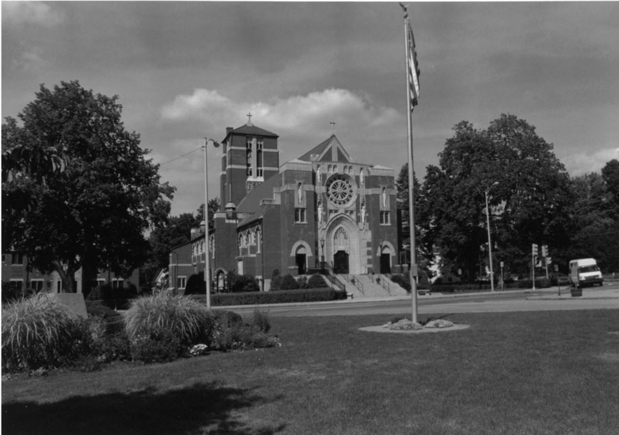
4. St. Mary's Church, 1 Church Square, south (facade) and west elevations (Photographer: Karen L. Davis, Fall 2002)
