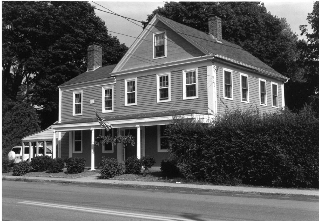
7. 287 Main Street, G.W. Morse House, west (facade) and south elevations (Photographer: Karen L. Davis, Fall 2002)
