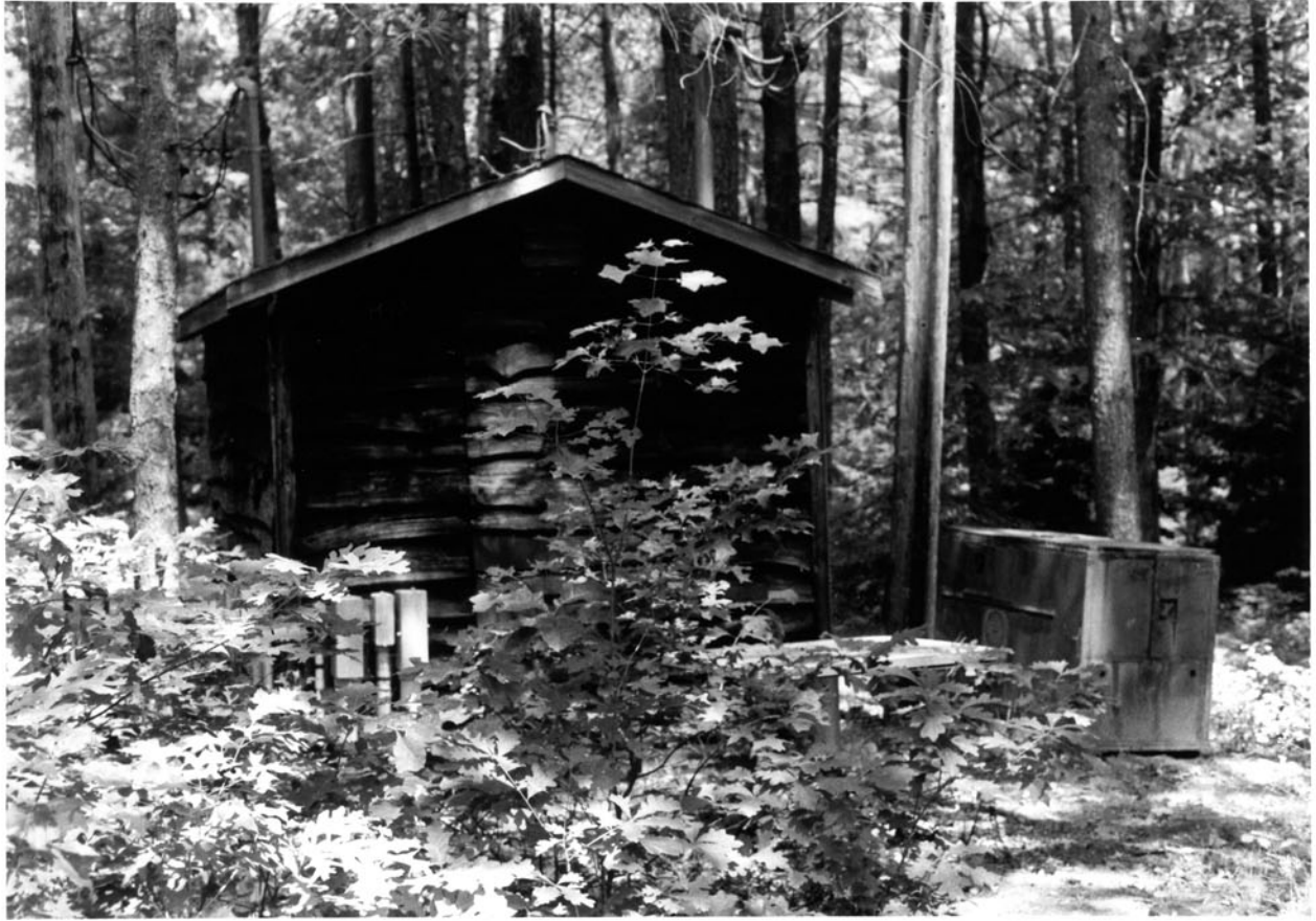
17. Electric Shop. Showing south façades, looking north. (Photographer: Timothy Orwig, July 2002)
