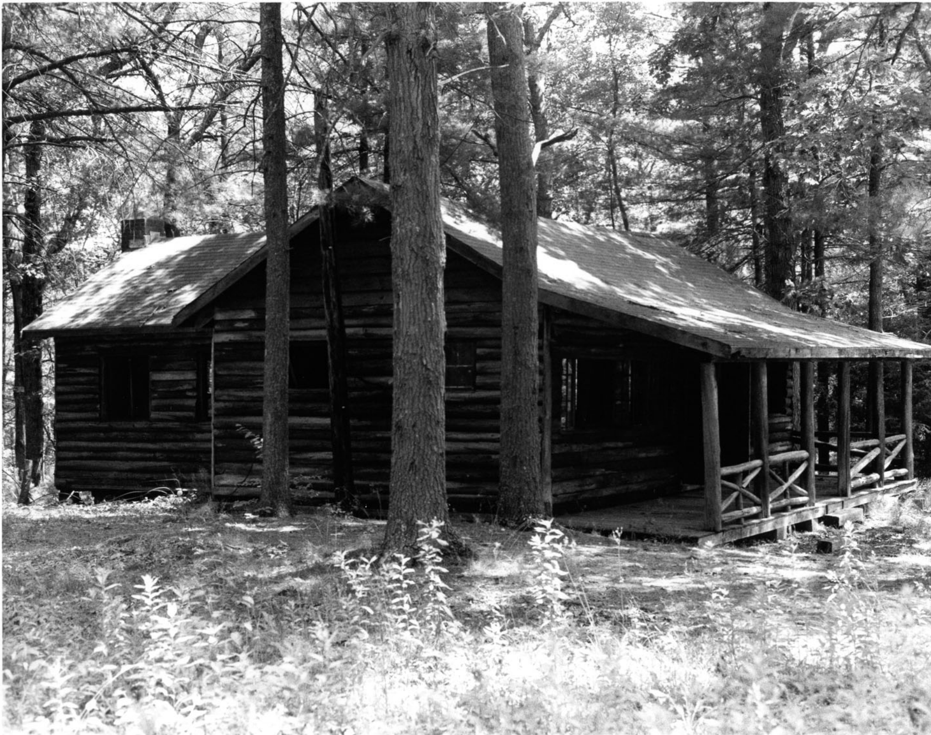
3. Gypsy Cabin. Showing north and west façades, looking southeast. (Photographer: Timothy Orwig, July 2002)
