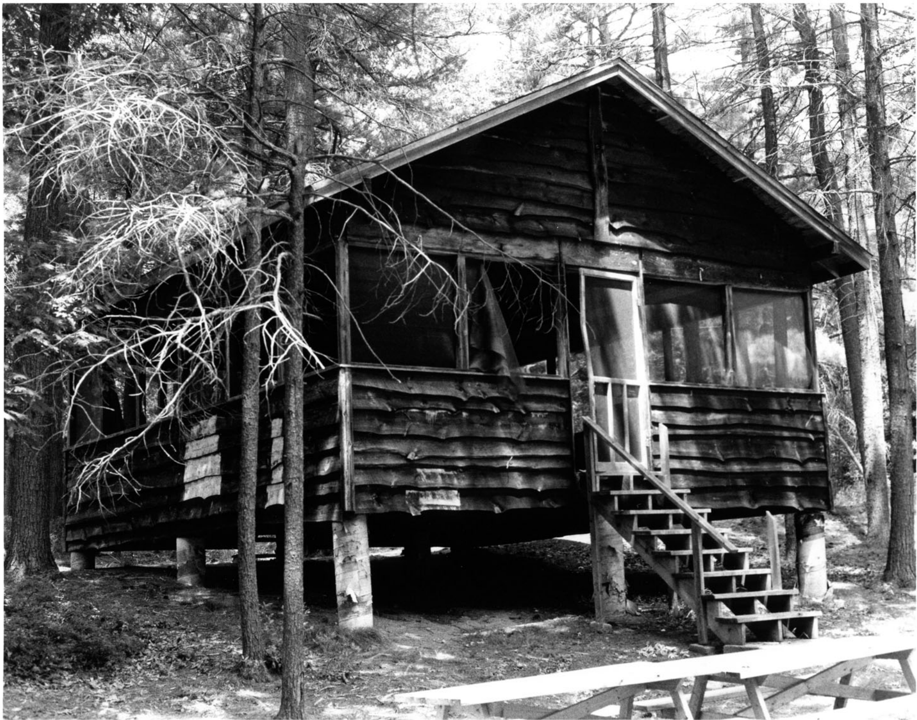
4. North Chalet. Showing south and west façades, looking northeast. (Photographer: Timothy Orwig, July 2002)
