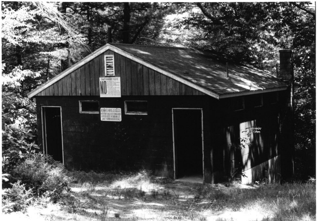
16. North Circle Bathhouse. Showing south and west façades, looking north. (Photographer: Timothy Orwig, July 2002)
