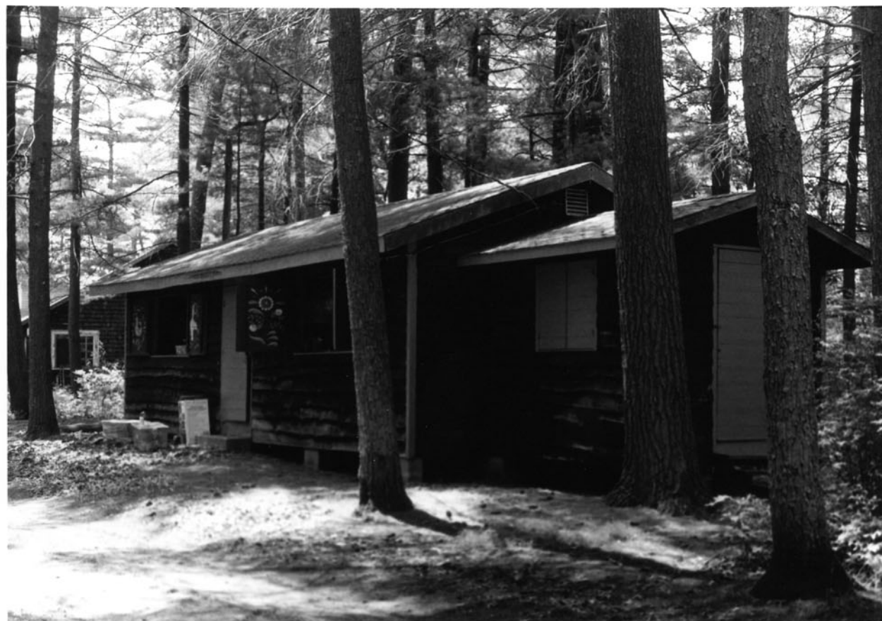
14. Craft Cabin. Showing north and east façades, looking southwest. (Photographer: Timothy Orwig, July 2002)
