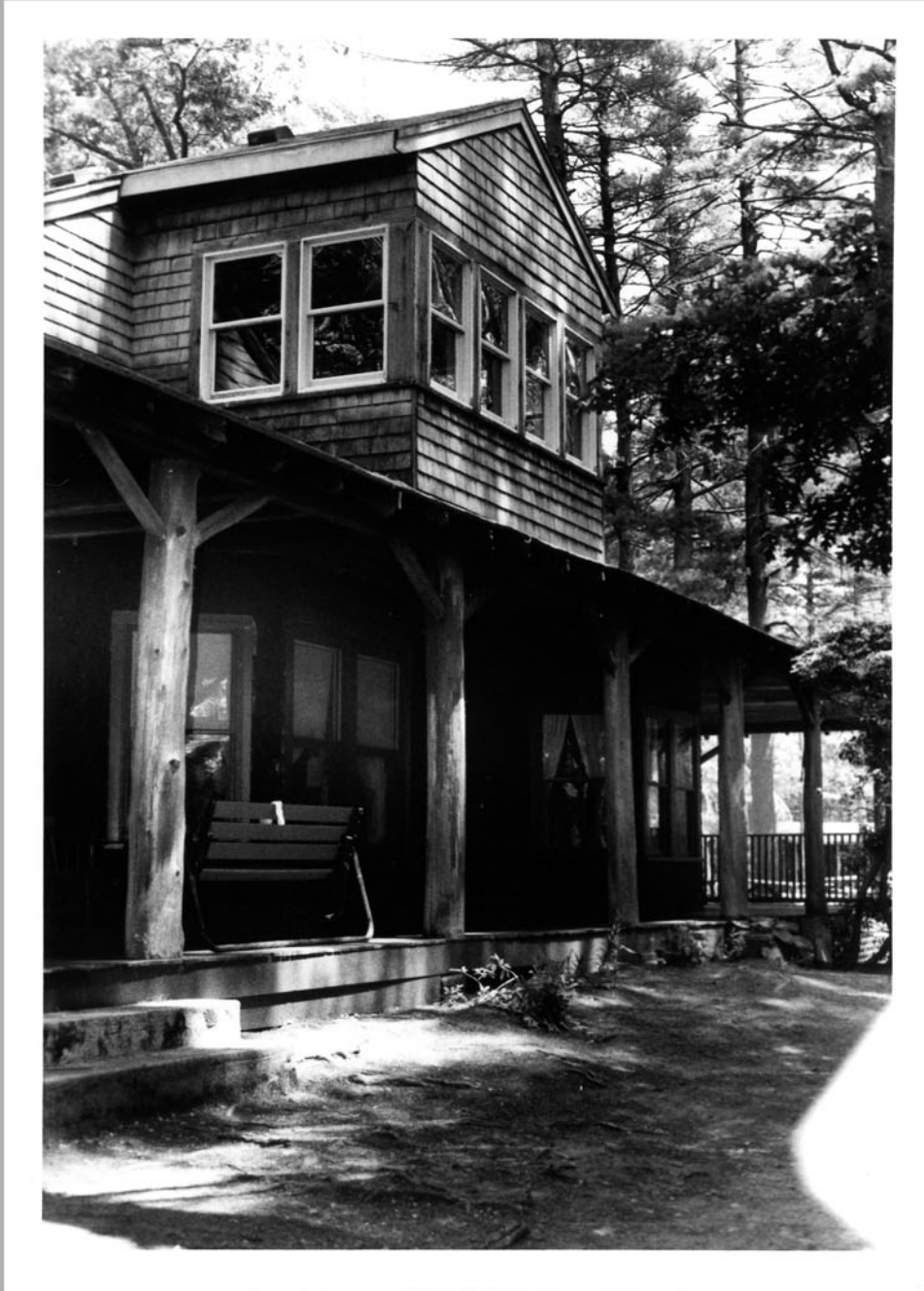
12. Main Bungalow. South façade detail, looking northeast. (Photographer: Timothy Orwig, July 2002)
