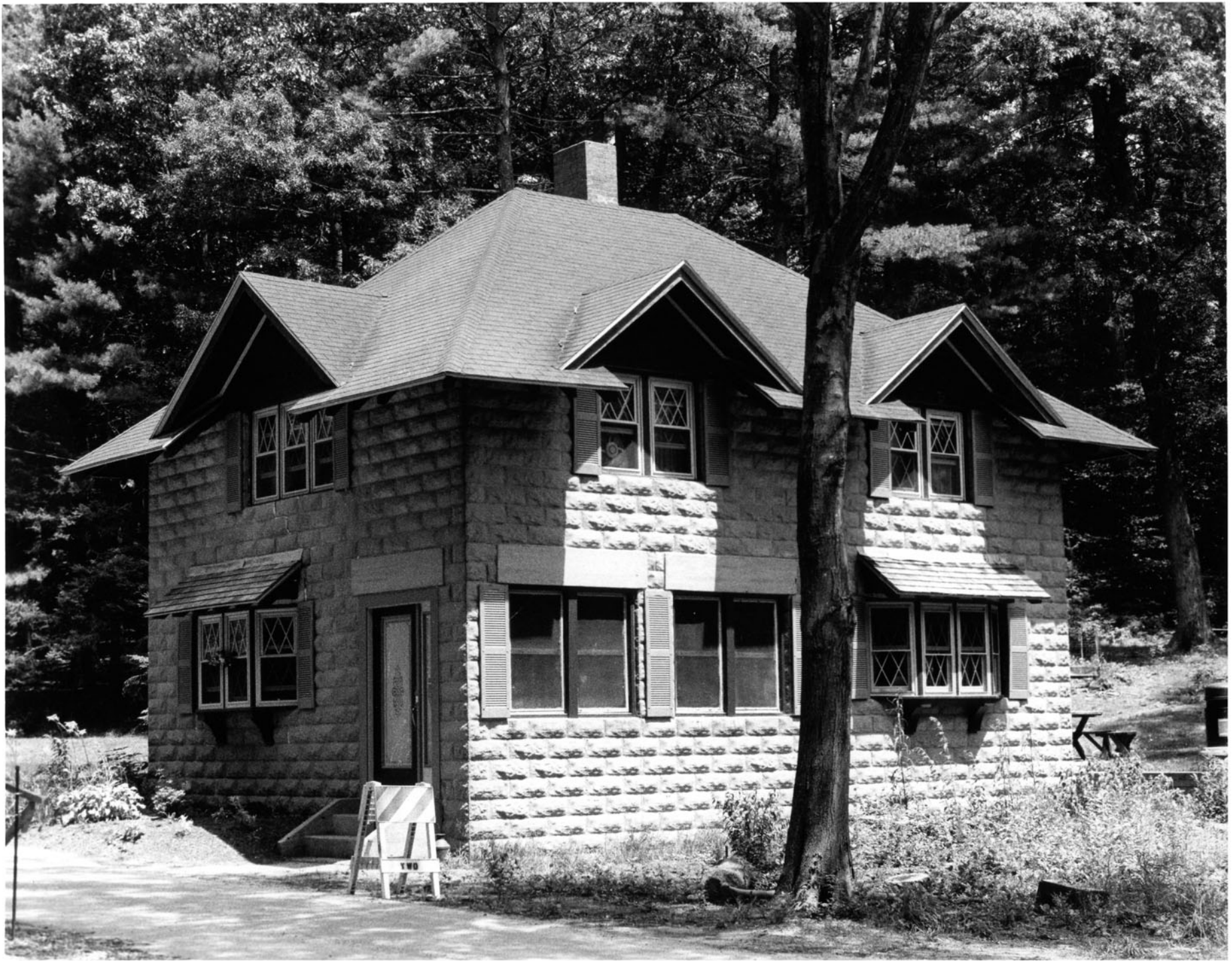
1. Gatehouse Lodge. Showing south and west façades, looking northeast. (Photographer: Timothy Orwig, July 2002)
