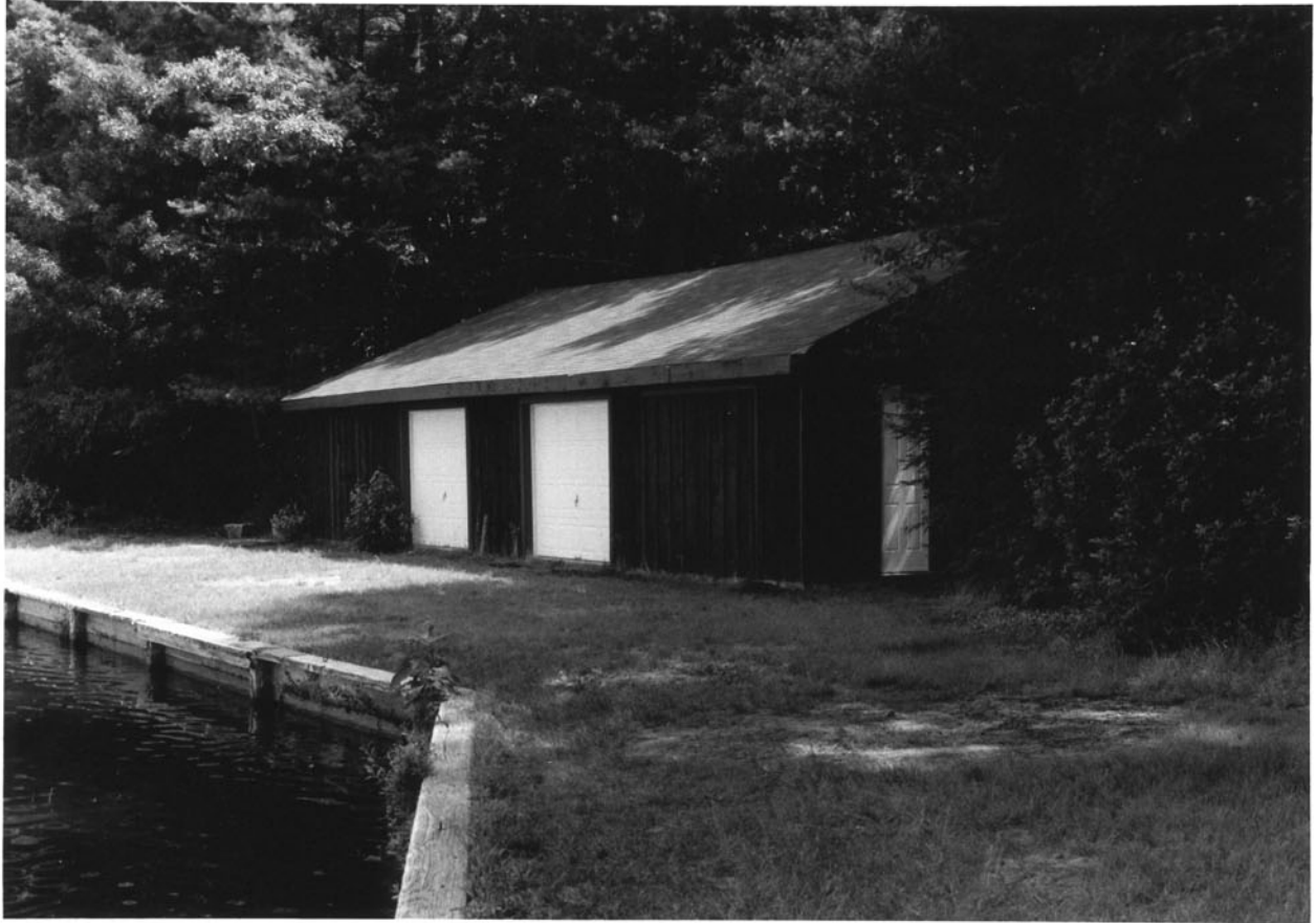
15. Boat House. Showing south and west façades, looking north. (Photographer: Timothy Orwig, July 2002)
