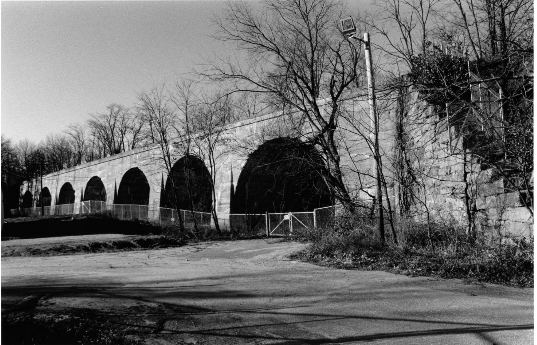
1. View looking northwest showing south face of Multiple-Arch Bridge with Multiple-Arch Bridge East Abutment at right (Photographer: Matthew A. Kierstead, 18 November 1999)
