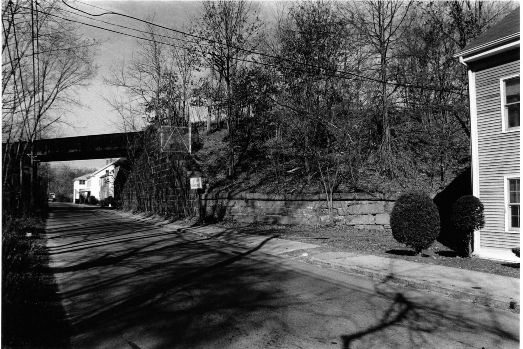
5. View looking northwest showing, from left to right, Canal Street Bridge Abutment, and West Embankment and granite retaining wall, with Waterford mill housing at right (Photographer: Matthew A. Kierstead, 18 November 1999)
