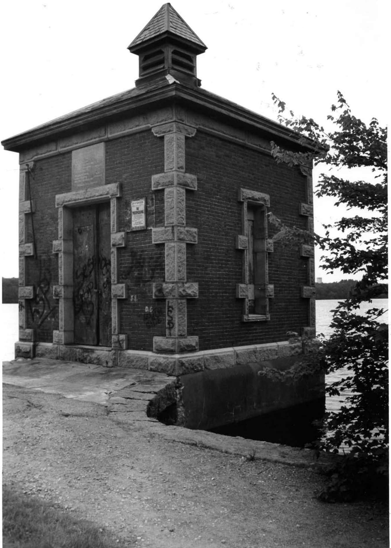
19. Reservoir Gate House (Photographer: Child Associates, June 1998)
