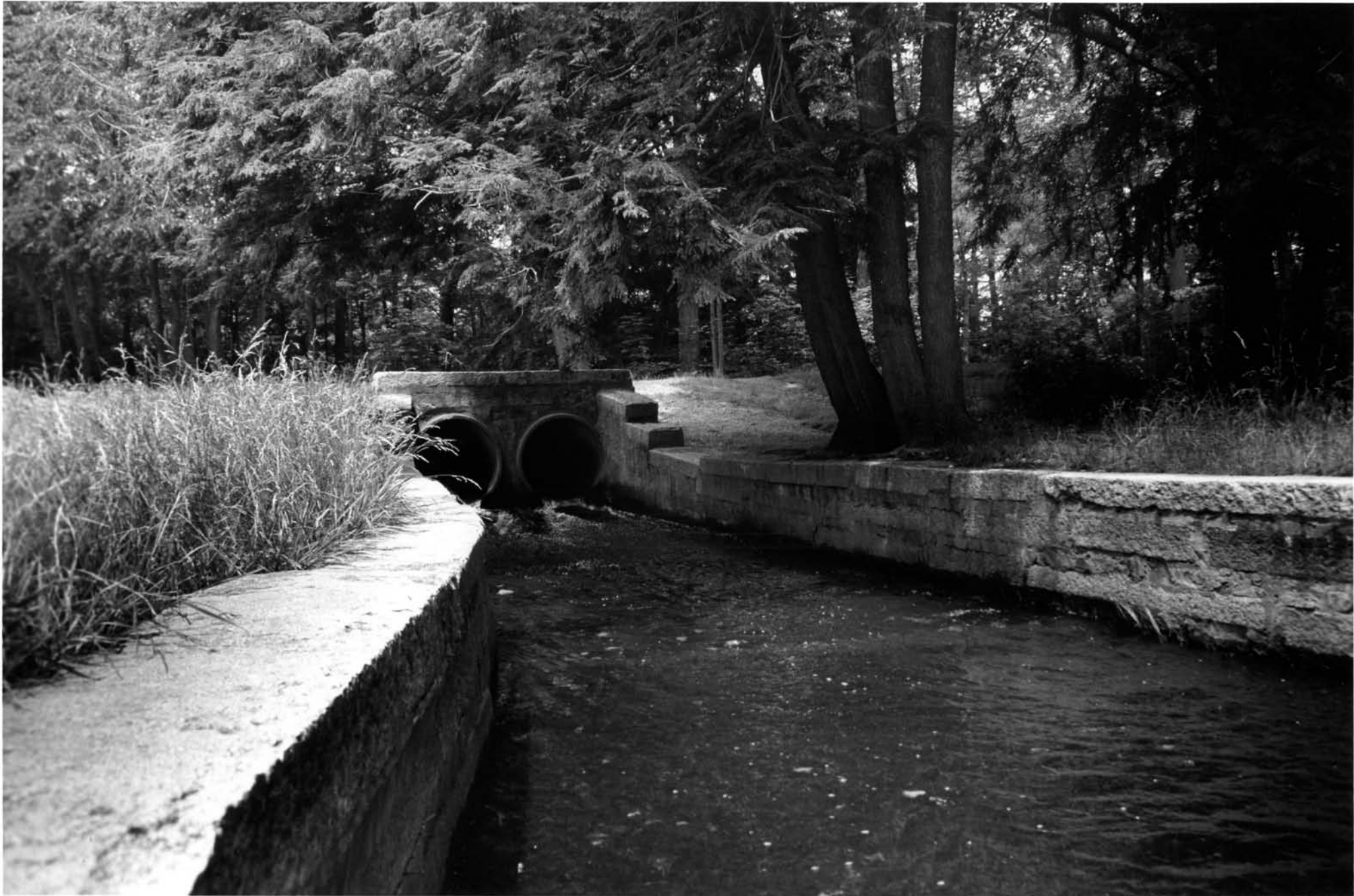
2. Sluiceway and parkway bridge, facing W (Photographer: Child Associates, June 1998)
