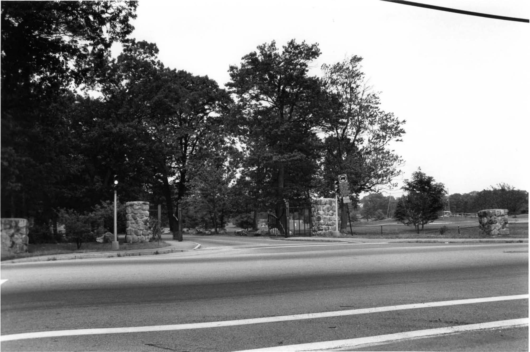
7. Oak Street, Brockton, entrance, facing E (Photographer: Child Associates, June 1998)
