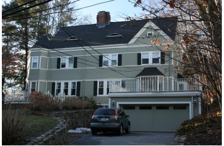
Façade (east) and north elevations.
